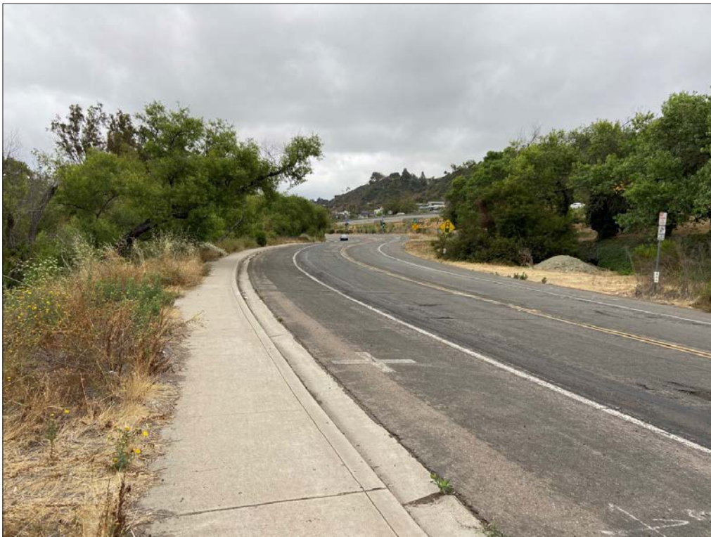
Looking east at the southern riparian forest habitat and non-native vegetation adjacent to developed land along Camino Del Rio North for the Regional Brine Line Extension. Open trench construction is proposed for this section of alignment.
