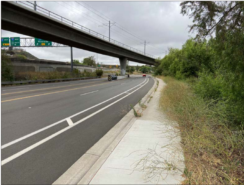
Looking west at the southern riparian forest habitat and non-native vegetation adjacent to developed land along Camino Del Rio North for the Regional Brine Line Extension. Open trench construction is proposed for this section of alignment.
