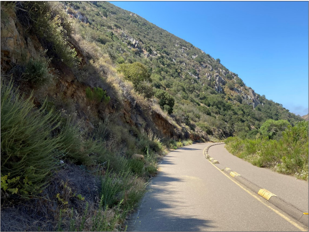
Looking south at the developed trail adjacent to Diegan coastal sage scrub and southern riparian forest habitats along the Father Junipero Serra Trail within Mission Trails Regional Park. Sliplining construction is proposed for this section of alignment.
