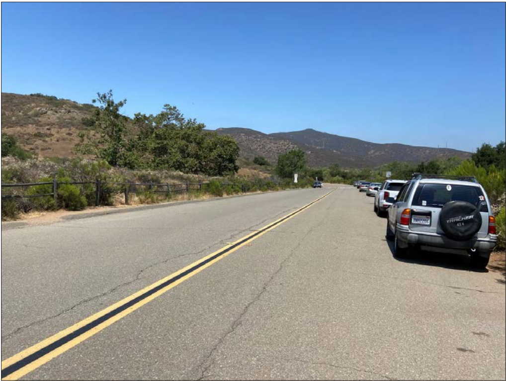
Looking south at the developed trail adjacent to Diegan coastal sage scrub habitat at the north end of the Father Junipero Serra Trail within Mission Trails Regional Park. Sliplining construction is proposed for this section of alignment.
