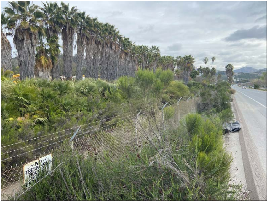
Looking northeast at the non-native vegetation adjacent to developed land along Mission Gorge Road. Sliplining construction is proposed for this section of alignment.
