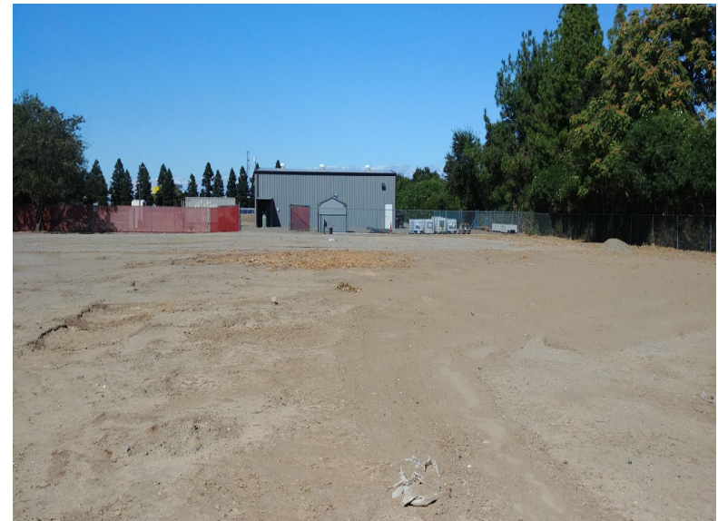
Eastern Portion of WTP Looking North, September 19, 2019
