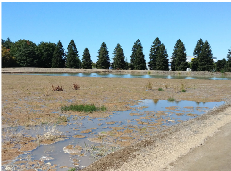
Backwater Basin Looking Northwest, September 19, 2019
