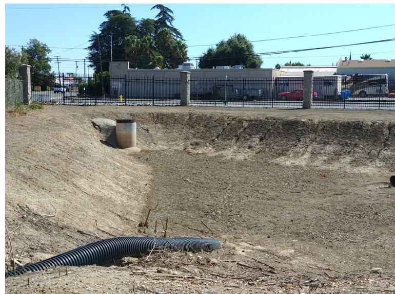
Detention Basin in Southeastern Portion of WTP, September 19, 2019
