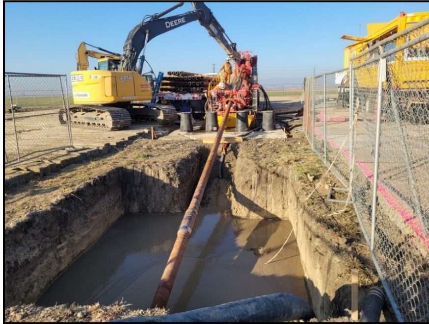
Figure 2-9. Photograph of an Example Drilling Rig and Bore Pit
