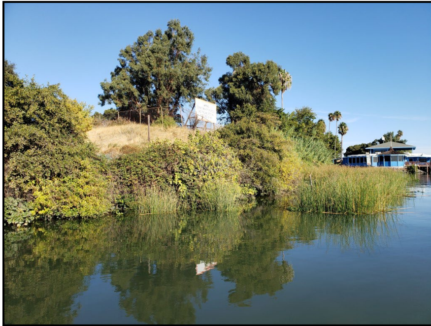
Figure 2-14. Photograph of the Segment 2 Pipeline Crossing the Sacramento River Taken of the West Bank
