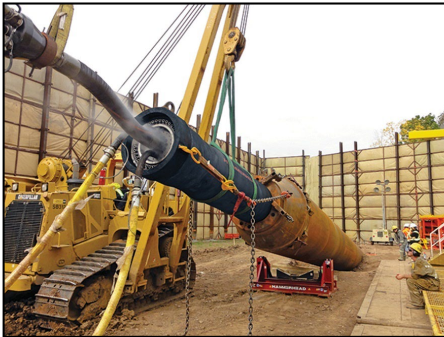
Figure 2-8. Photograph of Casing Installation with a Pneumatic Hammer
