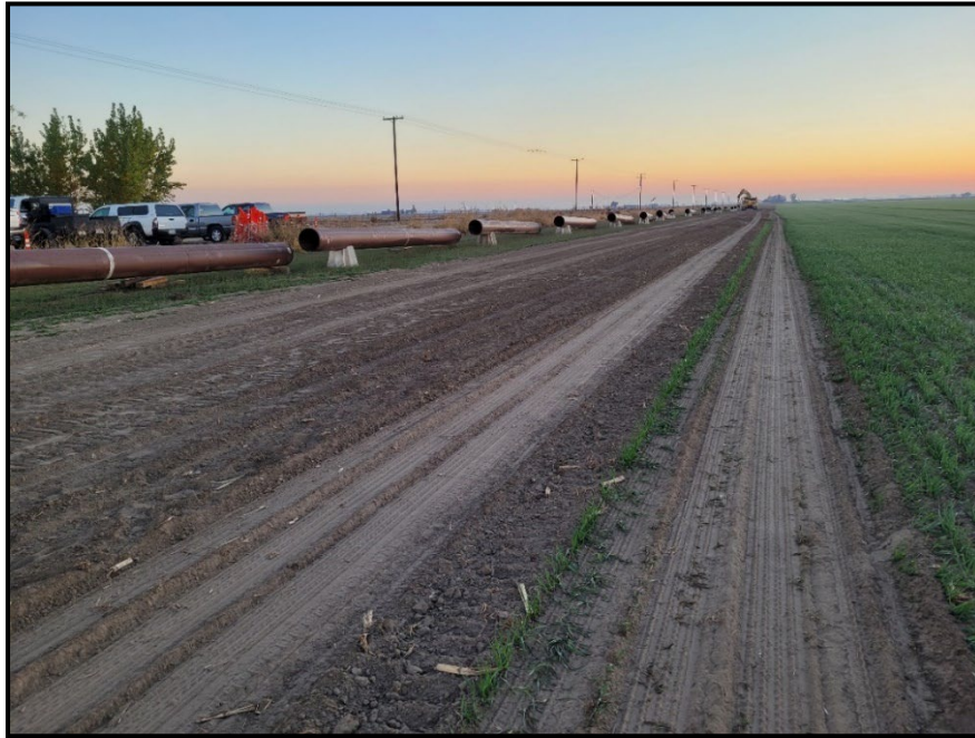
Figure 2-5. Photograph of Example Pipe Staging Area
