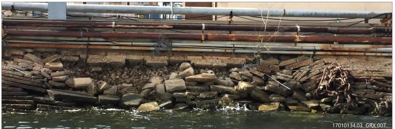
Source: Photograph by Anchor QEA, LLC in 2020.
