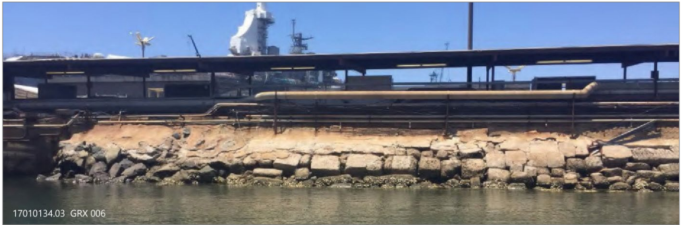
Source: Photograph by Anchor QEA, LLC in 2020.
