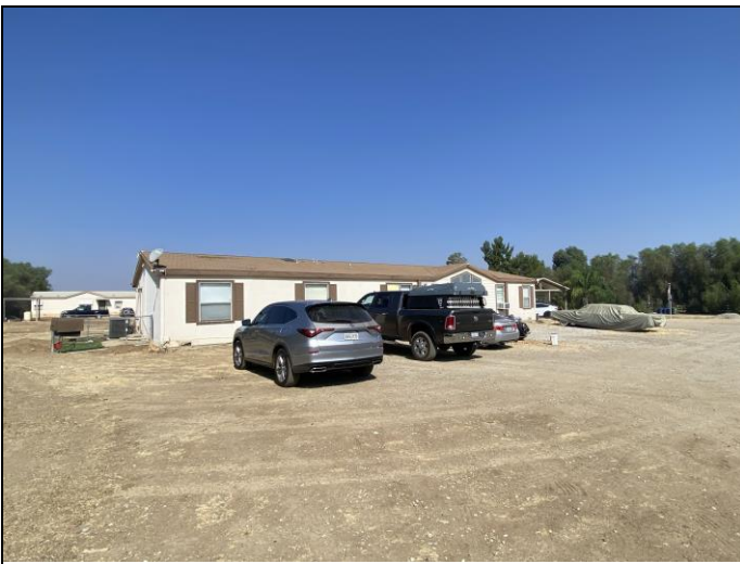
3. View of a typical onsite structure
