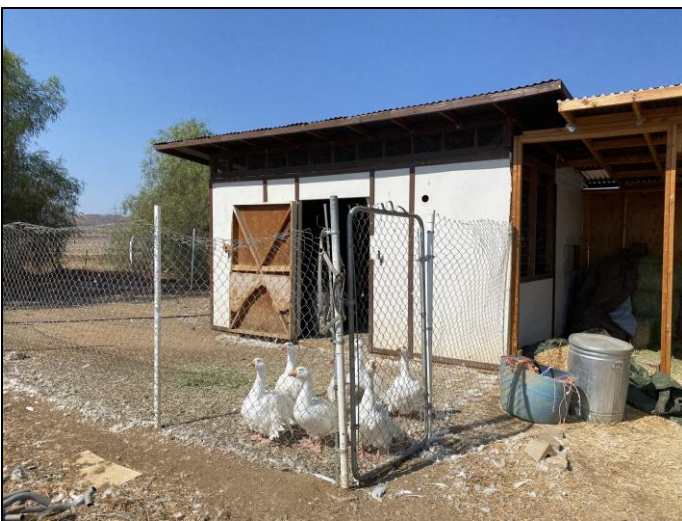
5. View of a typical onsite shed structure
