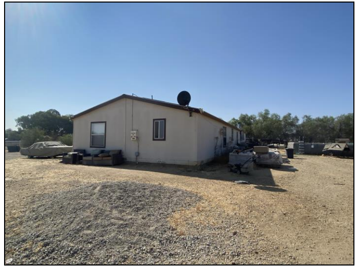
2. View of a typical onsite structure
