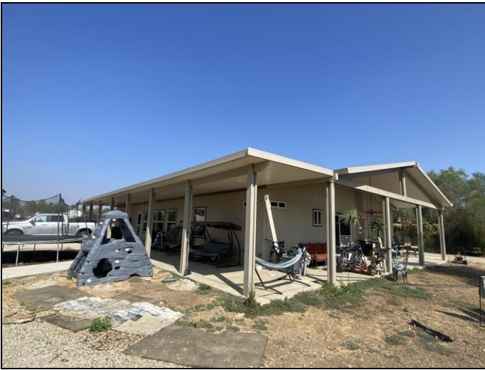
1. View of a typical onsite structure
