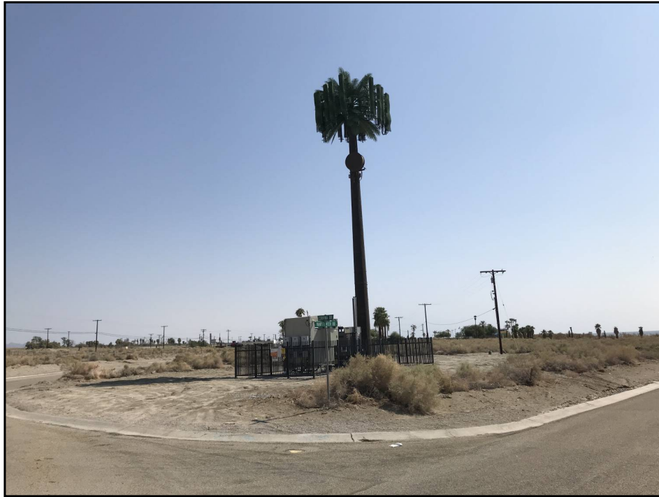
View of antenna equipment west of the Property, at Vander Veer Road and Corvina Drive.
