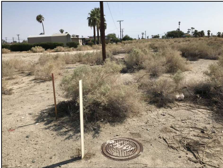
Water utility access cover at west Property line.
