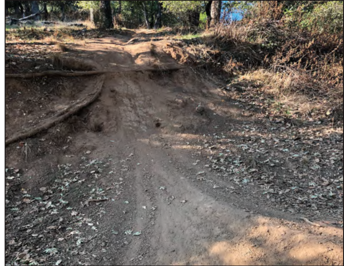
Photo 6: Jump showing exposed tree roots and erosion.
