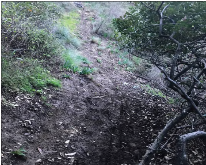
Photo 7: Narrow section causing vegetation loss.
