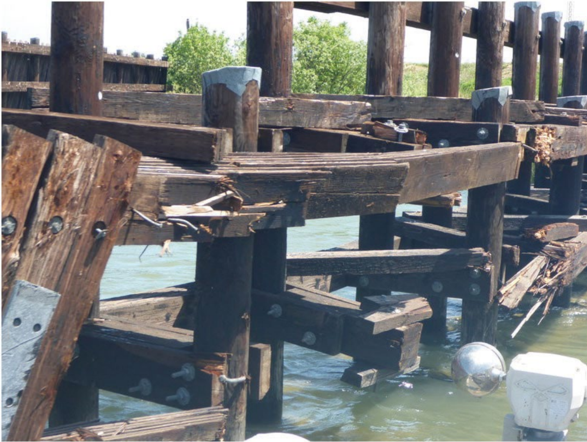
Figure 1-3. Existing Fender System on Ryer Island
