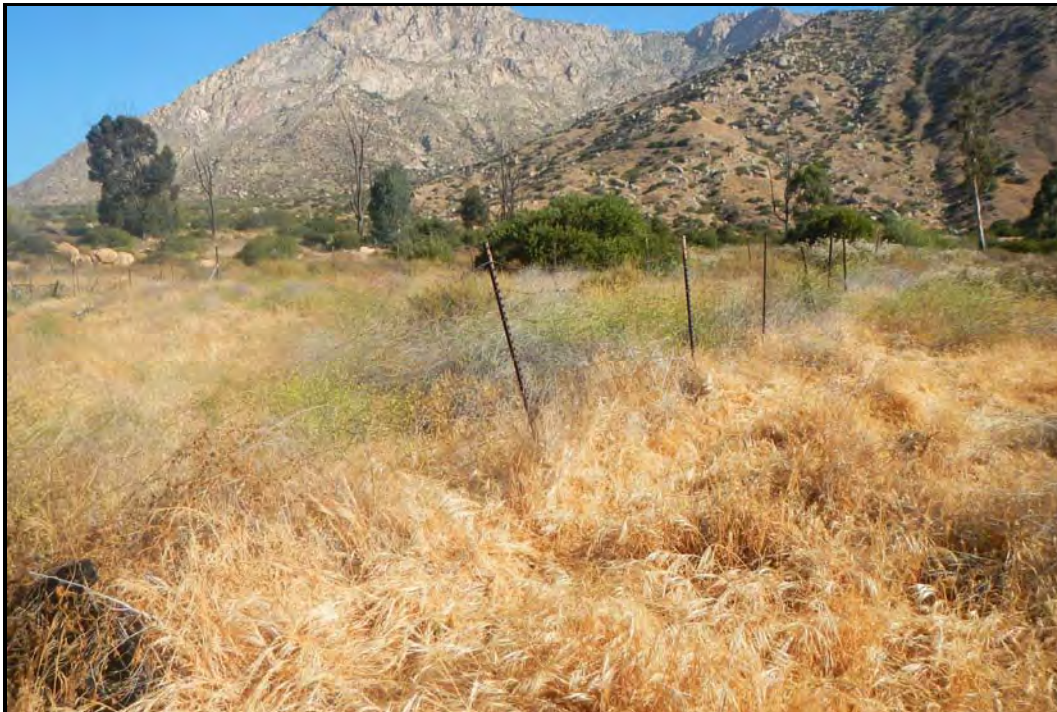
PHOTOGRAPH 18 El Capitan Spillway AA, View of Degraded Fence Included in Buffer June 6, 2018
