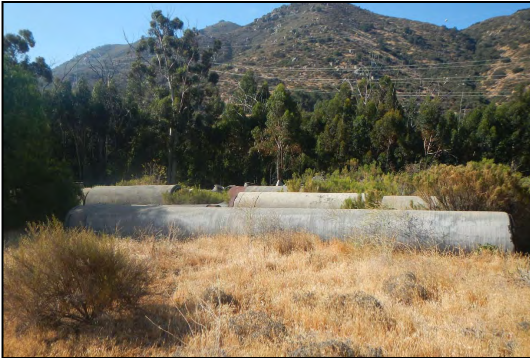
PHOTOGRAPH 17 El Capitan Spillway AA, View of Staging Yard Included in Buffer June 6, 2018
