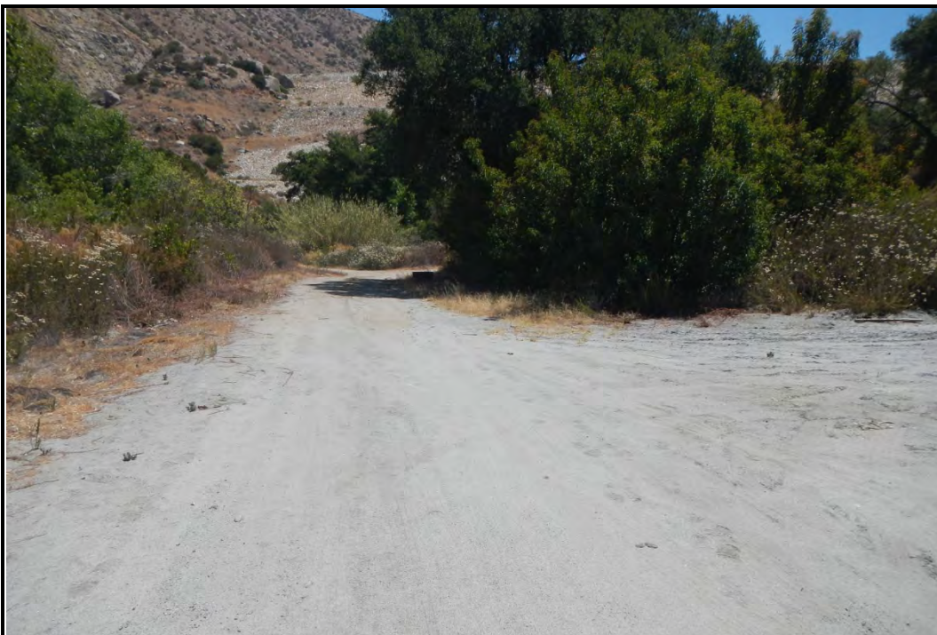
PHOTOGRAPH 8 El Capitan Dam AA, View of At-grade Unpaved Road Included in Buffer June 6, 2018
