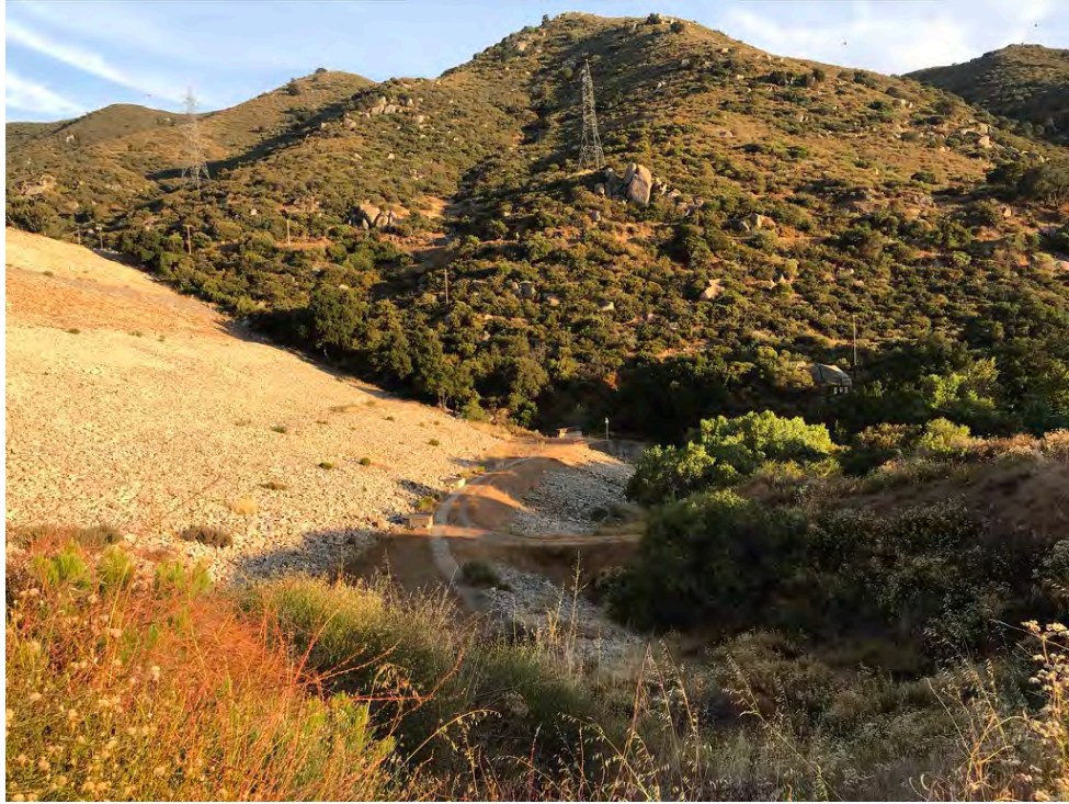
Photo 7. El Capitan Dam – View of the base of El Capitan Dam and the survey area downstream, facing east. June 23, 2020.
