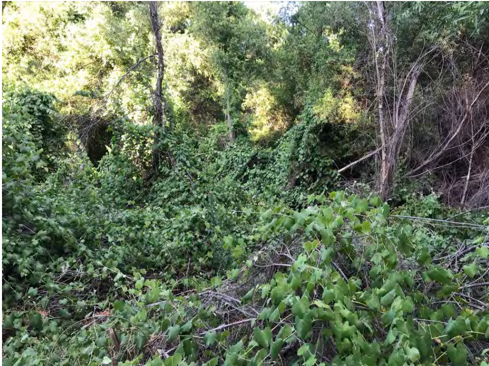
Photo 12. El Capitan Dam – View of vegetated streambed downstream of El Capitan Dam. June 23, 2020.
