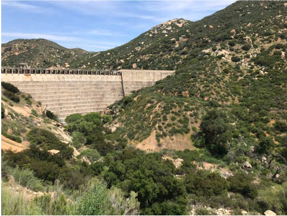
Photo 1. Barrett Dam – View from Barrett Lake Road of Barrett Dam and Cottonwood Creek within the survey area, facing north. April 29, 2020.
