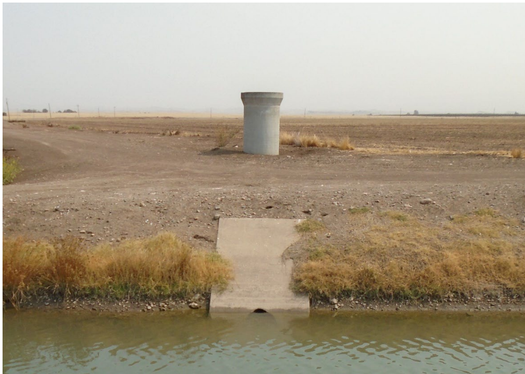
Description of Photo: F-12, cement culvert with cement cistern on the east side of the Le Grand Canal. View east. September 21, 2021 (Cistern: UTM 10 N 741109 mE/ 4131492 mN, . UTM 10 N 741098 mE/ 4131493 mN).
