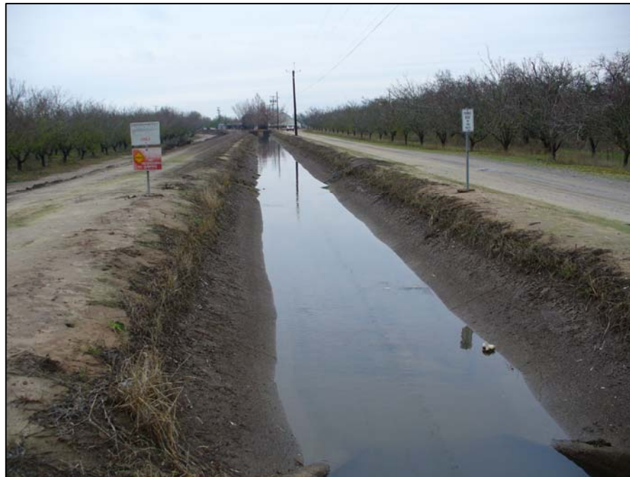
Photograph 45. Buhach Lateral at point BH1, camera facing north. 12/12/06.
