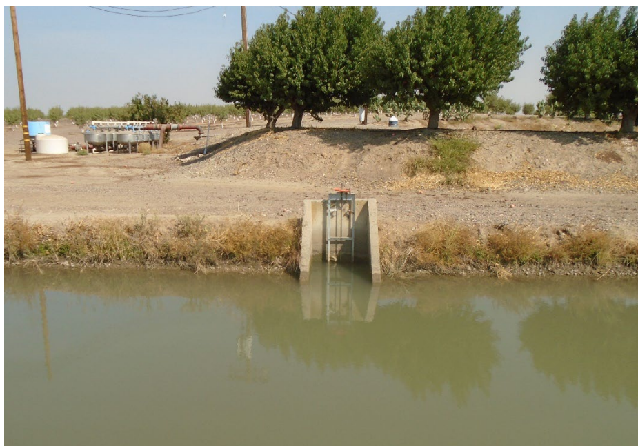
Description of Photo: F-33 overview. View north. Cement and metal sluice. Possibly leads to a holding pond approximately 63 feet to the northeast. September 23, 2021 (UTM 10N 742768 mE/ 4125527 mN).
