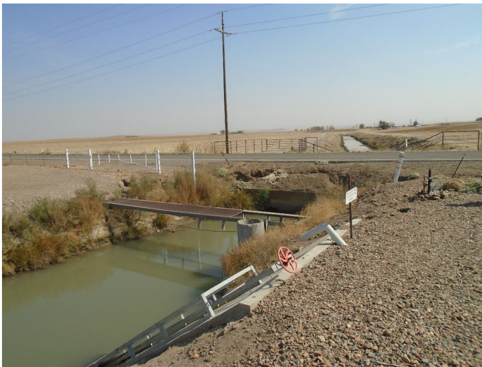
Description of Photo: Overview of F-35 and F-36. View east. September 23, 2021.
