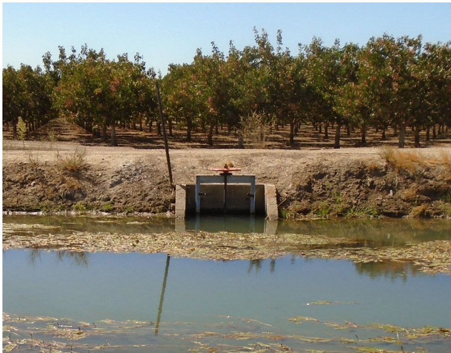
Description of Photo: F-04, concrete-lined sluice leading to south-flowing canal channel. View south. September 20, 2021 (UTM 10N 739293 mE, 4133103 mN).
