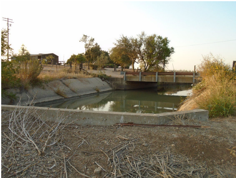
Description of Photo: North elevation of F-13. View south. September 22, 2021.
