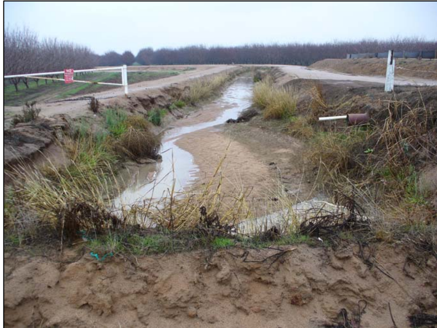
Photograph 39. Henderson Lateral at point HN1, camera facing north. 12/12/06.
