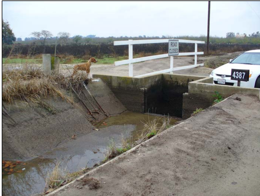
Photograph 33. Main Ashe Lateral showing slide gates at point MA3, camera facing southeast. 12/12/06.
