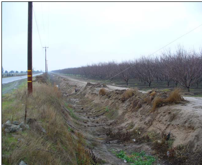
Photograph 47. Drainage Ditch at point DR1, camera facing west. 12/12/06
