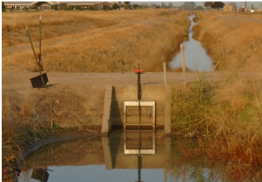
Description of Photo: F-08, cement-line sluice, leading to a historic west-flowing canal channel. A tag on the sluice reads "089596 R 24L 07 00 U." (UTM 10S 741152mE/ 4131135mN).
