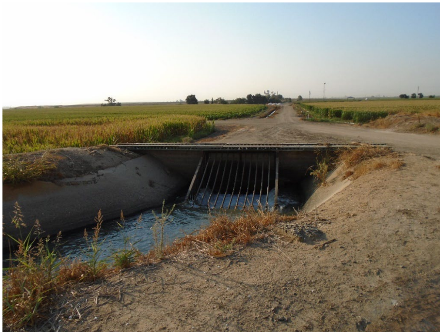
Description of Photo: F-17, cement inlet that leads into the underground flume. The inlet spans the Le Grand Canal and is approximately 30 feet wide. A metal barricade rests over the opening. The section of canal between features F-17 and F-18 is lined with cement. View south. September 22, 2021 (UTM 10N 741236 mE/ 4129296 mN).
