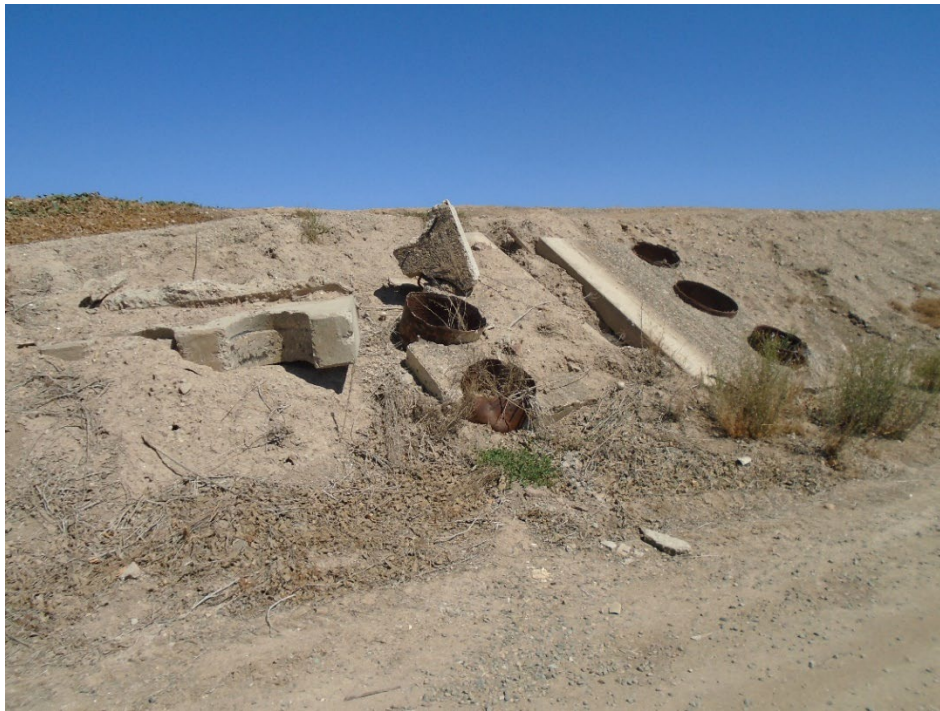
Description of Photo: Concrete and ferrous pipe debris on the western berm of the Le Grand Canal, 20 feet south of feature F-05. View north. September 20, 2021.
