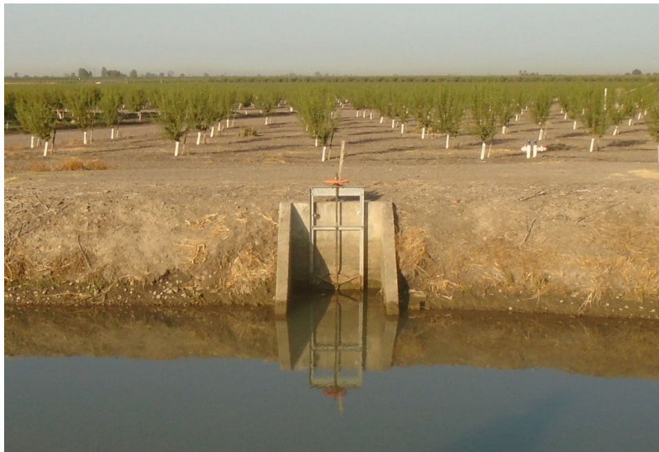
Description of Photo: F-24 overview. View west. Cement and metal sluice. A tag on the cement reads "101544 R 241 0500U." September 23, 2021 (UTM 10N 741334 mE/ 4128000 mN).
