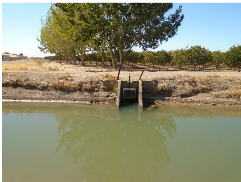
Description of Photo: Overview of F-01, cement-lined sluice leading to south-flowing channel. View south. September 20, 2021 (10N 739510 mE/ 4132707).
