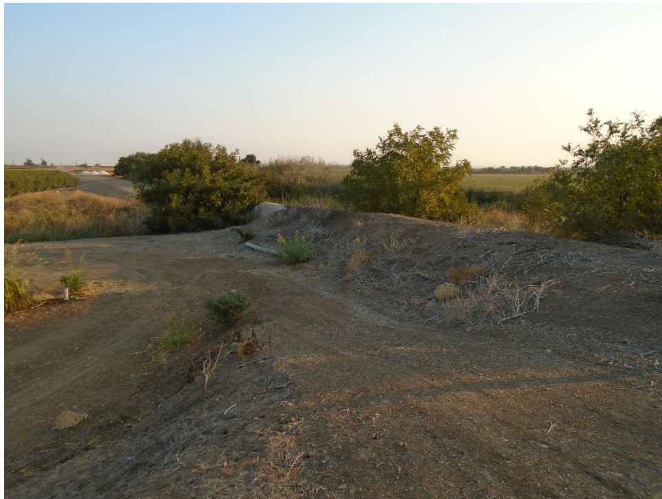
Description of Photo: Southern segment of F-14 at ground level but covered with dirt. View northeast. September 22, 2021.
