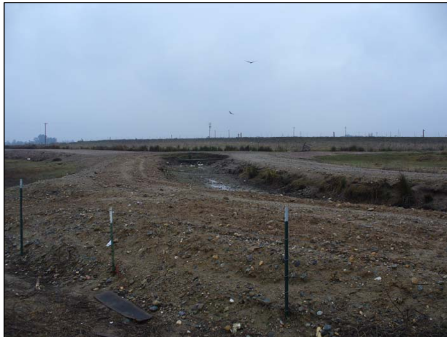
Photograph 40. Henderson Lateral at point HN1, camera facing southeast. 12/12/06.
