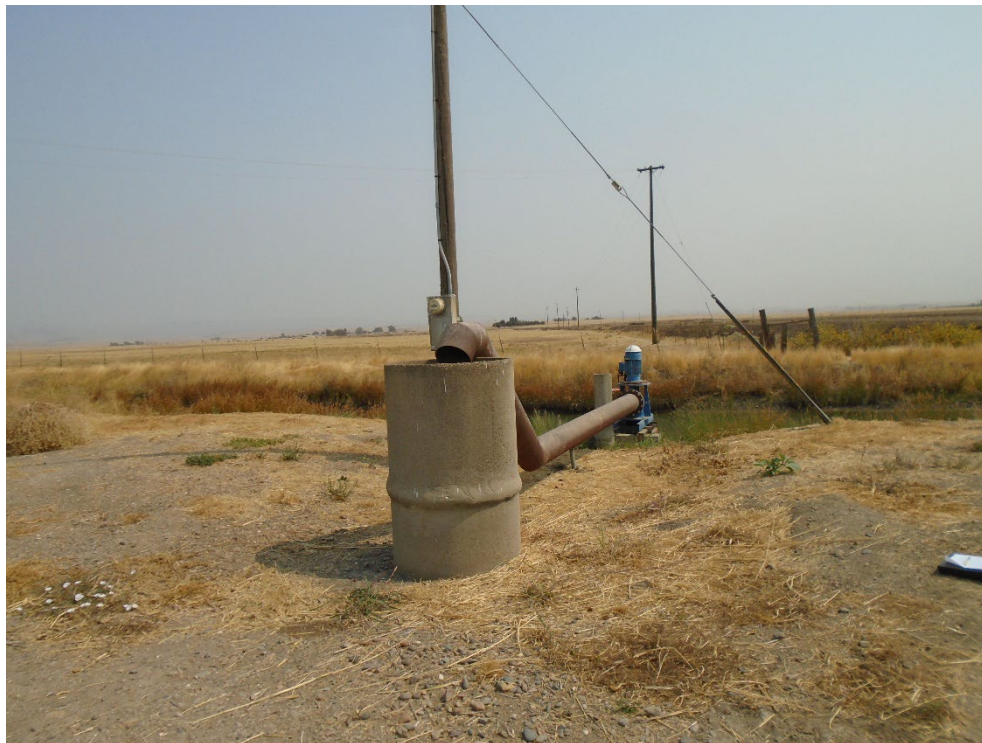
Description of Photo: Overview of F-09 pipe and cement cistern. View east. September 21, 2021.
