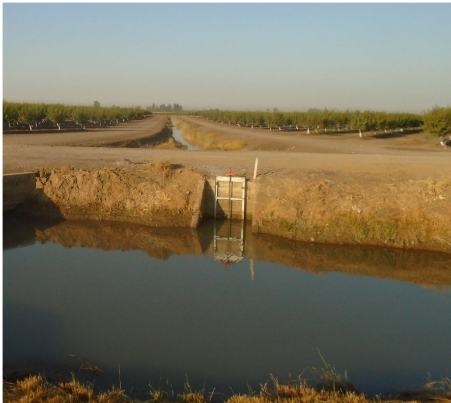
Description of Photo: F-26 overview. View west. Cement and metal sluice leading to a west-flowing canal channel. September 23, 2021 (UTM 10N 741519 mE/ 4127484 mN).
