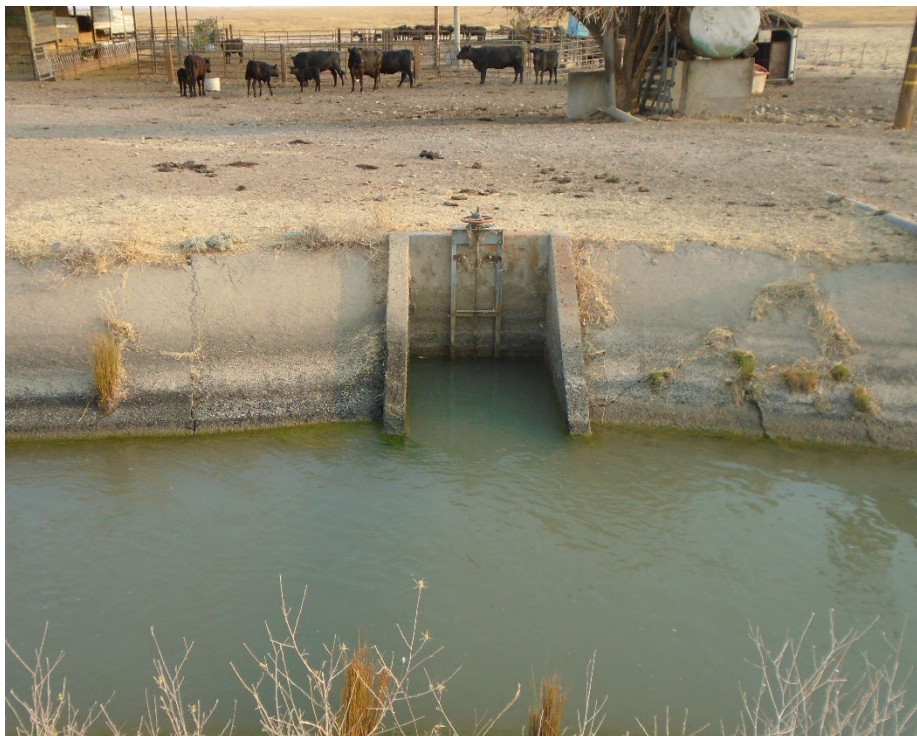
Description of Photo: F-40 overview with adjacent cattle ranch in the background. View north. Cement and metal sluice on the north side of the Le Grand Canal. A tag on the sluice reads "006620 R 12 7 0600U." September 24, 2021 (UTM 10N 744252 mE/ 4126037 mN).
