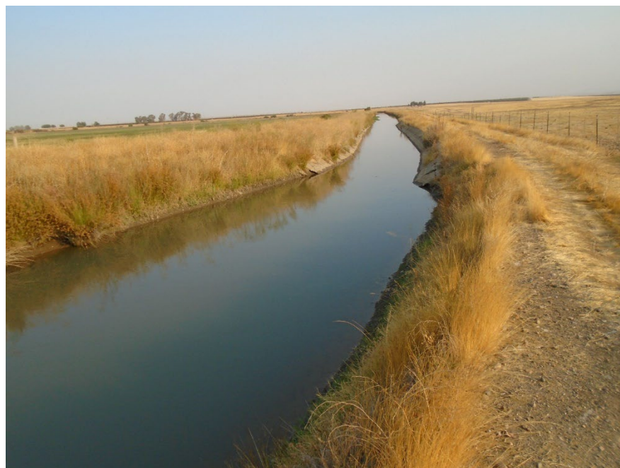
Description of Photo: Transition from earthen to cement-lined. Small segment of cement-lined canal that runs roughly southeast-northwest. This segment is approximately 285 feet long and lies between two widened earthen segments View north. September 21, 2021 (UTM 10N 741090 mE/ 4131618 mN)
