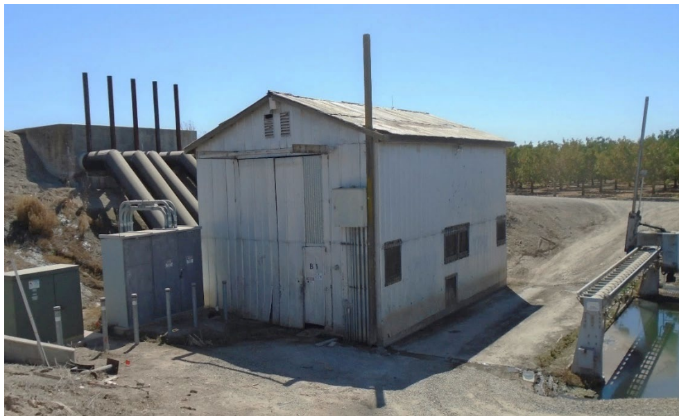
Description of Photo: North and east elevation of pump house (F-06). View southeast.
