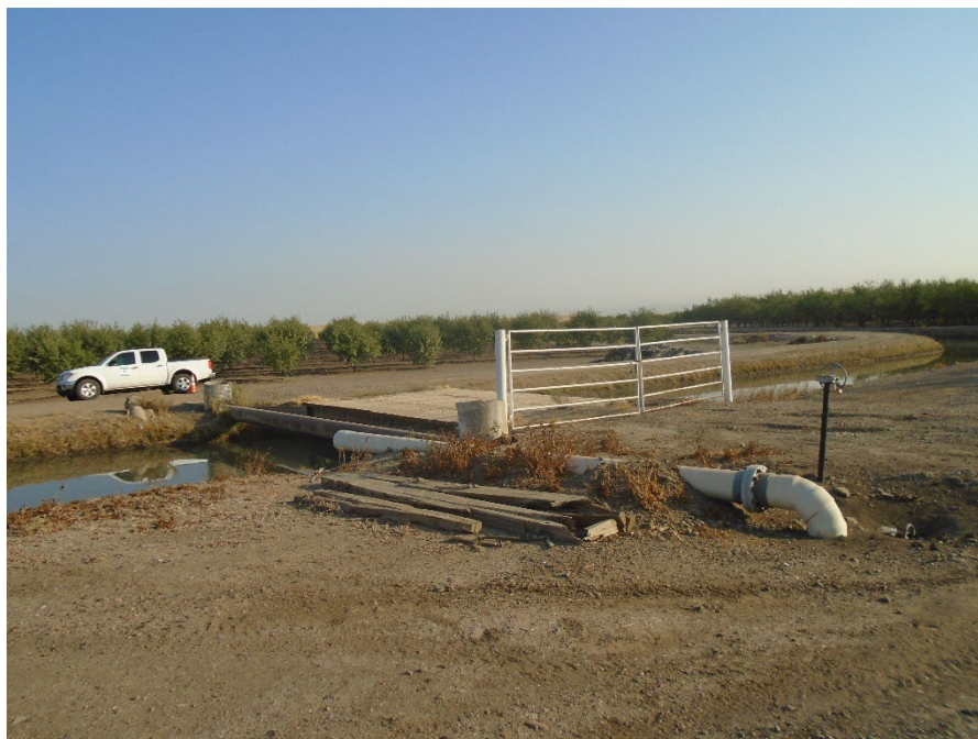
Description of Photo: F-28, overview. View northwest. Wooden bridge with cement footings. A metal gate prevents automobile access on the southeast side. A 22-foot length of PVC pipe leads into the Le Grand Canal on the southeastern side. A tag on the northeastern corner of the cement footing reads "110035 Y 2 16." September 23, 2021 (10N 742576 mE/ 4126524 mN).
