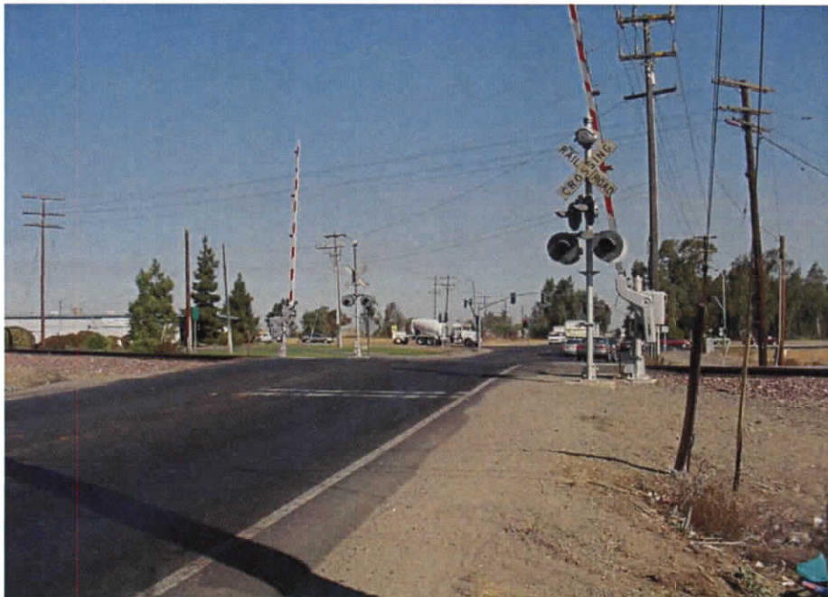
Intersection of Santa Fe RR and S.R. 59, looking north
