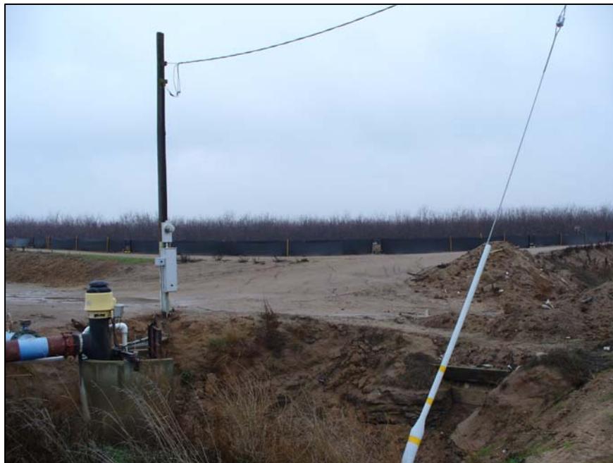
Photograph 41. Pump, lower left, timber supports for access road, lower right, fenced basin in background, camera facing northeast, near Henderson Lateral, point HN1. 12/12/06.
