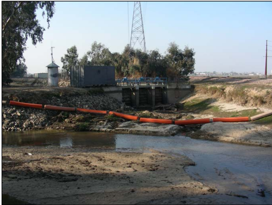
Photograph 49. Livingston Canal headgate (point LC1), Canal Creek in foreground camera facing west. 1/22/07.
