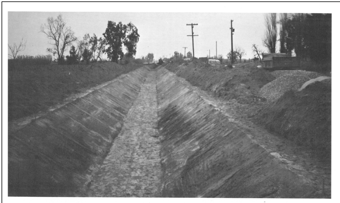
Figure 6. Arena Canal being shaped for concrete lining in 1950. (McSwain 174)
