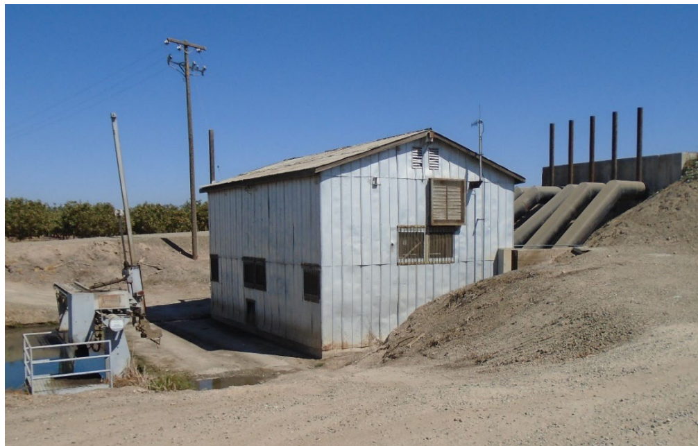
Description of Photo: South and west elevations of F-06. View northeast. September 20, 2021.
