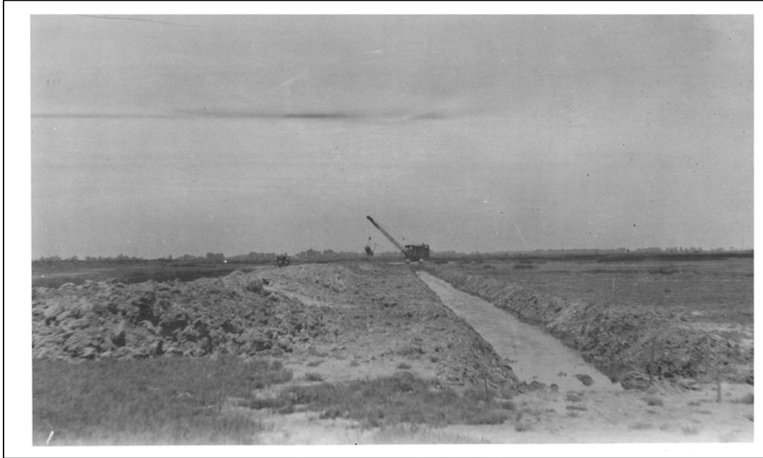
Figure 11. Dragline in 1929 digging a drainage ditch. (McSwain 95)
