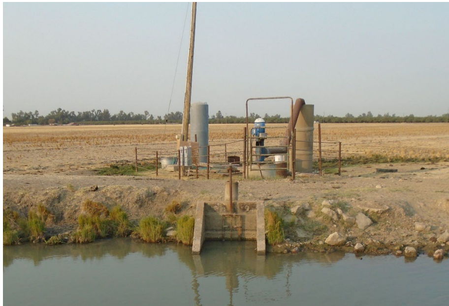
Description of Photo: Overview of F-42. View west. Metal and cement sluice in the west side of the Le Grand Canal. Approximately 20 feet west of the sluice are several cement cisterns, a pump, and a distribution pole September 24, 2021 (UTM 10N 744262 mE/ 4126016 mN).
