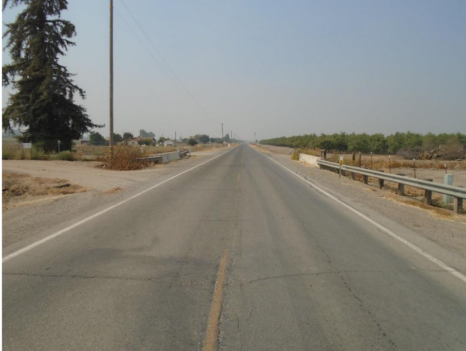
Overview of East Childs Road, facing west.
