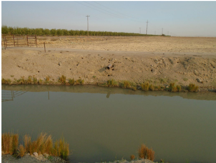
Description of Photo: Overview of F-45. View north. Ferrous pipe on the north side of the Le Grand Canal. The pipe no longer spans the canal. September 24, 2021 (UTM 10N 743714 mE, 4125968 mN).
