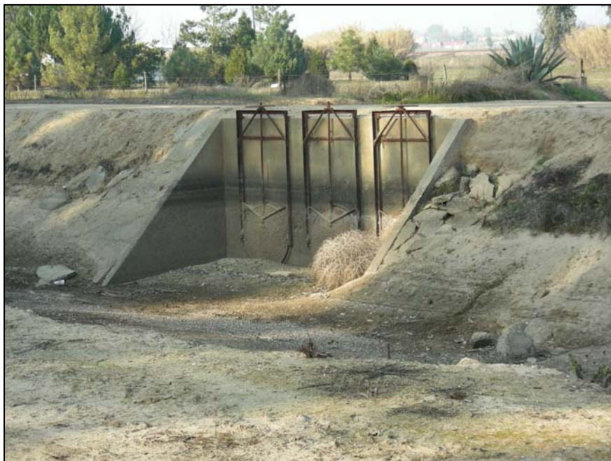
Photograph 50. Lateral gates off of Livingston Canal (point LC1), camera facing northwest. 1/22/07.
