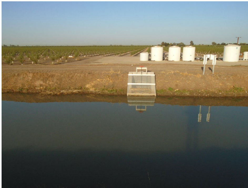
Description of Photo: F-22 overview. View west. September 23, 2021 (UTM10N 741283 mE/ 4128346 mN).
