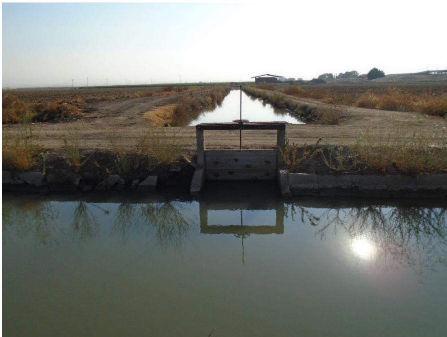
Description of Photo: Overview F-21. View east. Wooden sluice to allow water into a historic canal channel September 22, 2021 (UTM 10N 741323 mE/ 4130041 mN).
