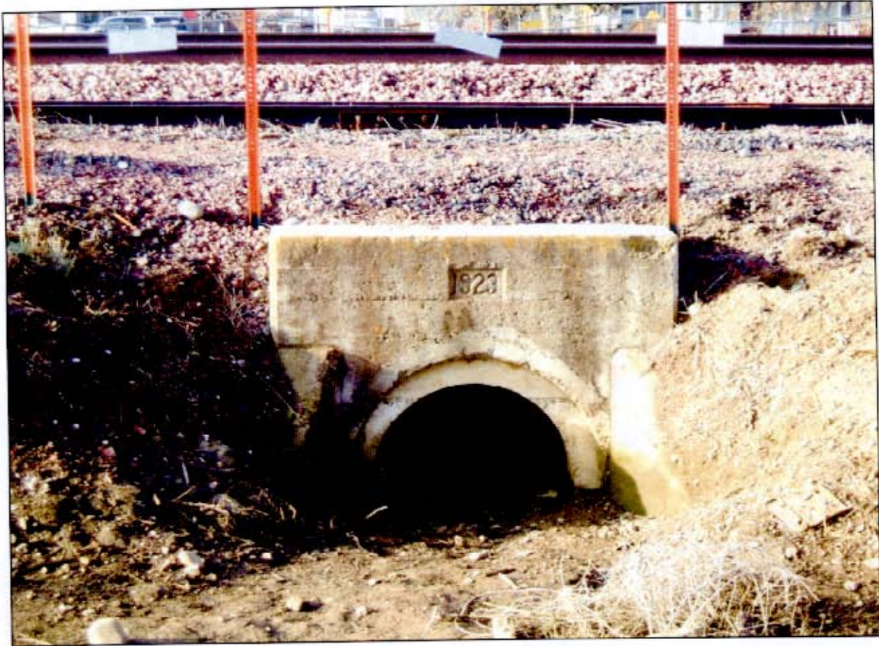
Concrete culvert with date stamp of 1923 (MP 1041.5)
