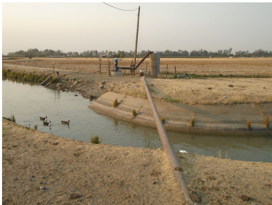
Description of Photo: Overview of F-41. View south. F-41 is a ferrous pipe that spans the width of the Le Grand Canal. The pipe leads to a cement cistern and pump on the south side of the canal. September 24, 2021 (UTM 10N 744255 mE/ 4126033 mN).
