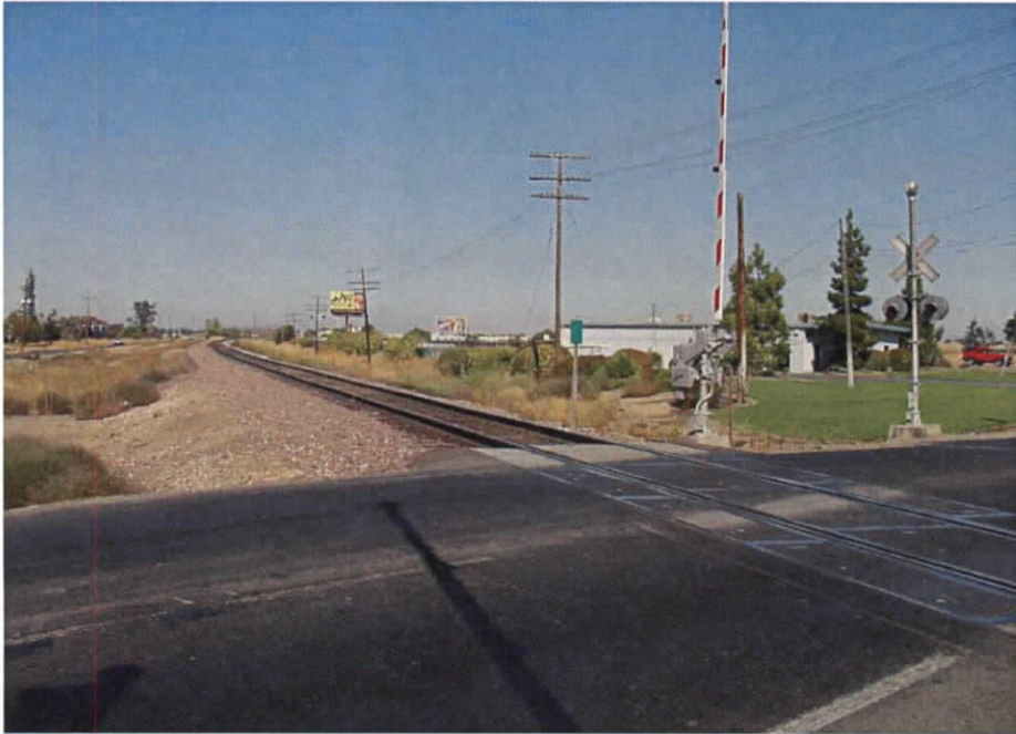
Looking west-northwest at intersection of S.R. 59
