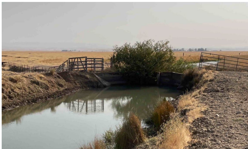
Description of Photo: West elevation of F-11. View northeast. September 21, 2021.
