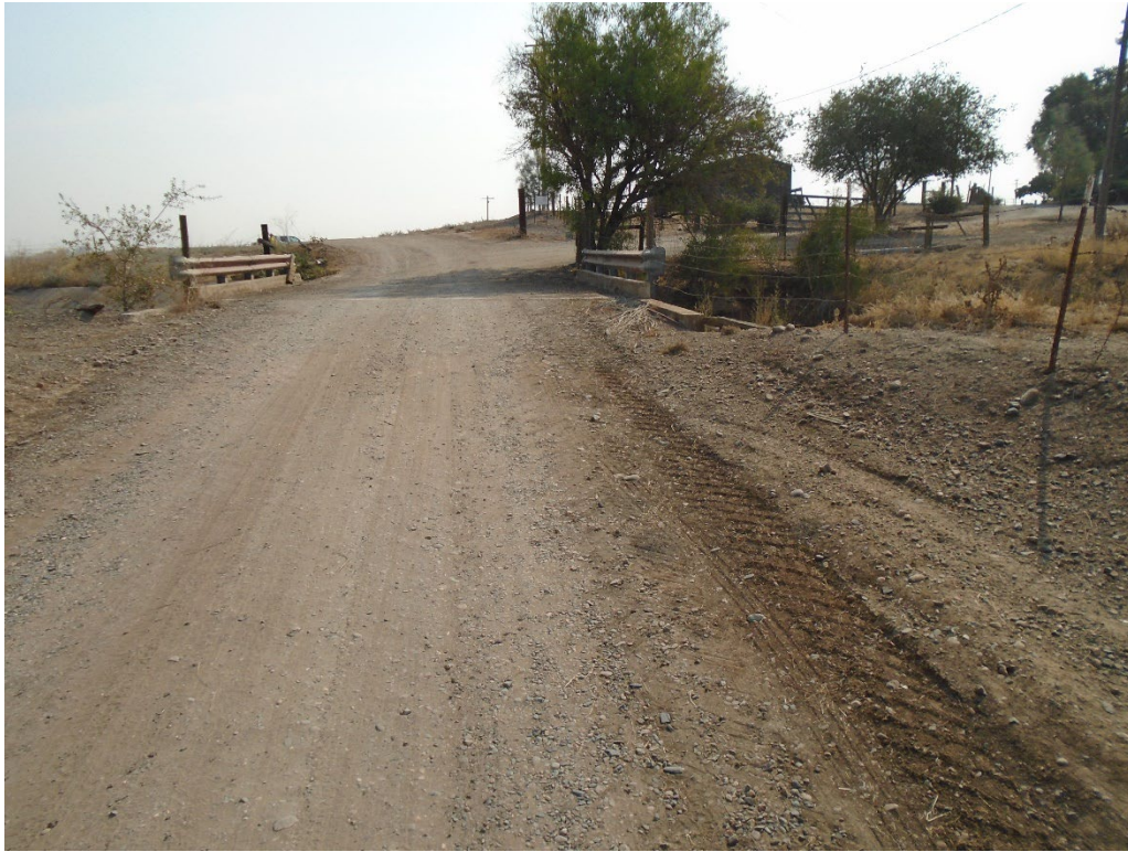
Overview of LG-06, facing northeast.
