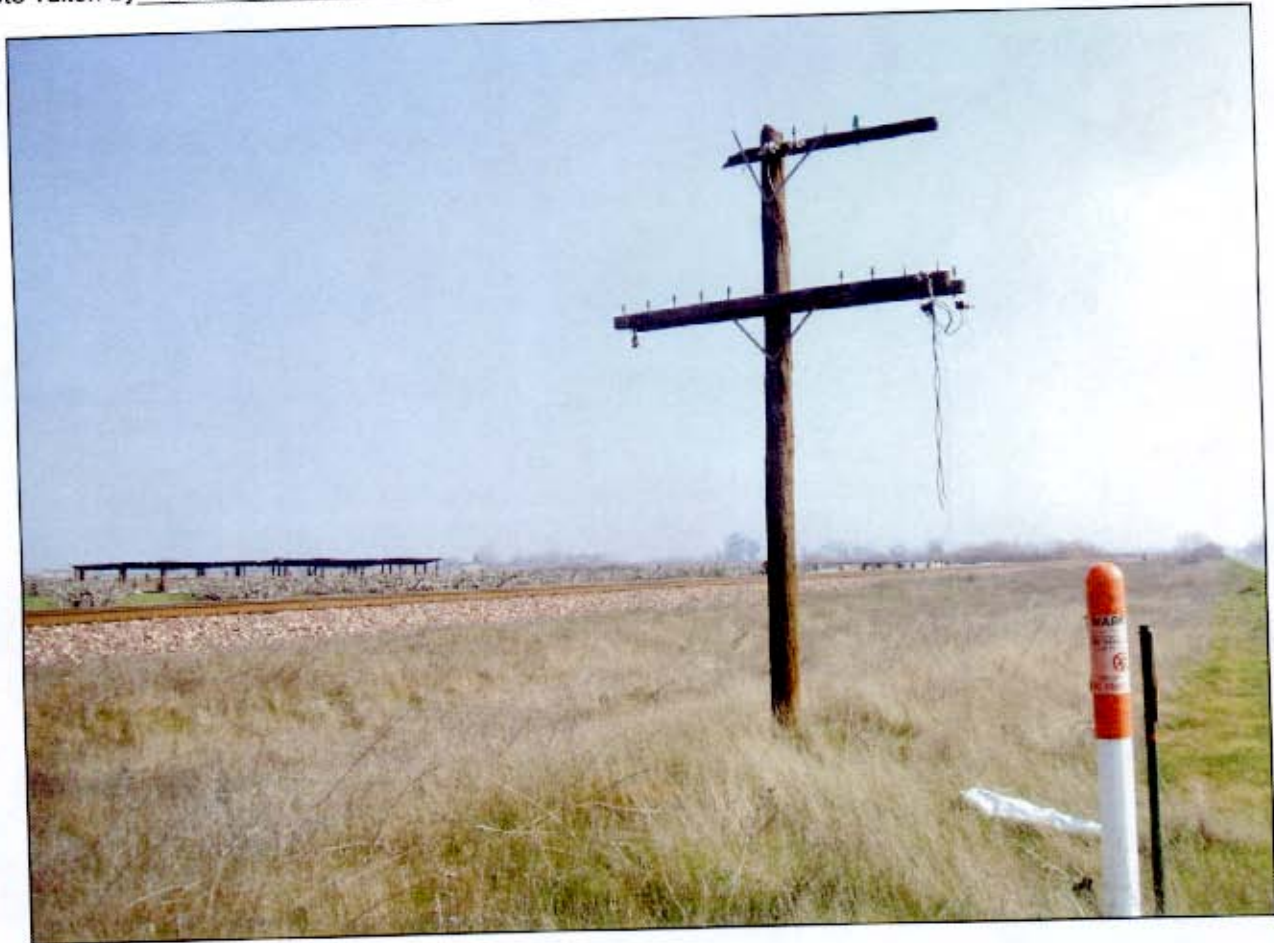
Abandoned isolated telegraph pole along the south side of the track (MP 1046.1)
