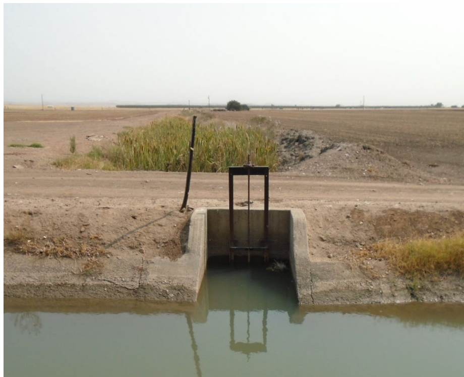
Description of Photo: F-07, cement-lined sluiceway, leading to a modern eastern-flowing canal channel. View east. September 21, 2021 (UTM 10N 741578 mE/ 4130875 mN).
