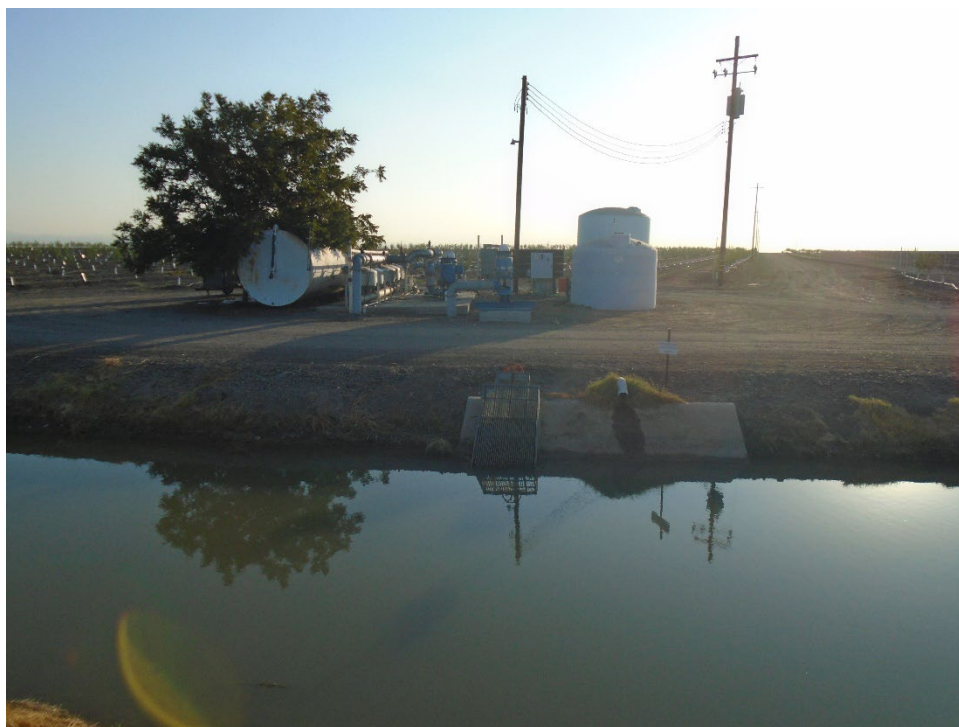
Description of Photo: F-25 overview. View east. Cement and metal sluice and associated machinery September 23, 2021 (Sluice: UTM 10N 741480 mE/ 4127647 and Machinery: UTM 10N 741494 mE/ 4127656 mN).
