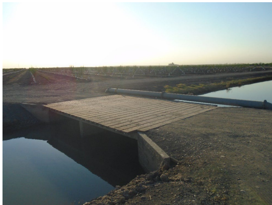
Description of Photo: F-27 overview. View east. Wooden bridge with cement footing and metal pipe on the south side. The bridge spans the Le Grand Canal and connects to access roads on either side. A tag on the northwest footing reads "103377 Y 2 16." September 23, 2021 (UTM 10N 741526 mE/ 4127478 mN).
