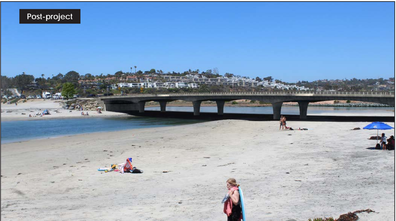
KEY VIEW 4 – From Sandy Lane Residences south of the San Dieguito River looking northeasterly toward the bridge.
