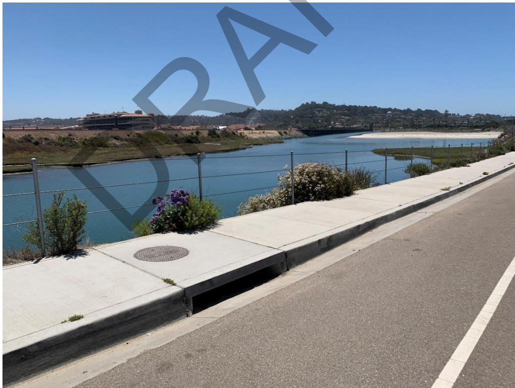
Photograph 14 - View of stormwater curb inlet along northeastern portion of the Project, looking southeast. The Del Mar Fairgrounds observed in the distance.
