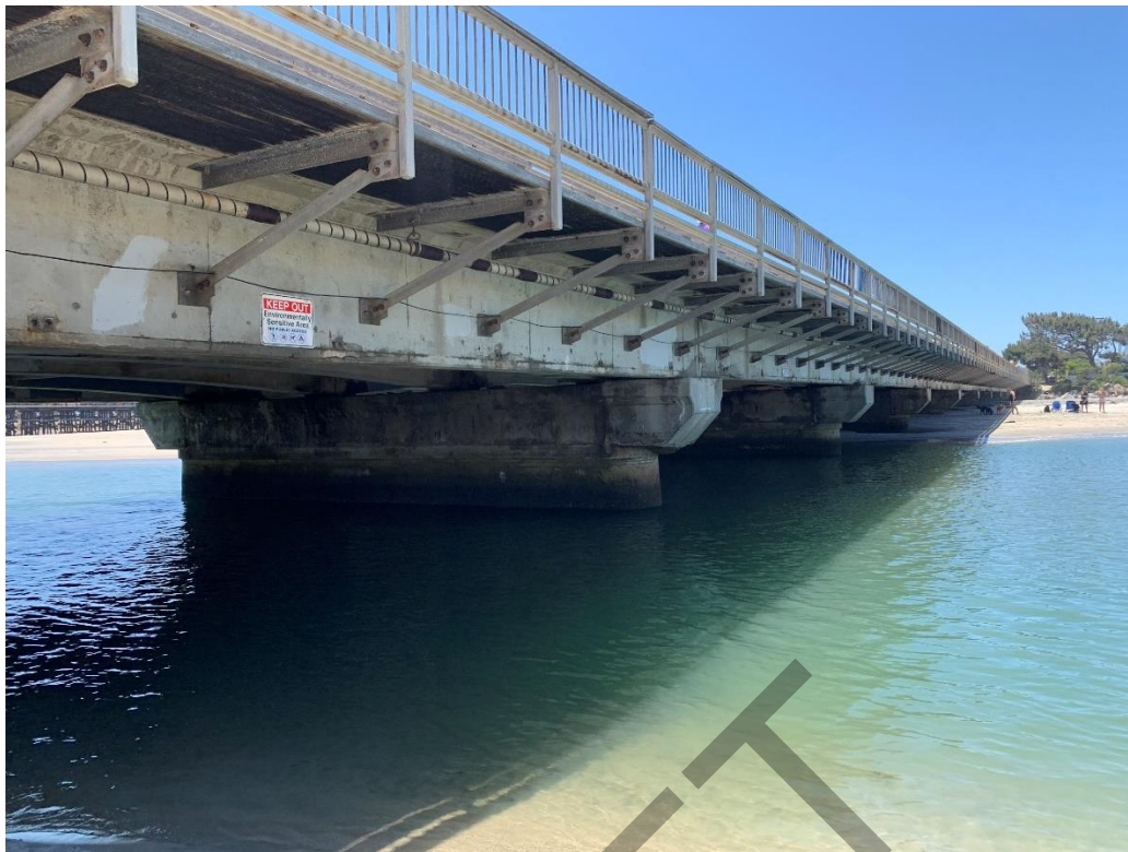
Photograph 5 - View of bridge structure from west side, looking southeast.
