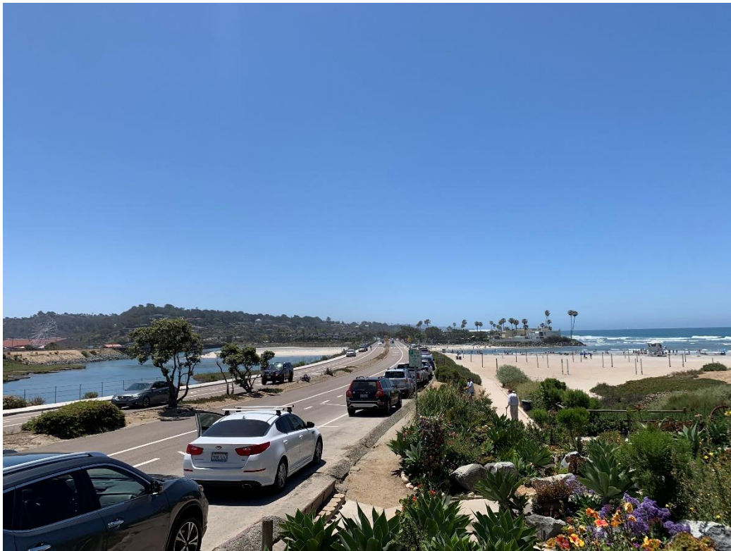
Photograph 15 - View of Camino Del Mar Bridge and Project area looking south.
