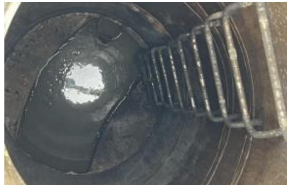
Manhole Before Install
