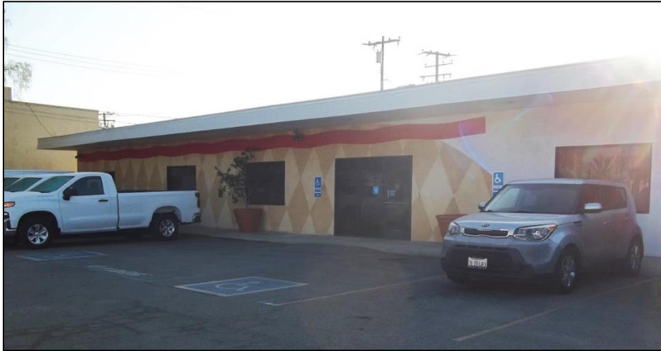
Figure 8. Northern half of west façade of 14202 Van Ness Avenue
