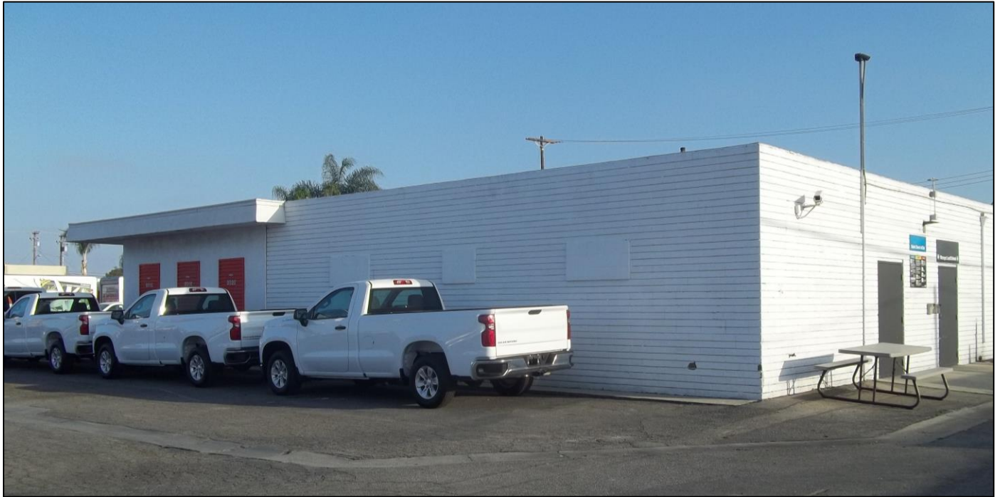
9. South elevation (left) and portion of east elevation (right) of 14202 Van Ness Avenue
