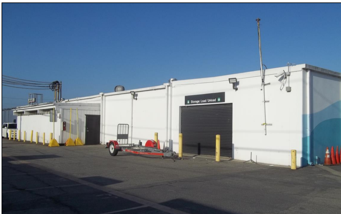
6. East elevation (left) and portion of north elevation (right) of 14206 Van Ness Avenue
