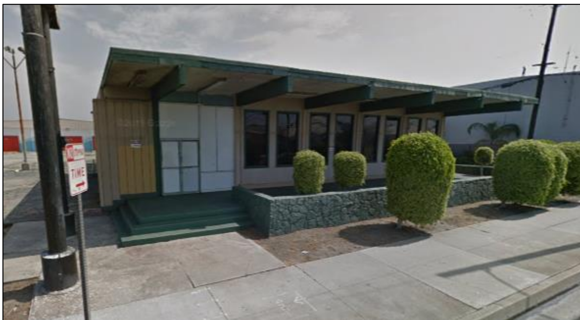
2145 Rosecrans Avenue, south façade, facing northeast (Google Street View 2016)
