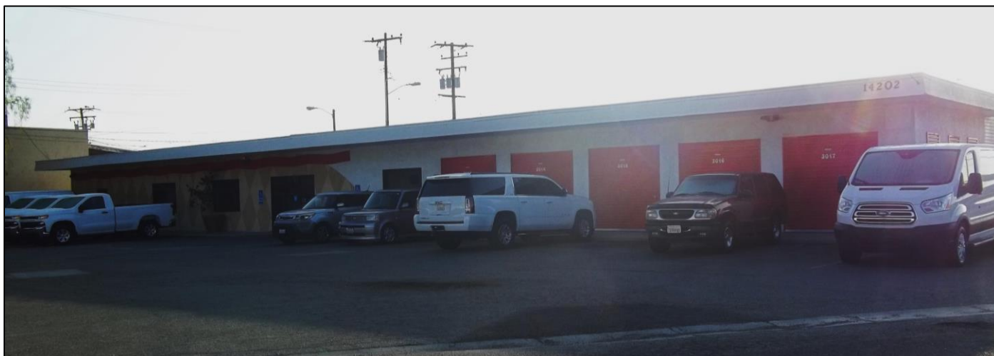
Administration building, July 2021
