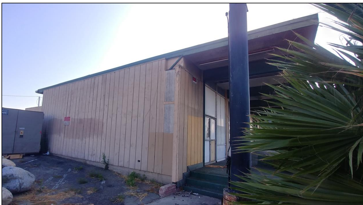
West elevation (left) and south façade (right); taken June 2021
