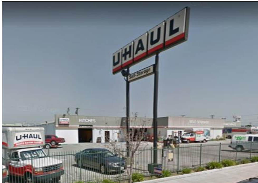
Main storage building, Google Street View; May 2012
