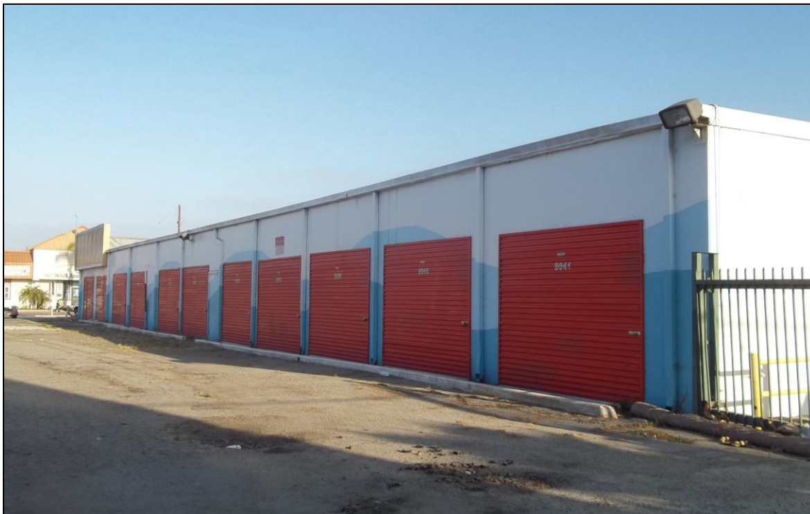
4. South elevation (left) and partial east elevation (right) of 14206 Van Ness Avenue
