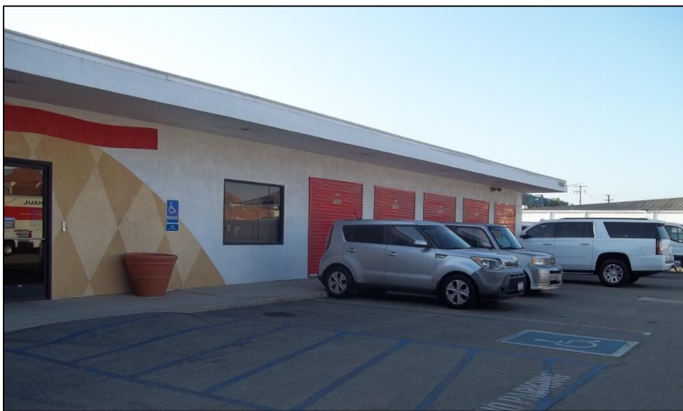
Figure 9. Southern half of west façade of 14202 Van Ness Avenue
