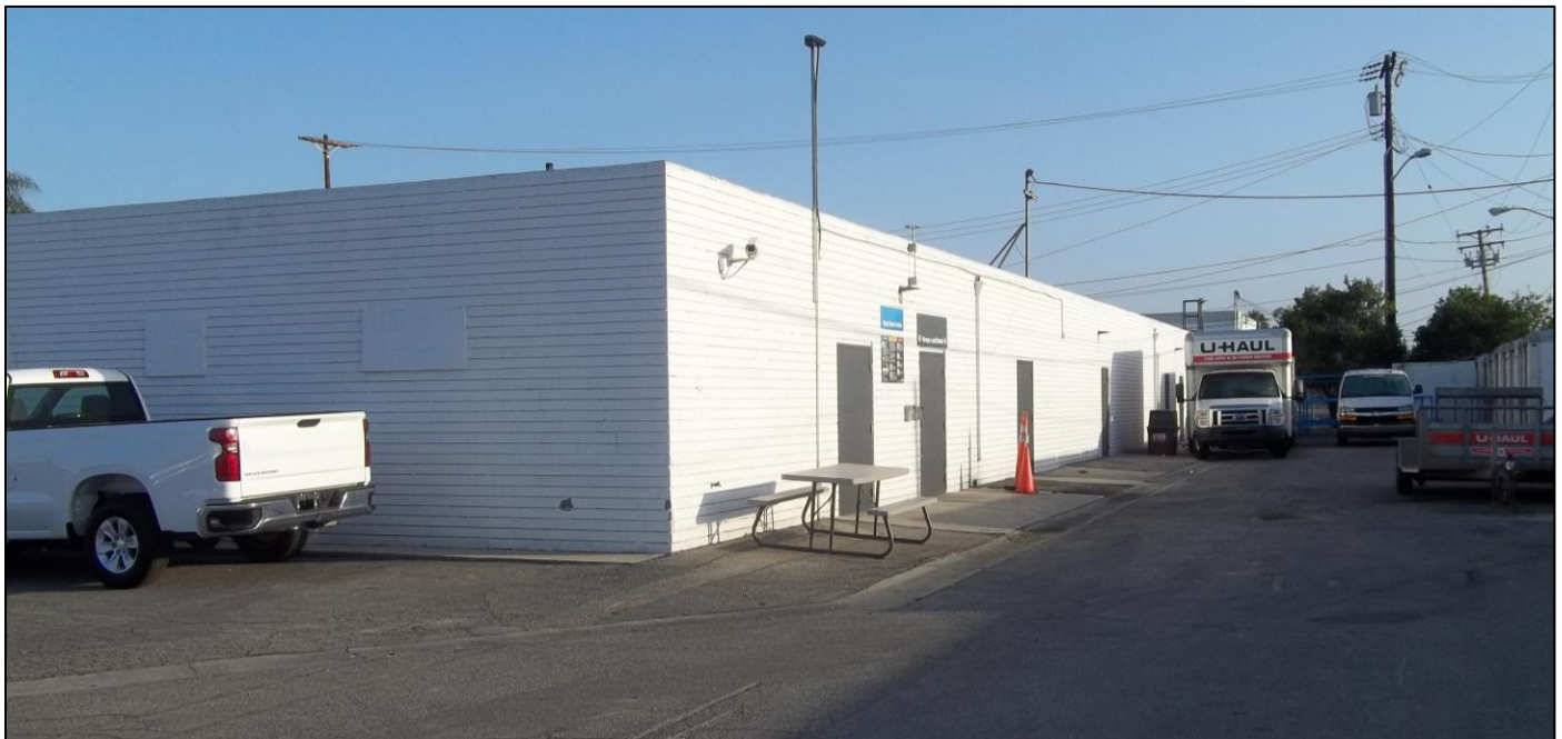
10. South elevation (left) and portion of east elevation (right) of 14202 Van Ness Avenue
