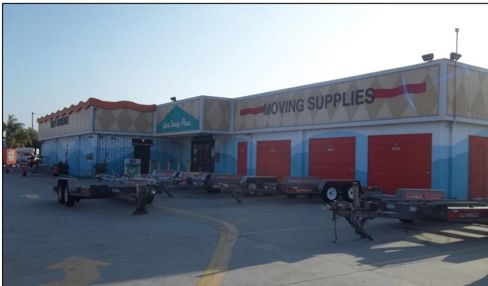
Figure 7. Main Storage, southern half of west façade
