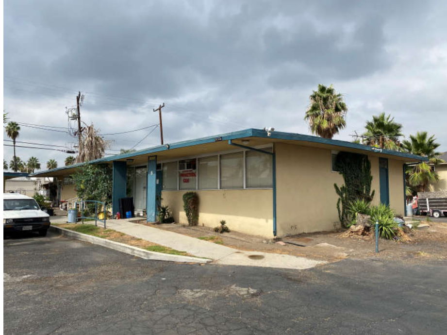
Photograph 5. Rear addition, south and east elevations; facing northwest.
