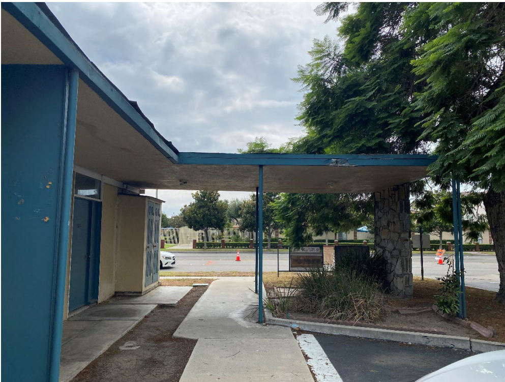
Photograph 4: View of hallway of south building. View west.
