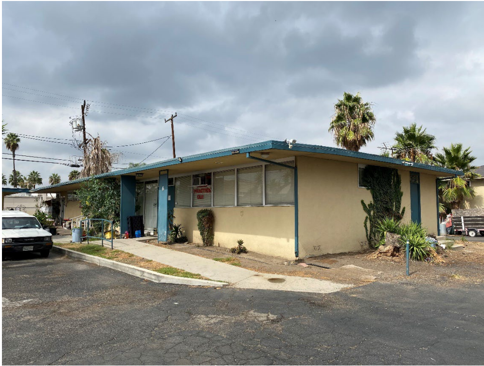
Photograph 7: Structure located at eastern end of property. View northeast.
