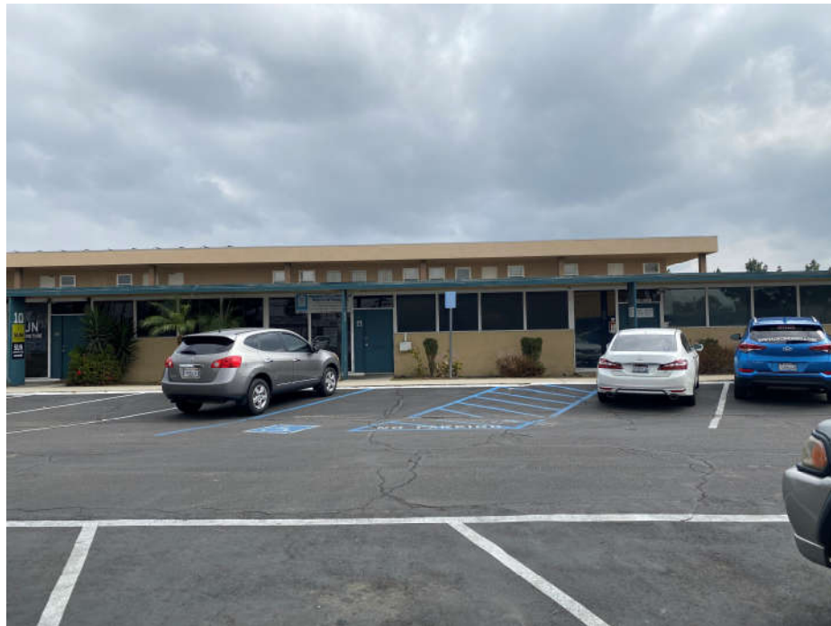
Photograph 4. 1661 West Broadway, west elevation; facing east.
