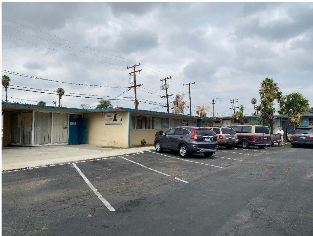
Photograph 6: View of north building. View northeast.
