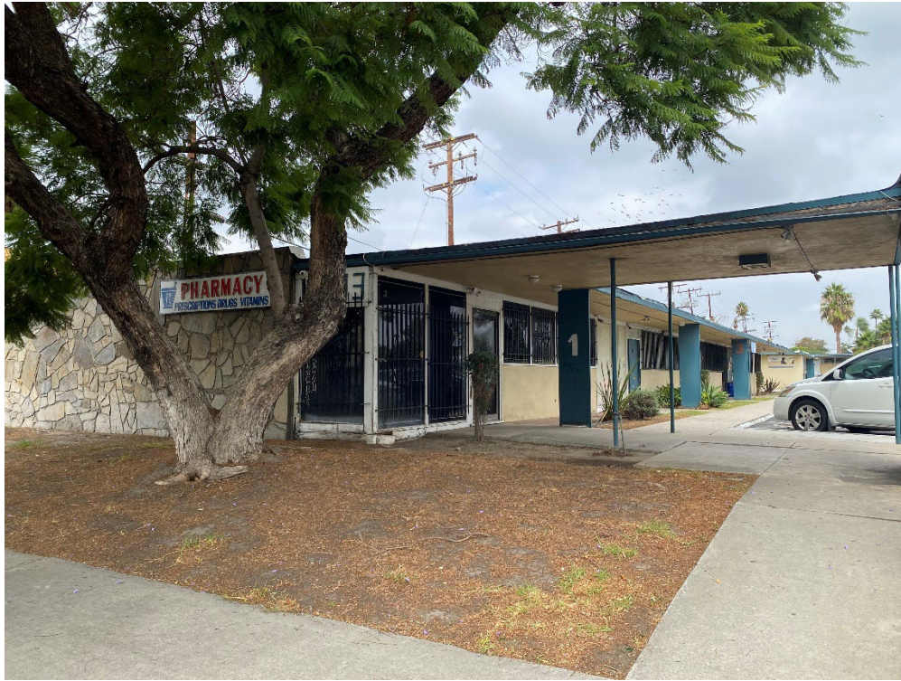
Photograph 1: View of north building. View northeast.
