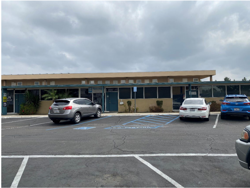
Photograph 5: View of south building. View south.
