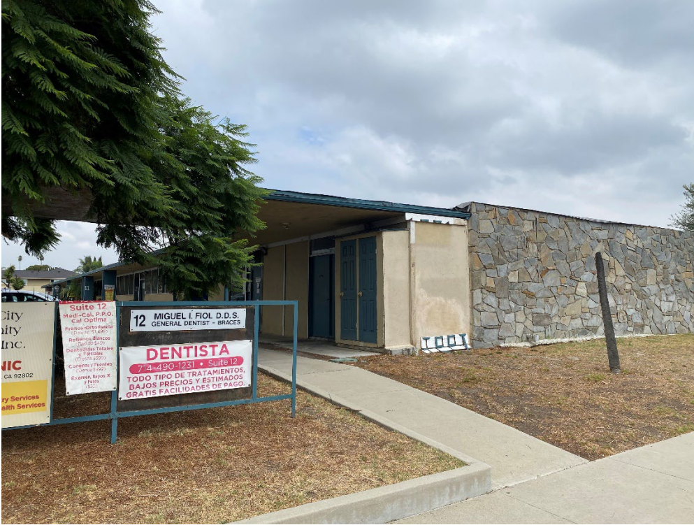
Photograph 3: View of south building. View southeast.
