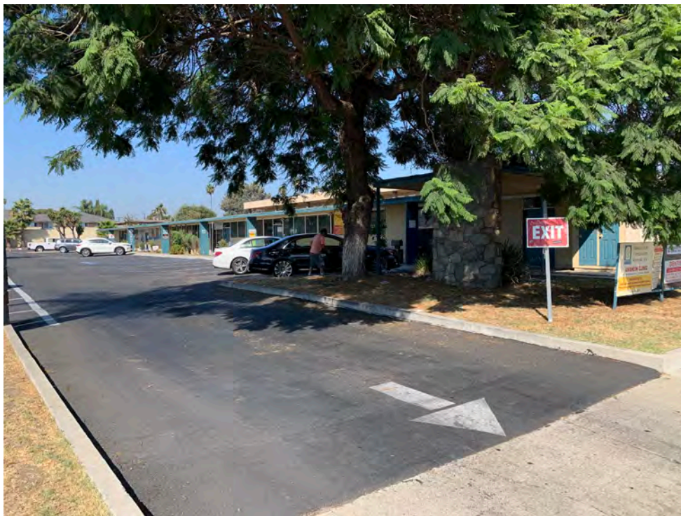
Photo #2 View of the eastern portion of the Property (Suites 8 through 14 – no Suite 13).
