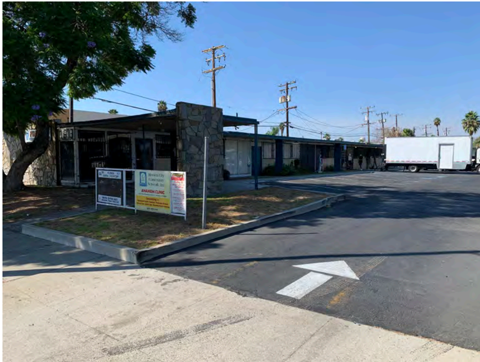
Photo #1 View of the western portion of the Property (Suites 1 through 5B).
