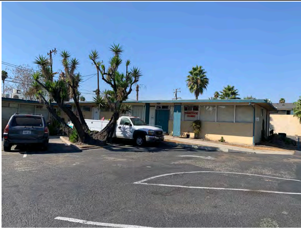
Photo #3 View of the northern portion of the Property (Suites 06A/06B/06C).
