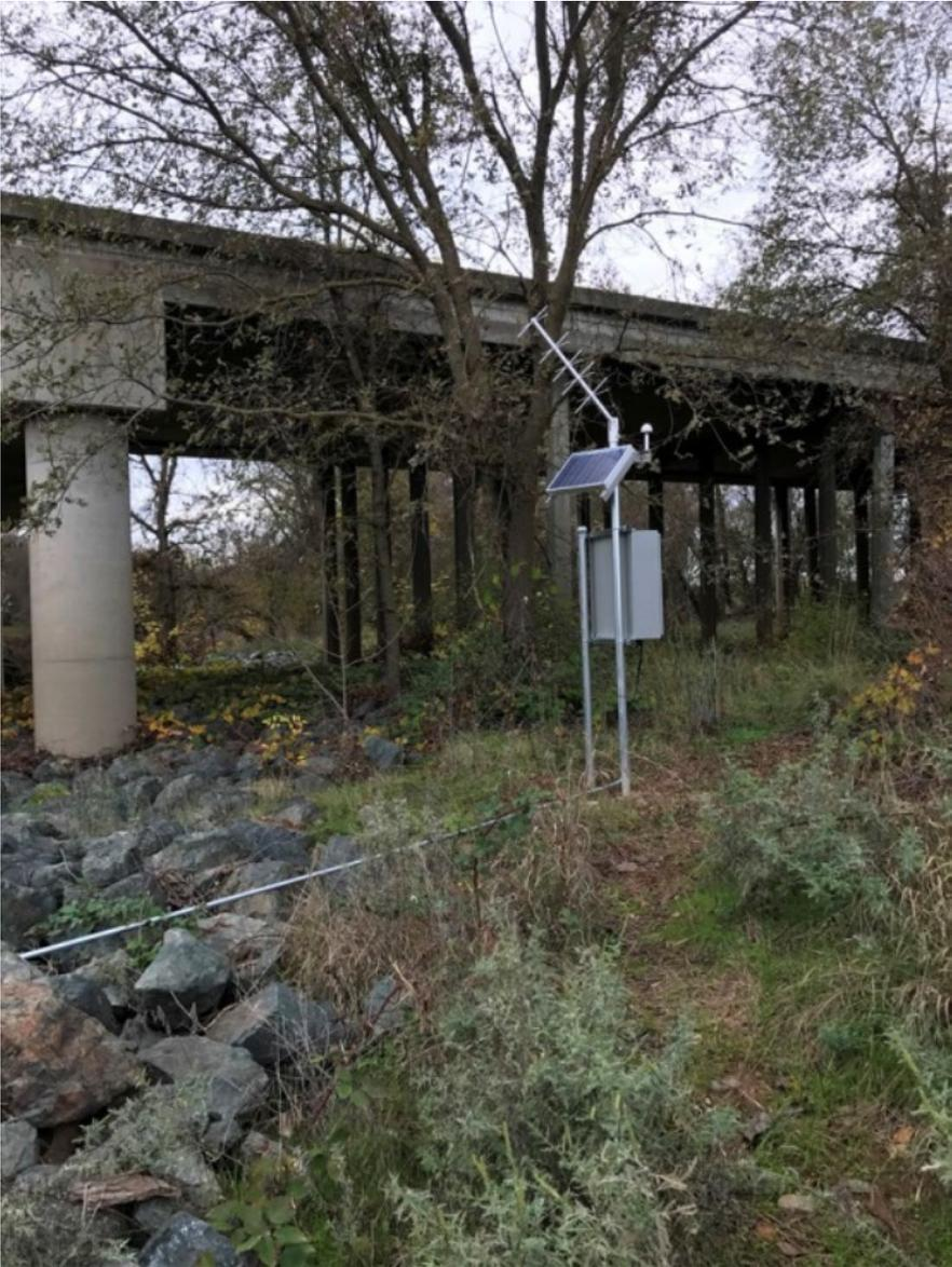
Figure 7. Example of a constructed RTU enclosure with an antenna/solar panel mast.
