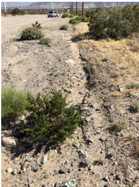
PP-11: Downstream, South-Facing View of roadside ditch near Ordinary High Water Mark Data Point (ODP)-4 along generation tie line alignment.
