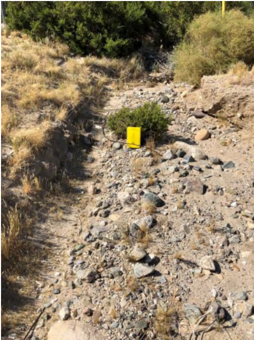
PP-9: Upstream, North-Facing View of roadside ditch outside of Review Area. Upstream of Ordinary High Water Mark Data Point (ODP)-4
