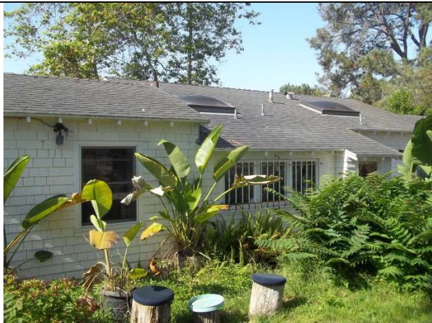
11. Residence, east half of north elevation
