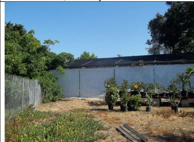
21. Greenhouse, western end of south façade
