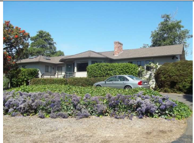
2. Residence, overview of southeast façade
