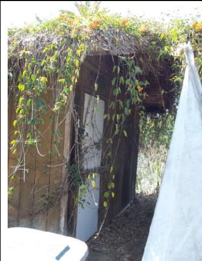
3. Administration building, west façade
