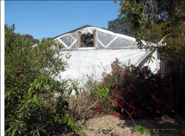
17. Greenhouse, west elevation
