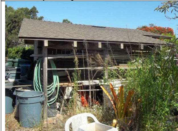
23. Ancillary building, east elevation
