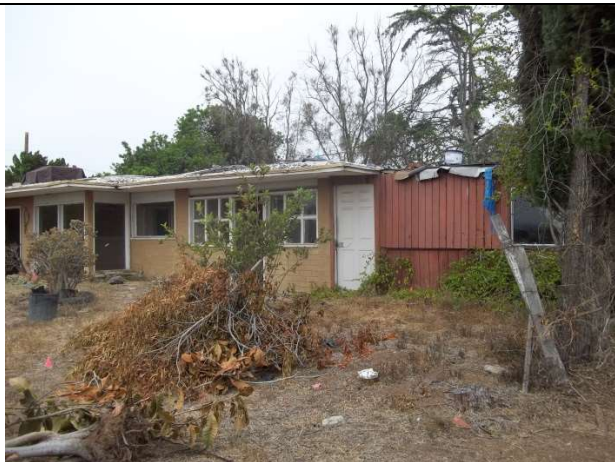
17. Main building, overview of northern half of eastern elevation
