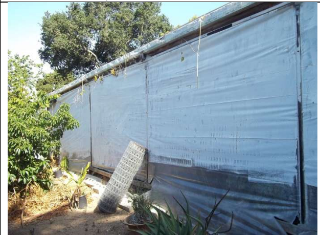
19. Greenhouse, south façade
