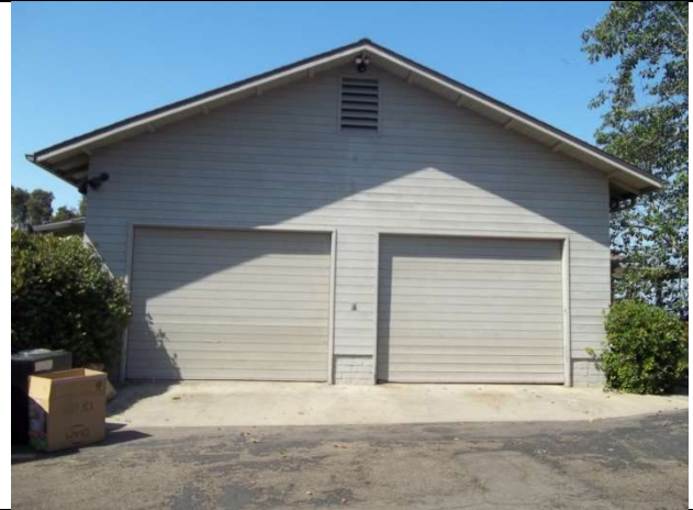
4. Residence, northeast elevation
