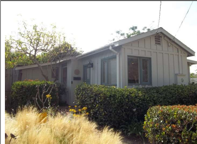
1. Residence, north façade (left) and west elevation (right)
