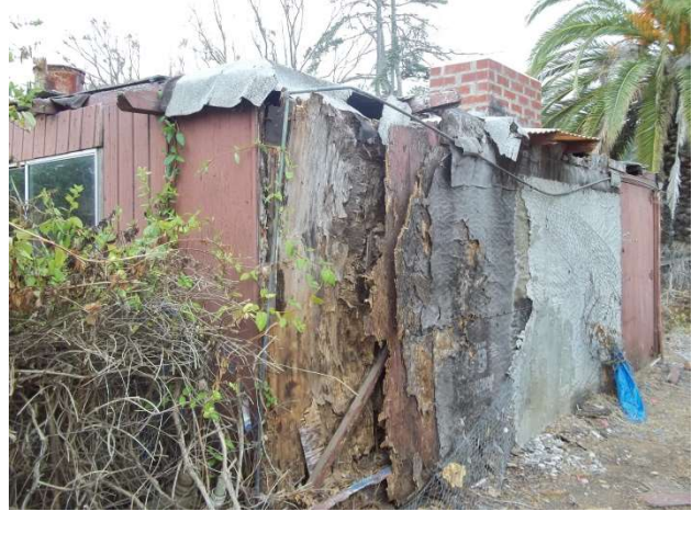
16. Main building, north elevation
