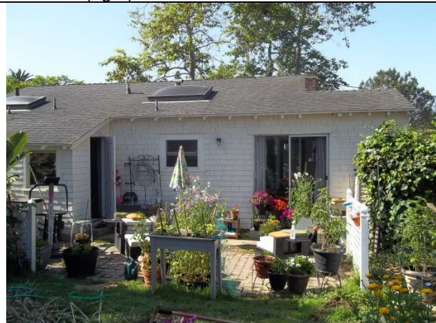
12. Residence, west half of north elevation
