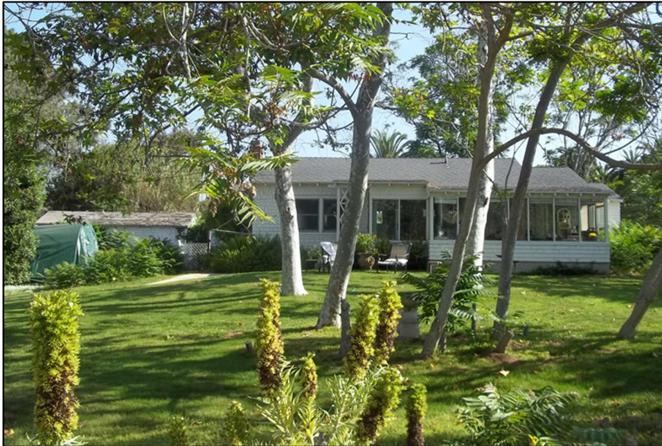
Figure 11. 1220 Melba Road, south façade, facing north
