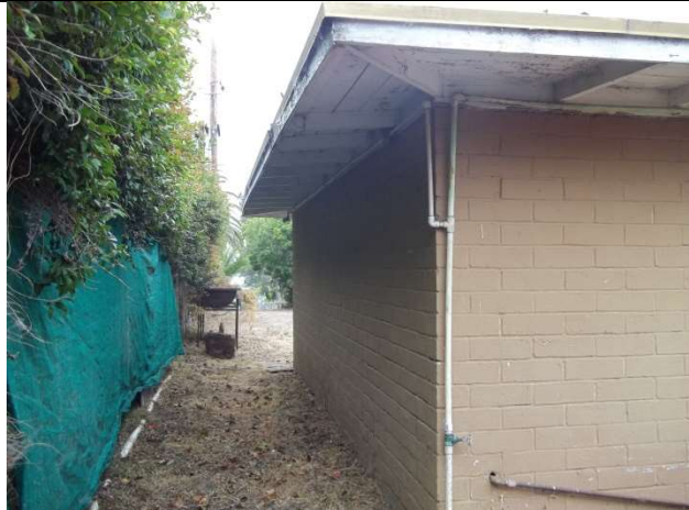
5. Ancillary building, south elevation (left) and east elevation (right)
