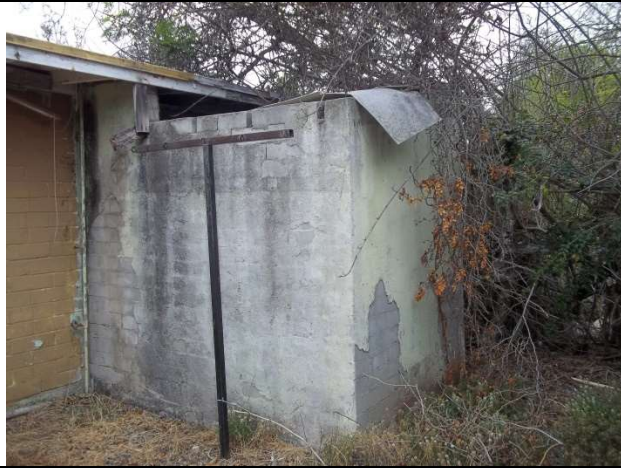
7. Ancillary building, east elevation
