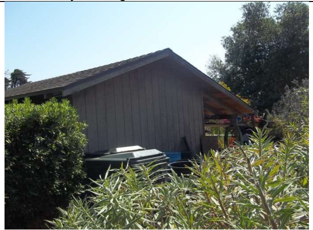
24. Ancillary building, south elevation
