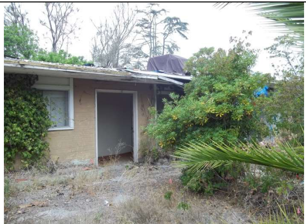
18. Main building, east elevation
