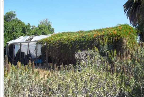
6. South elevations of greenhouse (left) and administration building (right)
