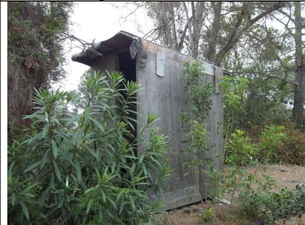
21. Shed, south façade (left) and east elevation (right), facing west
