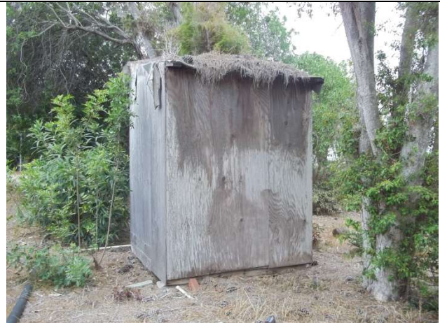
22. Shed, north elevation
