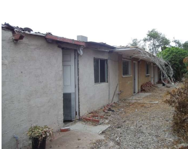
15. Main building, overview of west façade, facing southeast
