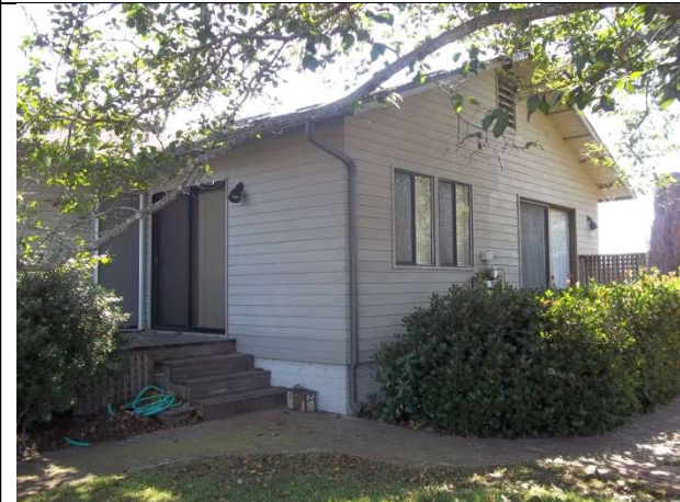
9. Residence, northwest elevation (left) and southwest elevation (right)
