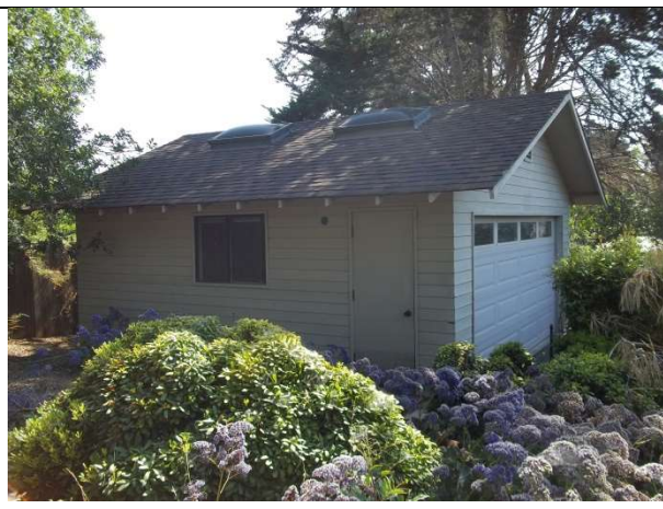
18. Garage, west elevation (left) and south façade (right)
