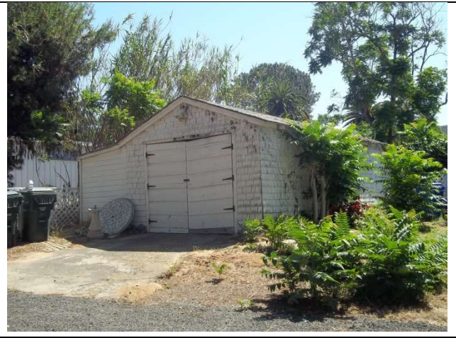
14. Detached ancillary building
