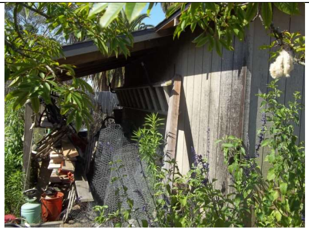
22. Ancillary building, east elevation
