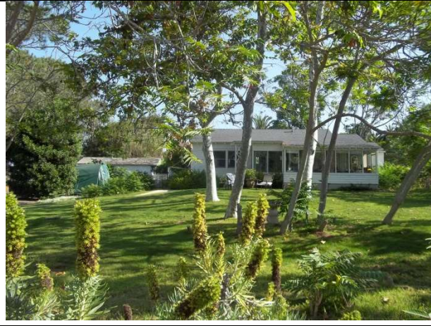
2. Overview of 1220 Melba Road, south façade
