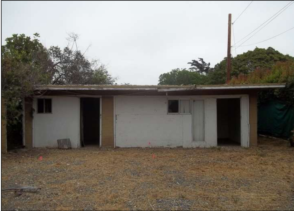
Figure 8. 1190 Island View Lane, large ancillary building, west facade, facing east
