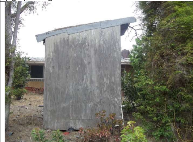
23. Shed, west elevation
