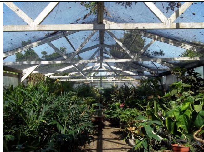
24. Interior, western half of greenhouse
