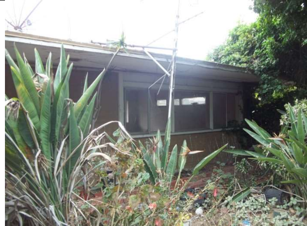
12. Main building, south end of west façade
