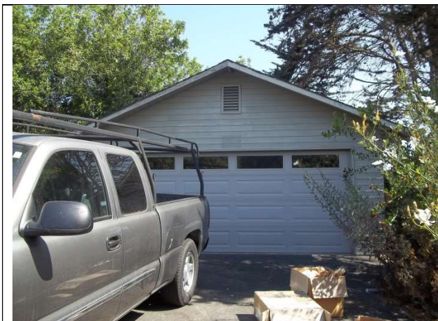
17. Garage, south facade
