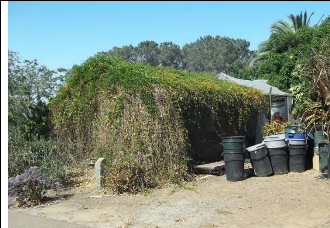
1. Administration building, east elevation (left) and north elevation (right)
