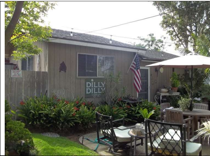
1. Residence, west façade
