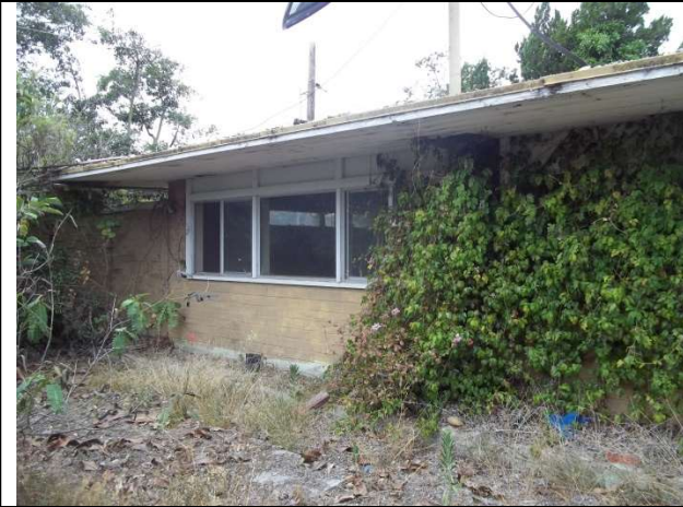
19. Main building, southern end of east elevation
