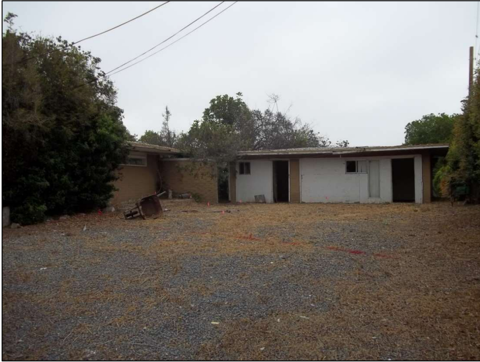
Figure 7. Partial site overview of 1190 Island View Lane, facing east
