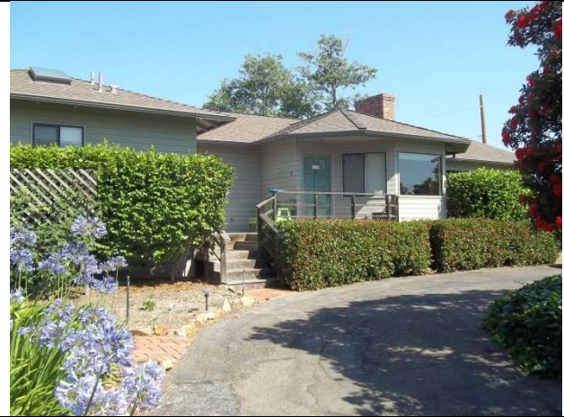
3. Residence, northern end of southeast façade
