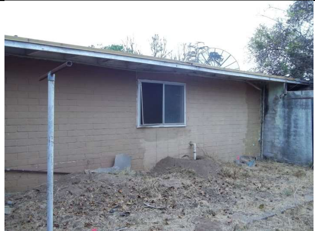
6. Ancillary building, east elevation
