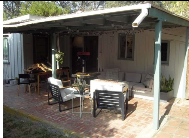
4. Residence, east elevation with porch overhang
