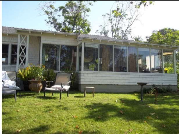
3. Residence, east side of south façade (sunroom)
