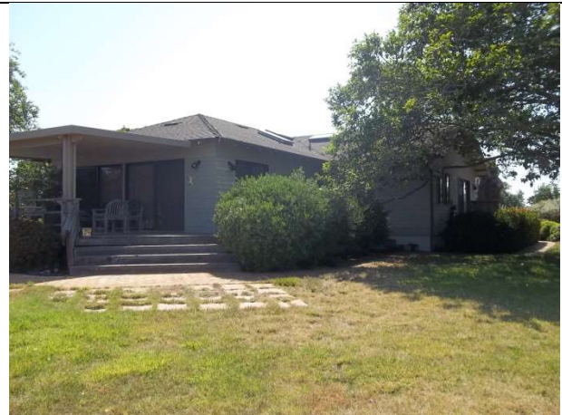
8. Residence, northwest elevation (left) and southwest elevation (right)
