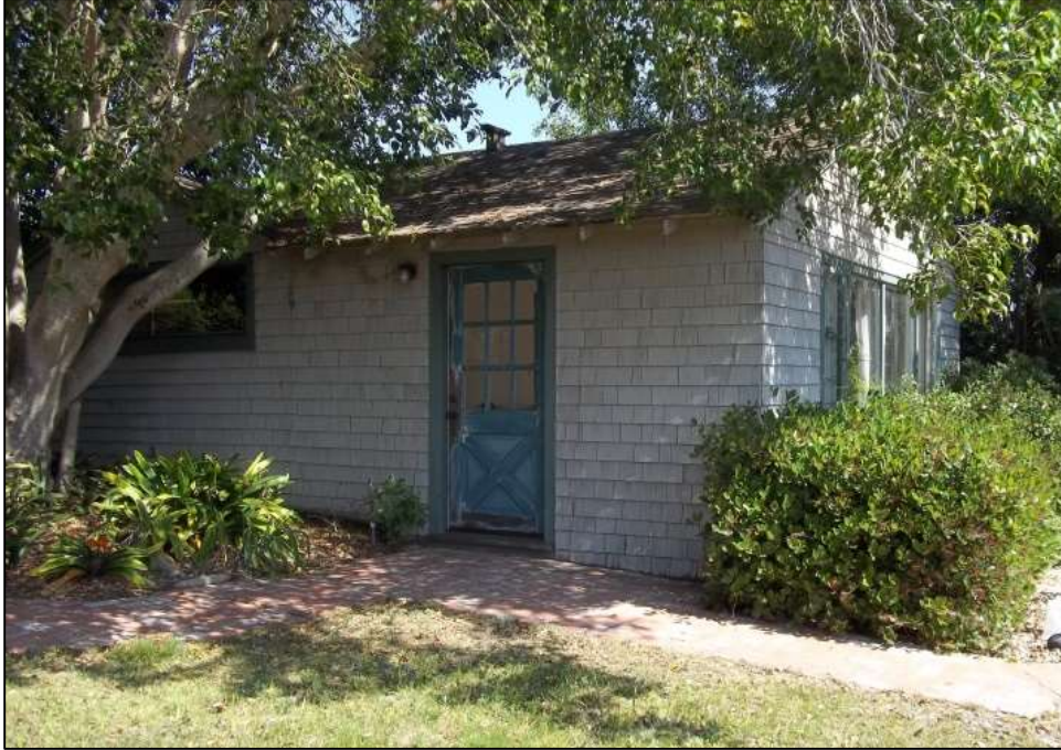
Figure 14. 1240 Melba Road, guest house, south façade
