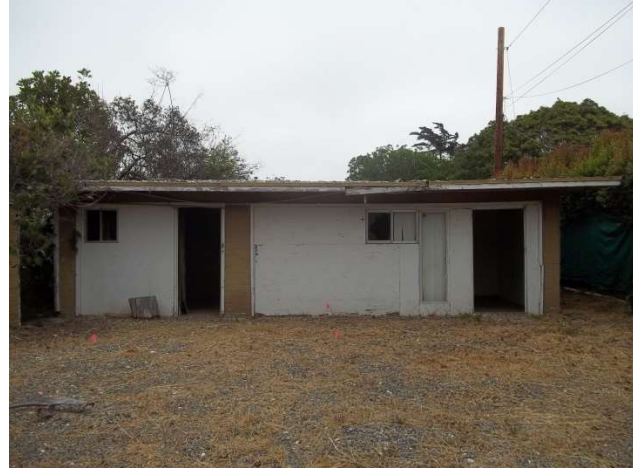
4. Ancillary building, west façade, facing east
