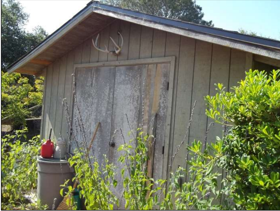
Figure 16. 1240 Melba Road , shed, north façade
