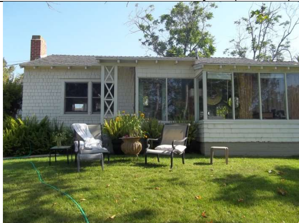
5. Residence, west side of south façade
