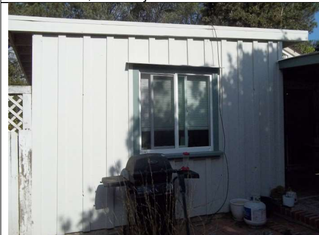
5. Residence, south end of west elevation
