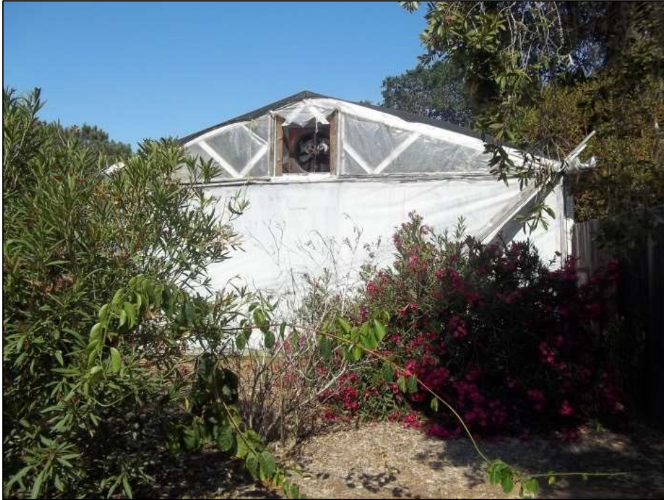
Figure 18. 1234 Melba Ave., Greenhouse, west elevation, facing east
