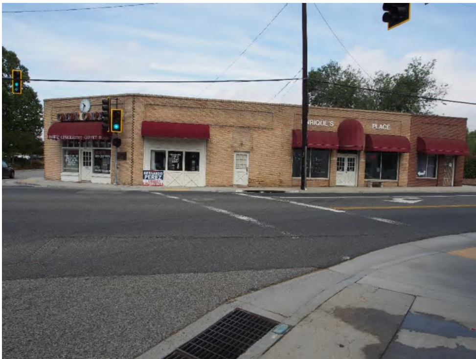
Photograph 5. Tanner Corner Building, east elevation, view west
