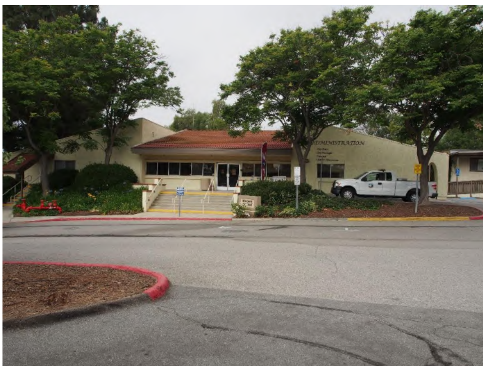
Photograph 1. Administration Building, east elevation, view west
