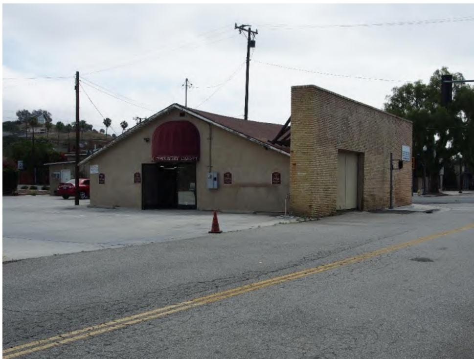
Photograph 6. Tanner Corner Building, west elevation, view east
