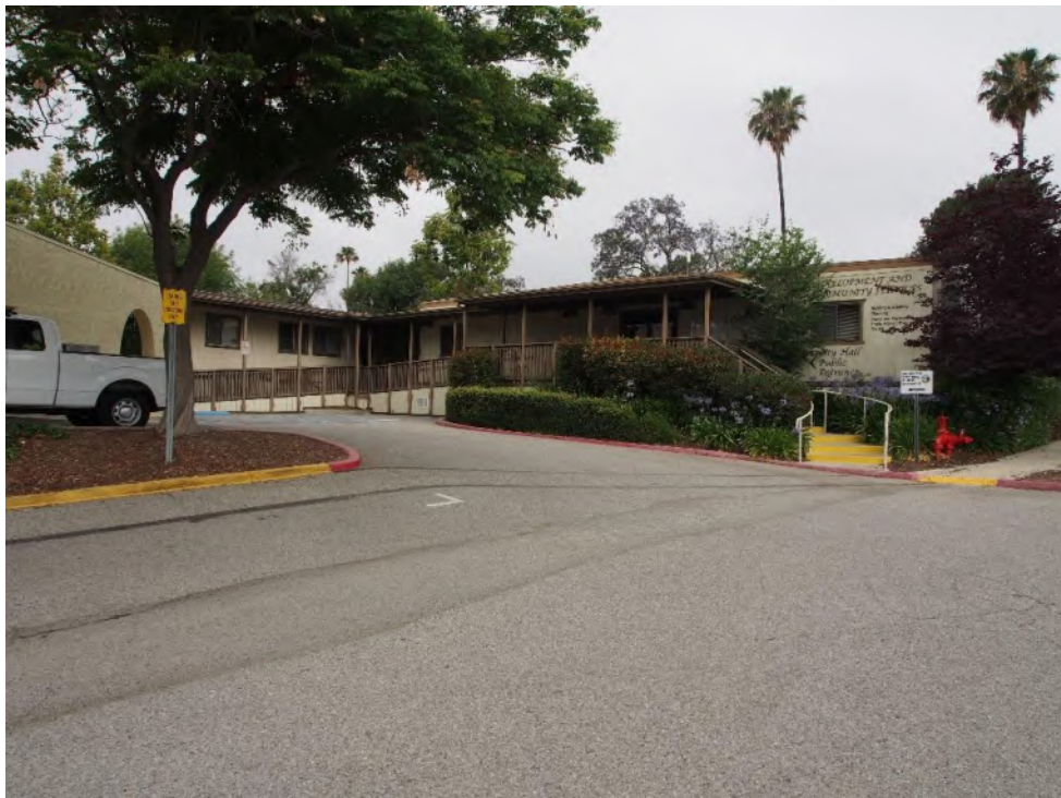
Photograph 3. City Hall temporary building, south elevation, view northwest
