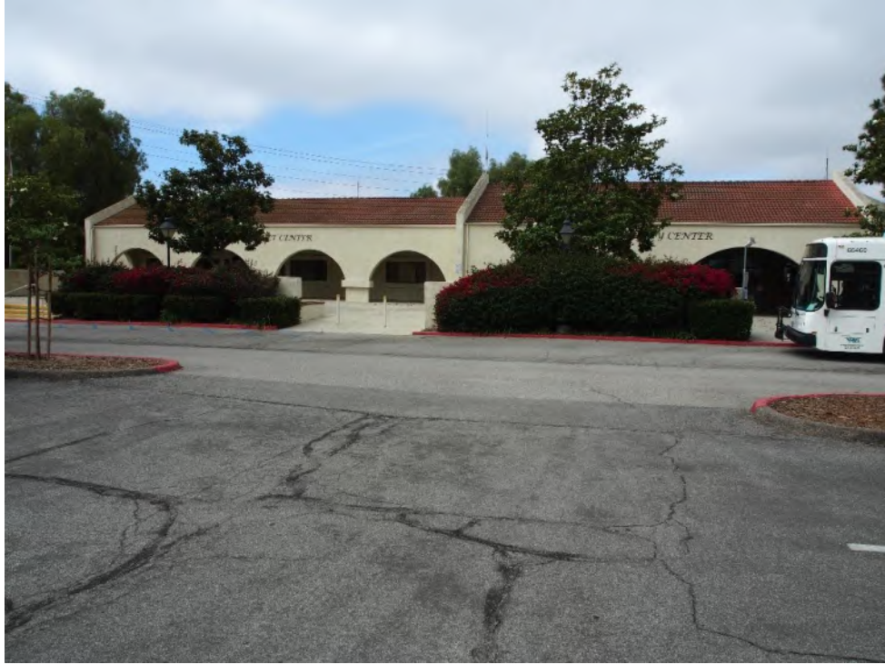
Photograph 2. Active Adult Center/Community Center, northeast elevation, view southwest
