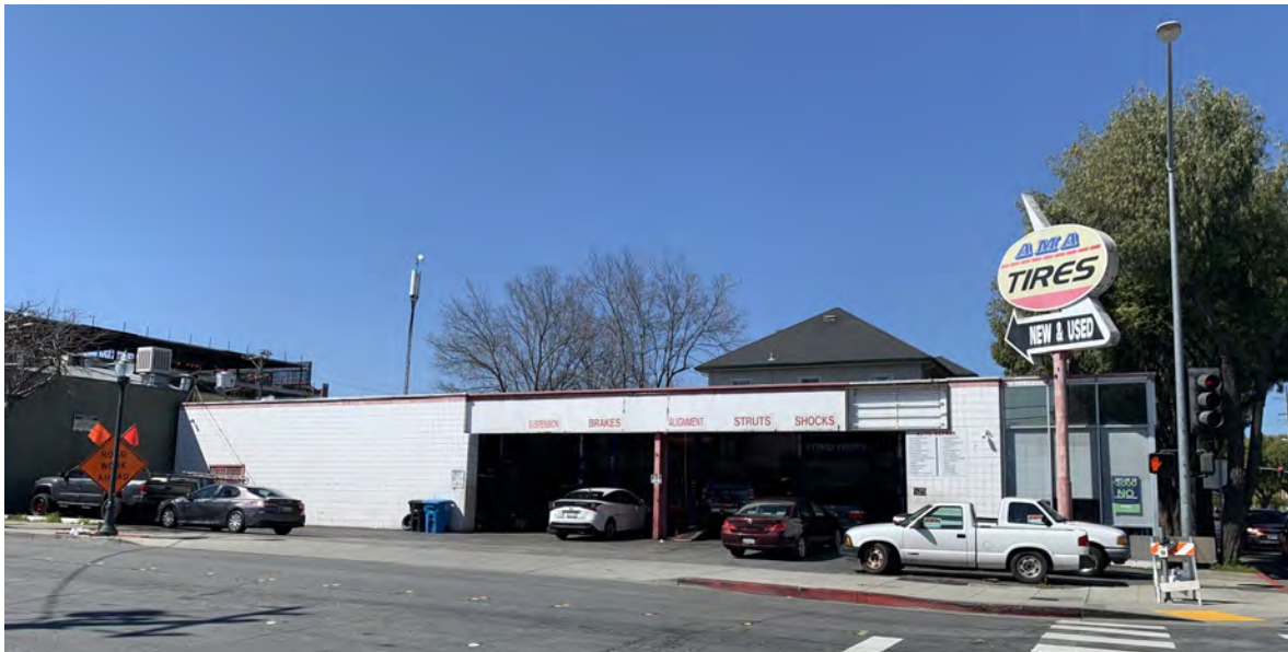
Property overview, view facing north.
