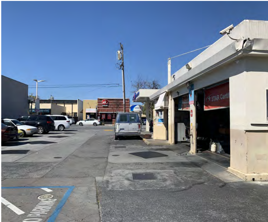
300 S. Delaware St - Rear of property, view looking north.
