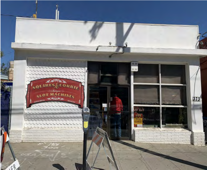
373 S. Claremont St. – Primary facade, view facing east.
