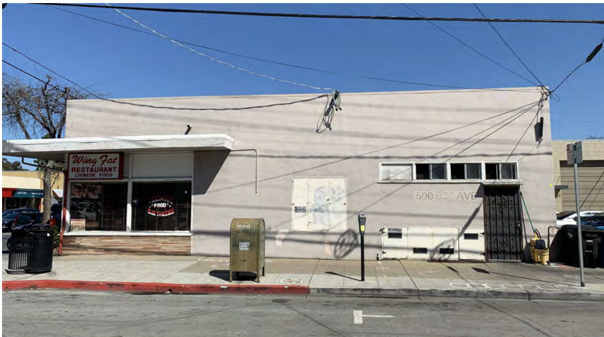
500 E. 3rd Ave. West facade, view facing east.
