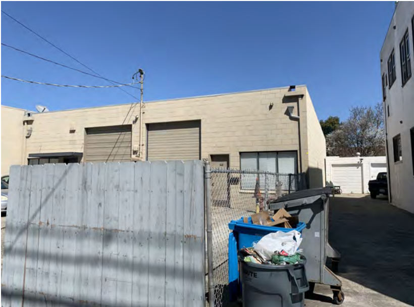
307 S. Claremont St. Property overview, view facing east.
