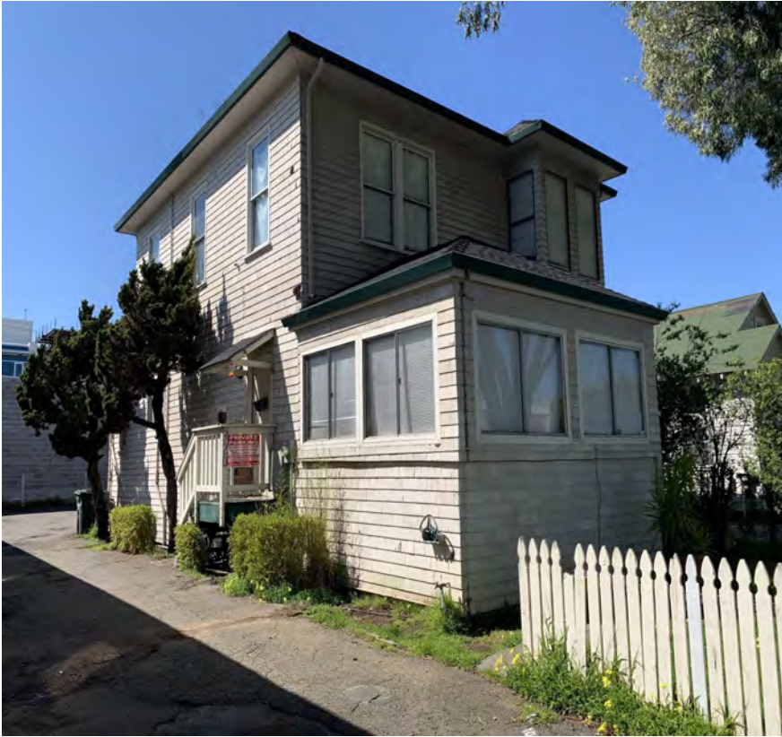
320 S. Delaware St. Property overview, view facing northwest.
