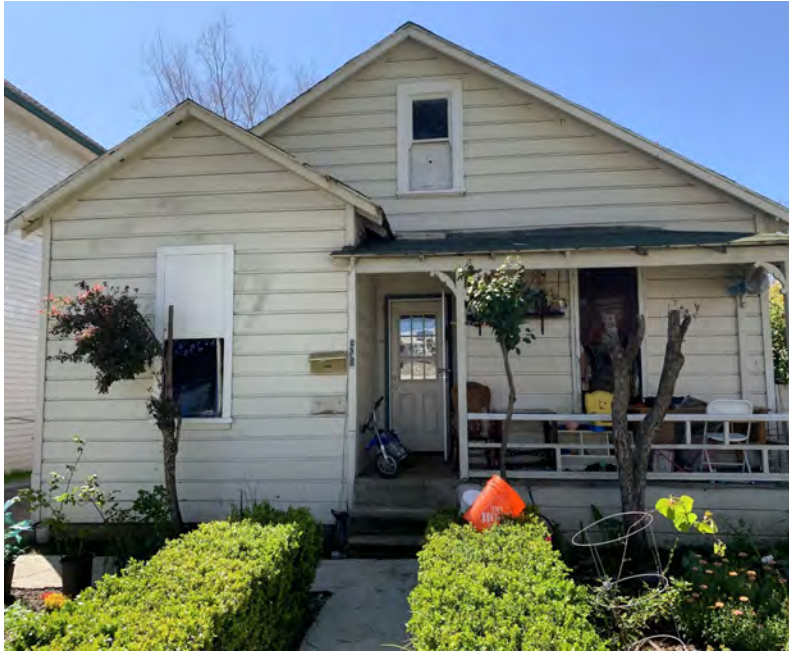
318 S. Delaware St – Primary facade, view facing west.
