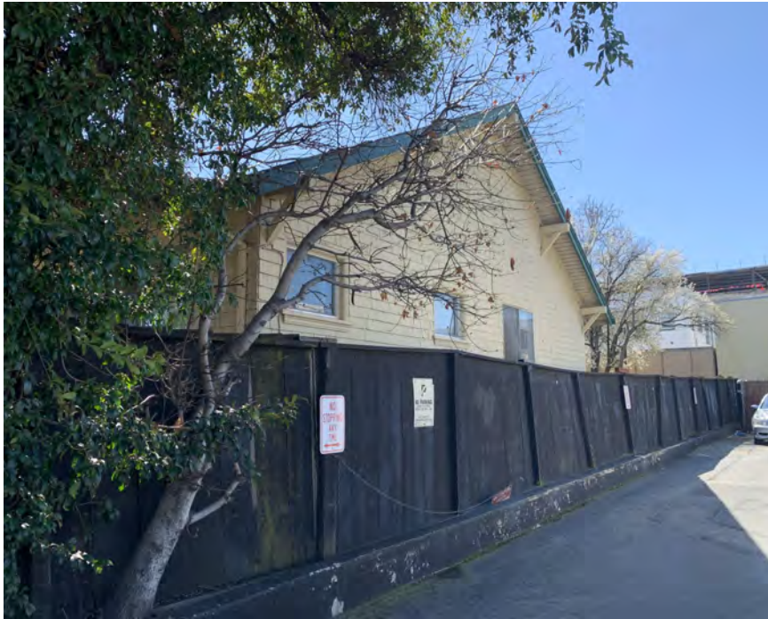
312 S. Delaware St. - North facade, view facing southwest.
