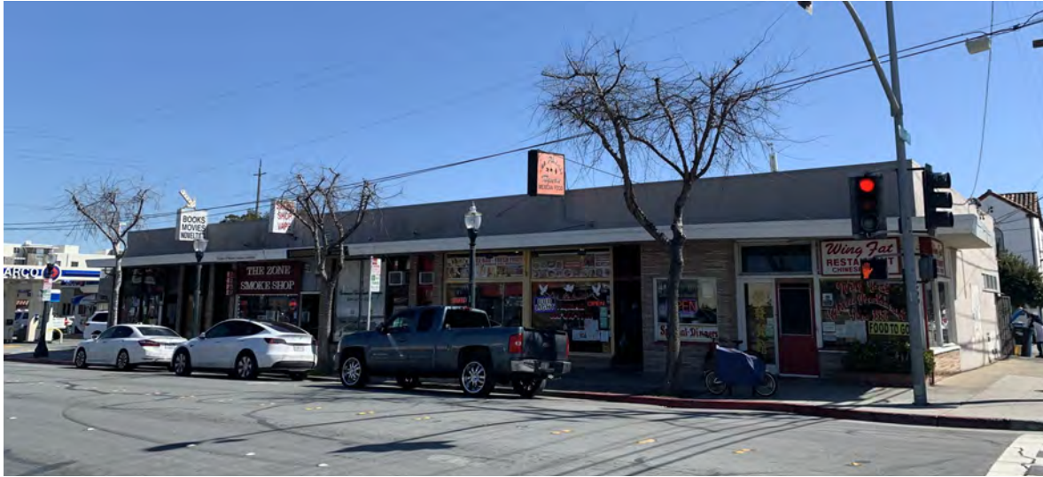
500 E. 3rd Ave. Storefronts on north facade, view facing southeast.
