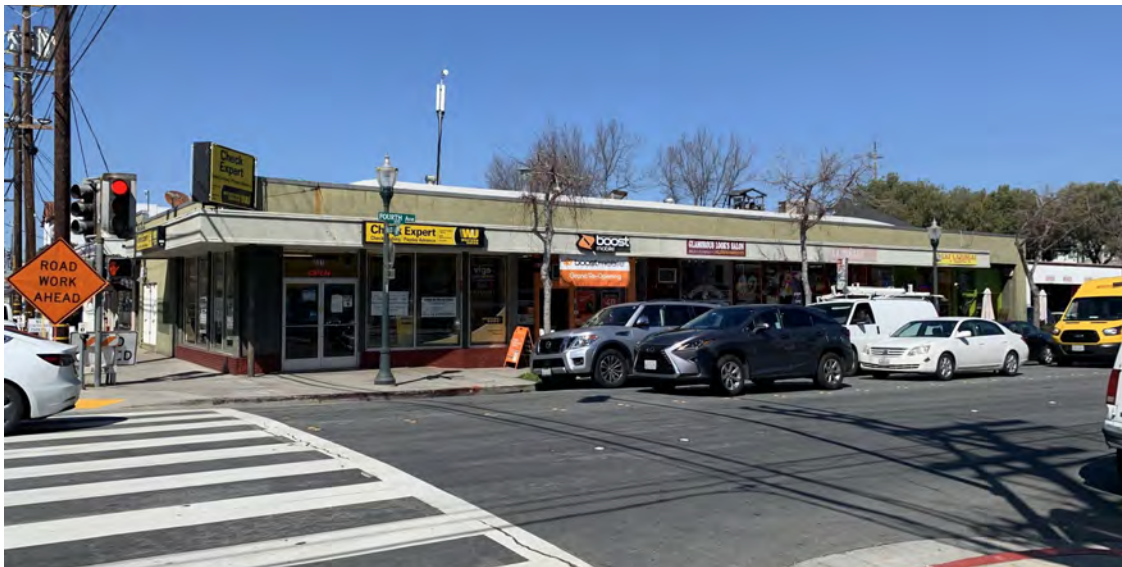
511 E. 4 th Ave. - Property overview, looking northeast.
