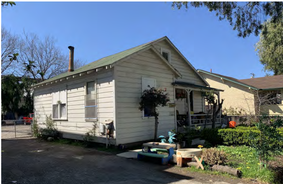
318 S. Delaware St - Property overview, view looking northwest.
