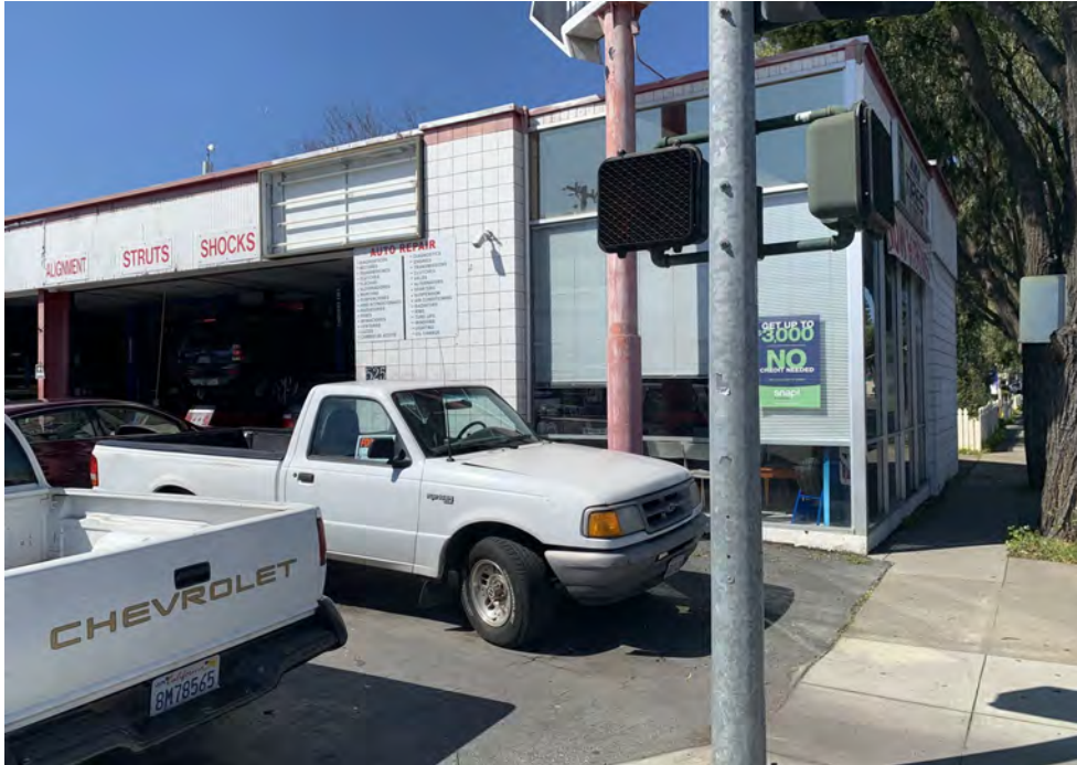
Detail of corner; view facing northwest.
