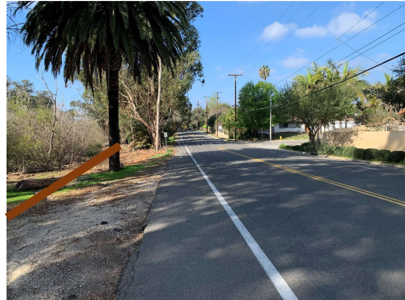
b. Bike path alignment near Encore Drive (east), facing west
