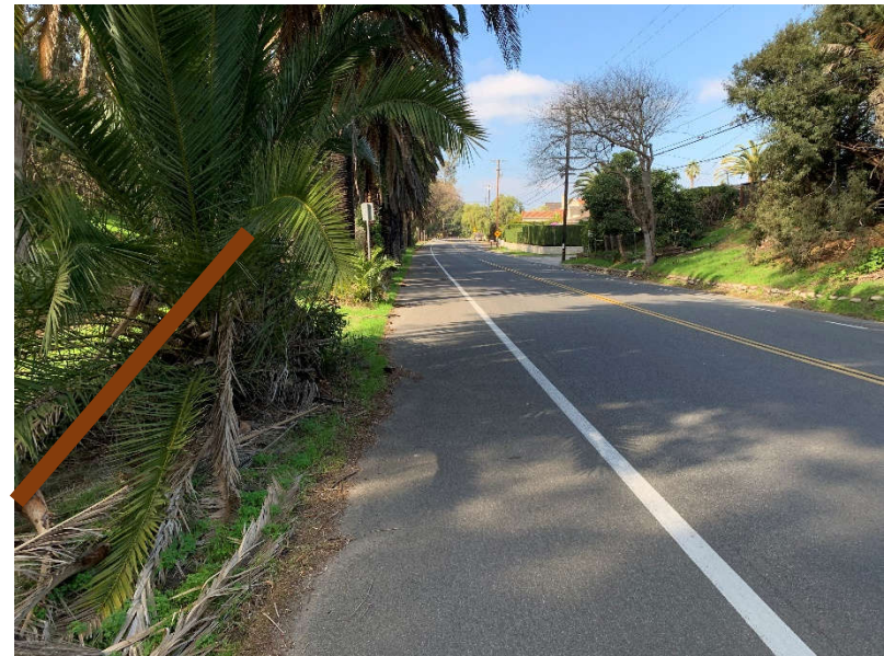
d. Bike path alignment (~300 feet west of 3.c), facing west
