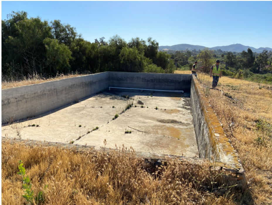
Photograph #7 Irrigation reservoir within the north central portion of the Site.
