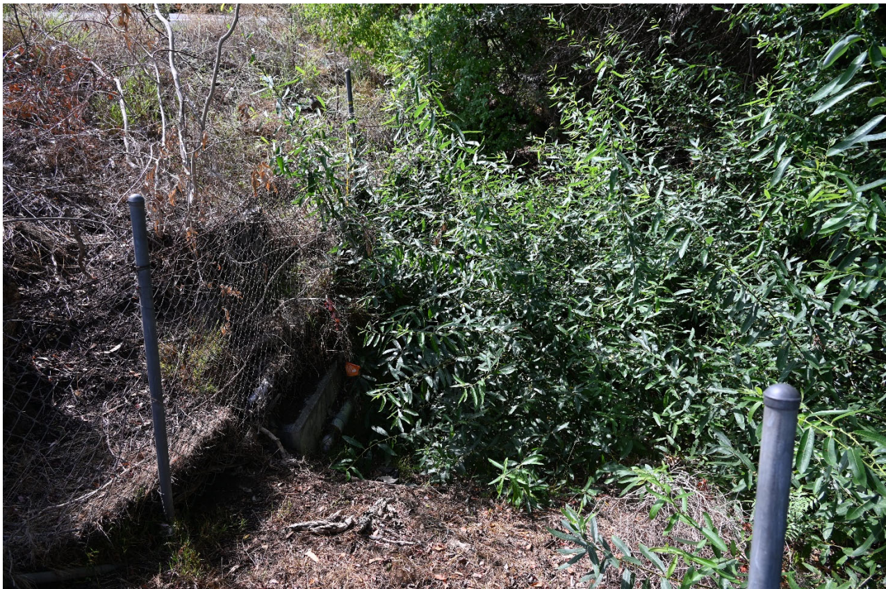
Figure 2. North Santa Fe Avenue Culvert Outlet at POC B
