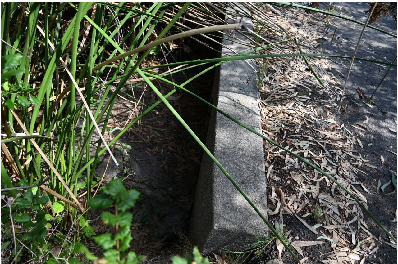
Figure 6. Roadway Culvert Crossing between Reach 2 and 3 (Permanent Grade Control)
