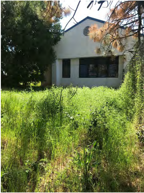
Photo 67. View to the south across the Site, beyond which is a National Guard building. (March 2022).
