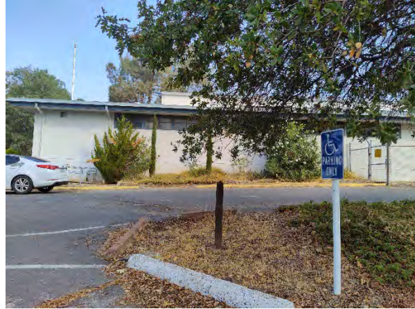
Photo 78. View looking northwest towards main building from parking lot (July 29, 2021).
