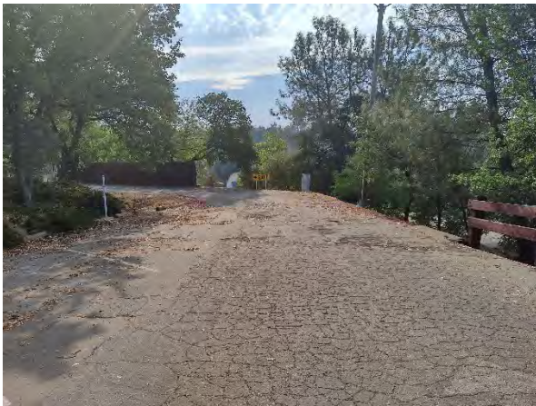
Photo 89. View looking east along driveway and southern perimeter of Site towards eastern perimeter of Site (July 29, 2021).
