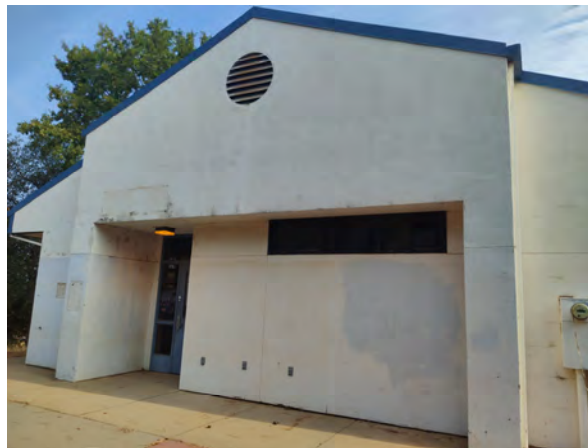
Photo 5. View facing north of southern exterior of auxiliary building (July 29, 2021).
