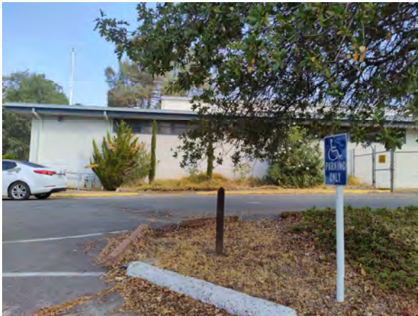
Photo 1. View looking northwest towards main building from parking lot (July 29, 2021).
