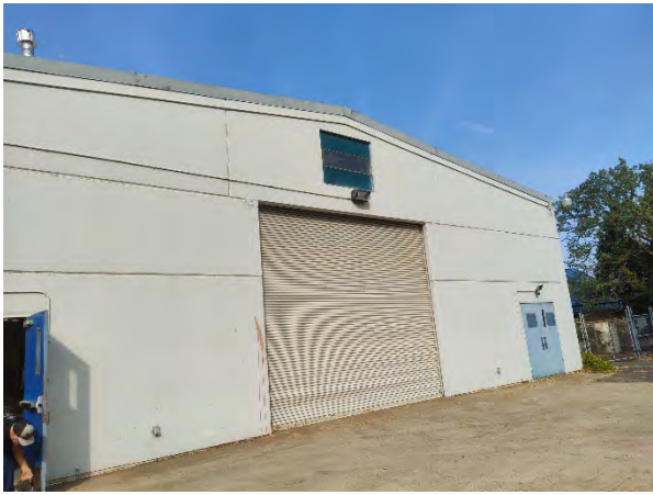
Photo 21. View looking northwest of exterior of eastern side of main building (July 29, 2021).
