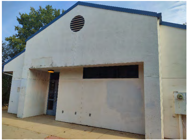
Photo 22. View facing north of southern exterior of auxiliary building (July 29, 2021).
