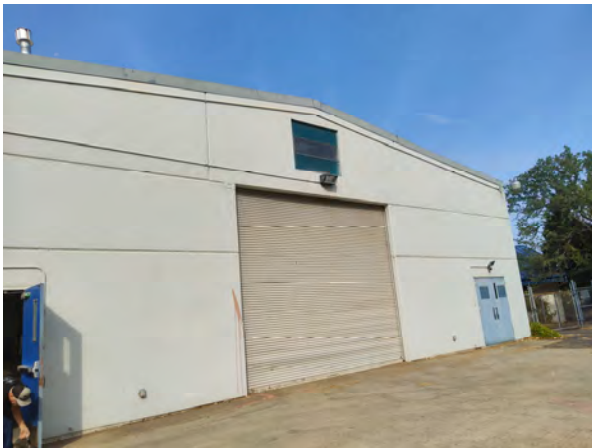
Photo 4. View looking northwest of exterior of eastern side of main building (July 29, 2021).
