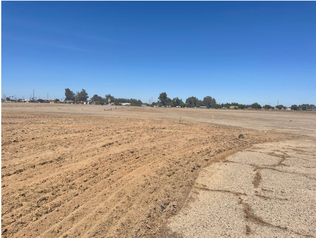
Combination of asphalt and sandy loam sediment in middle of project site. View to west. June 11, 2021.
