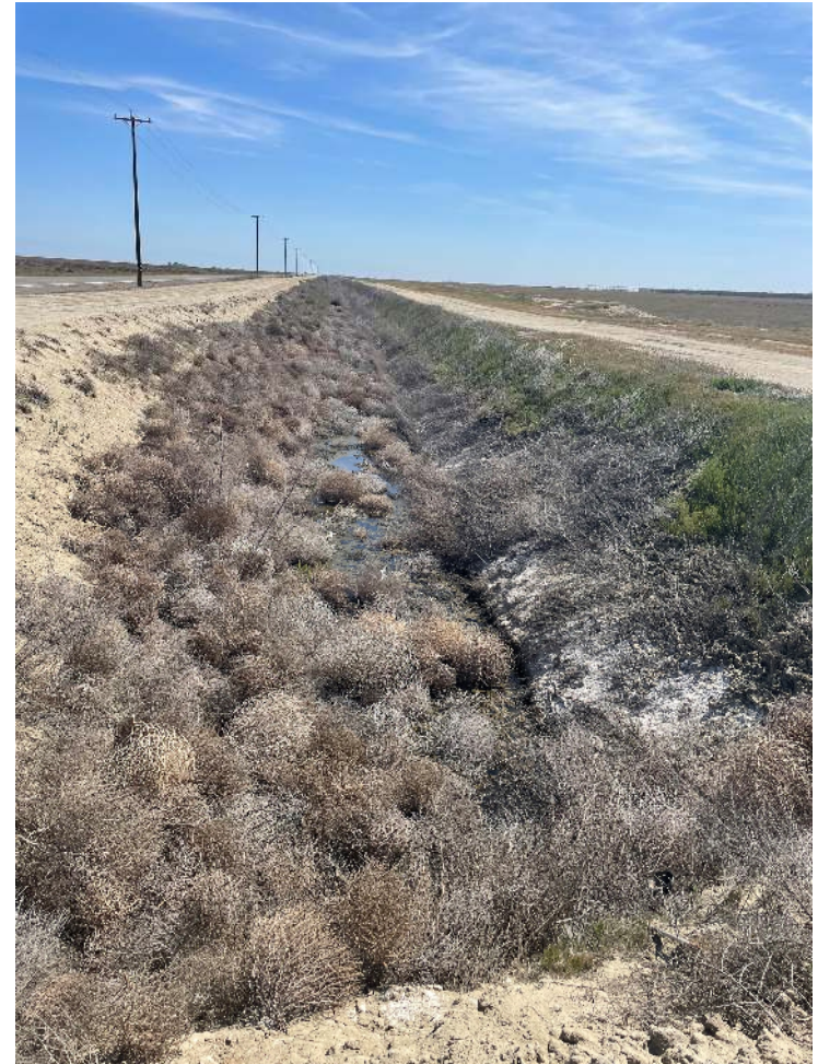
View of offsite canal along northern boundary
