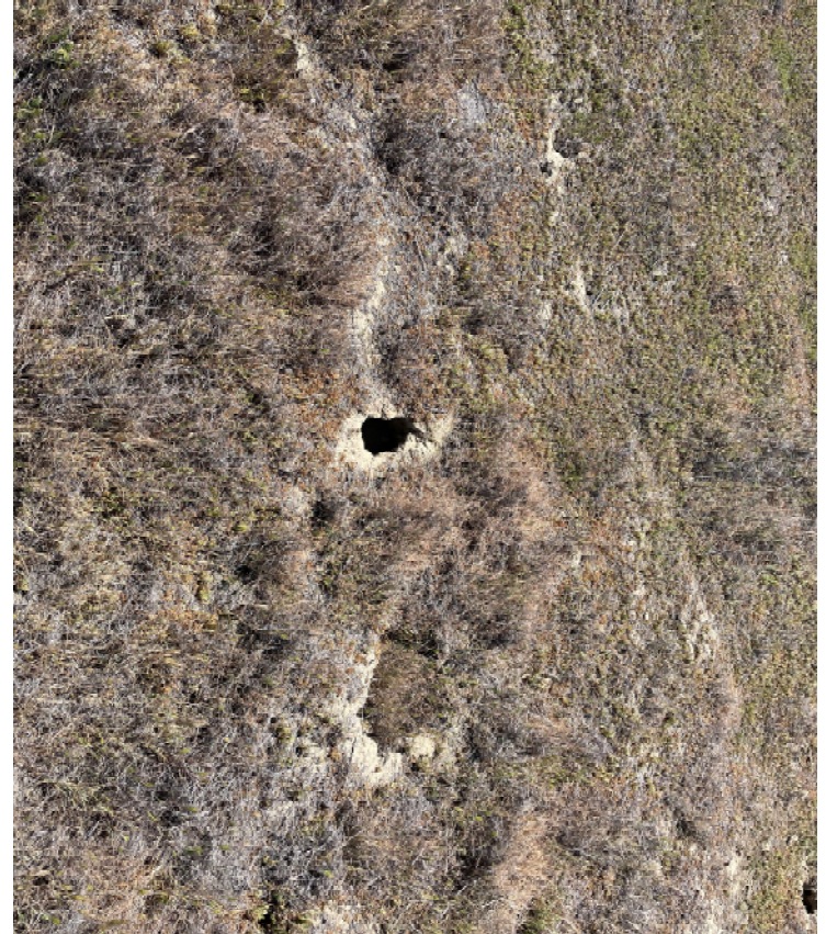
View of typical rodent hole at Site
