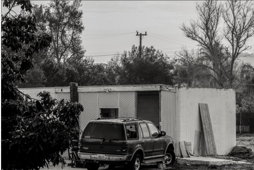
Photo 2: 3/4 View Noting Wood Lattice Enclosure of Office Porch and Entrance View Southeast. DSC7169
