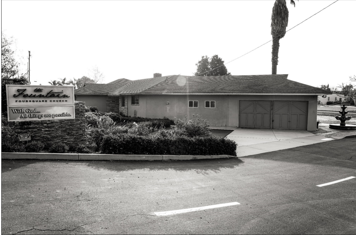
Photo 1: 11930 3/4 View of North Elevation. View East-Southeast
