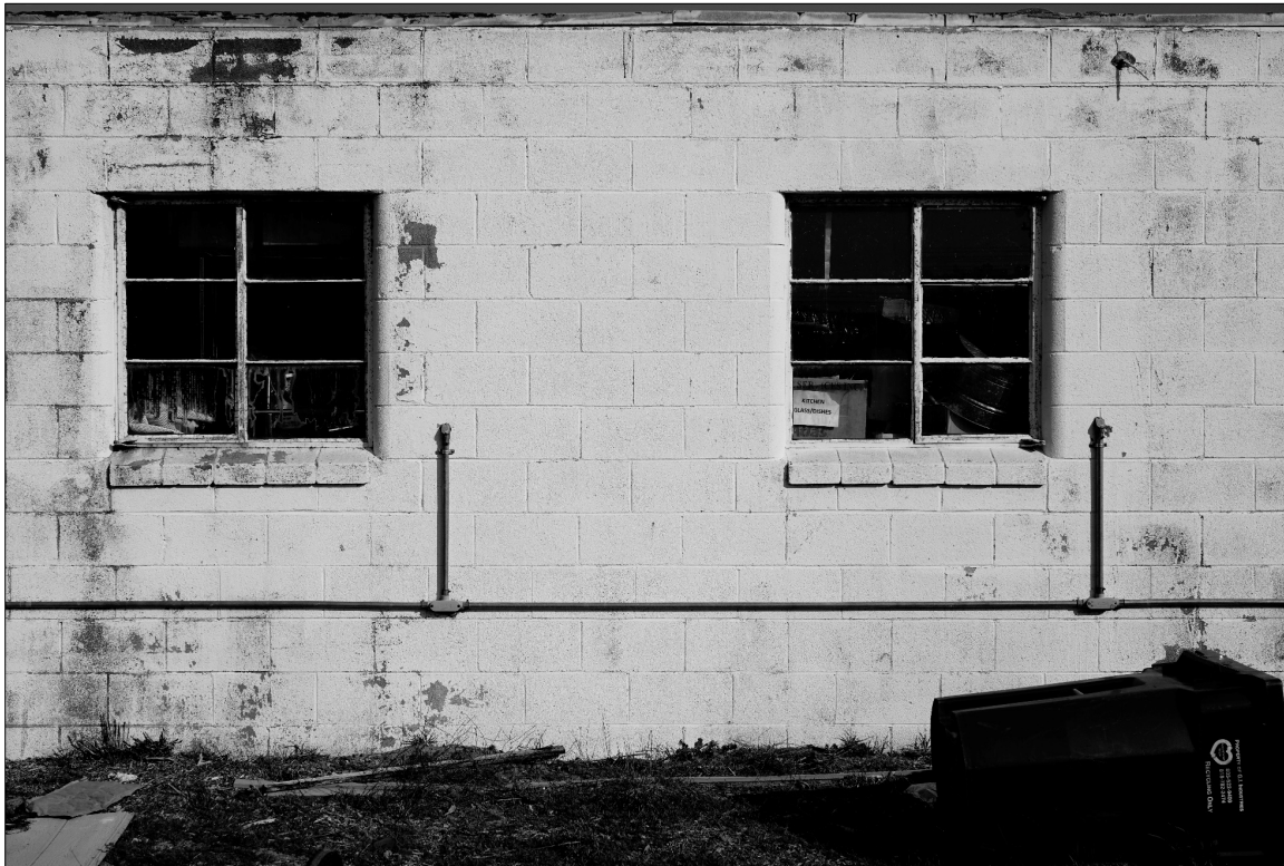
Photo 19: Detail of Window Sets in South Wall. View North
