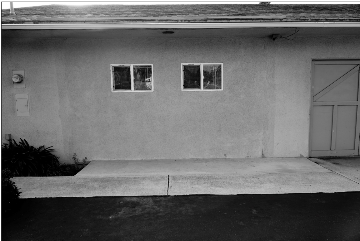
Photo 4: Area of Possible Remodel Adjacent to Garage Doors. View South-Southeast
