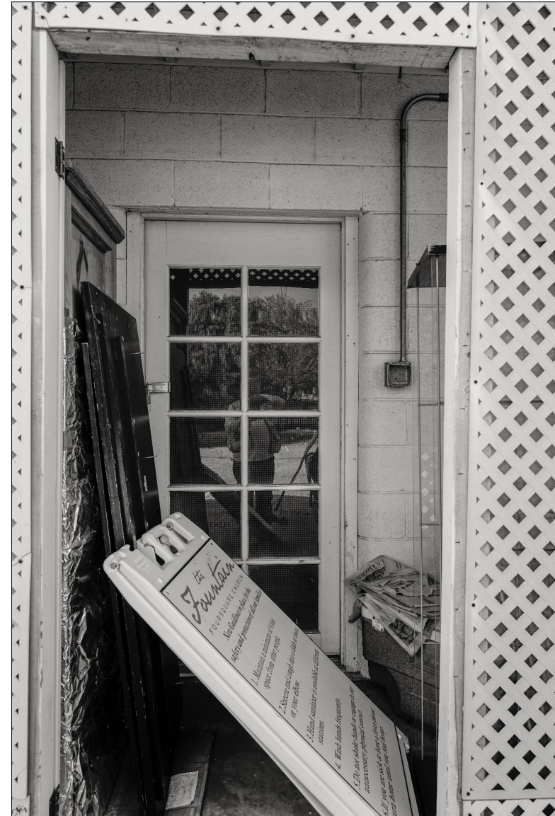
Photo 21: Detail View of Front Door to Office of Garage. View South
