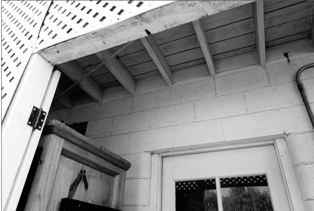
Photo 7: Detail View of Office Entrance. Note Rafters and Board Sheathing. DSC7196
