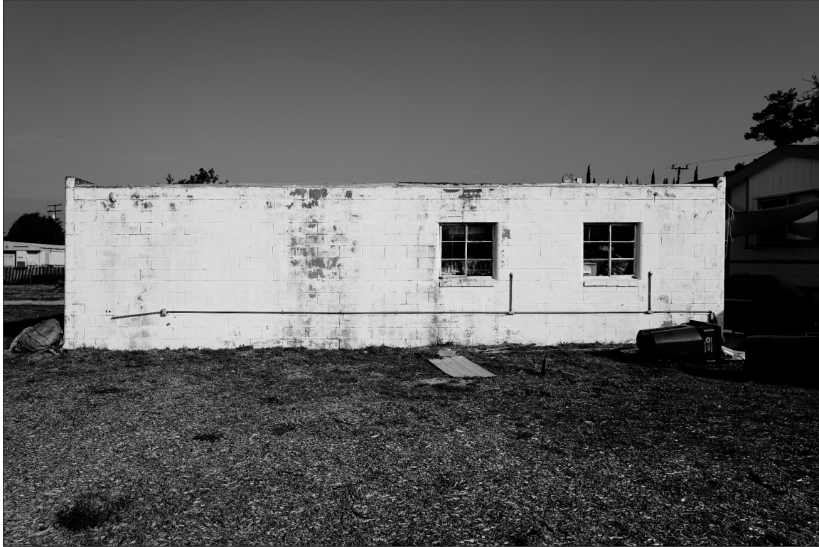
Photo 18: South Elevation of Garage. View North
