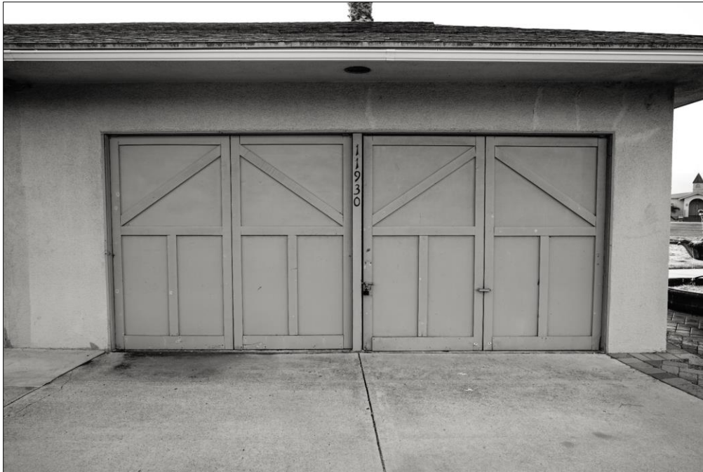
Photo 2: Replacement Garage Doors in Original Framing. View South-Southeast. DSC7110
