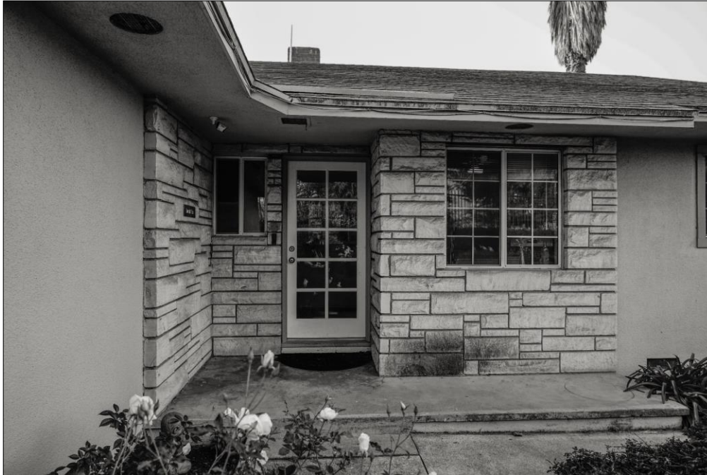
Photo 1: Formalized Entrance. View South. DSC7105
