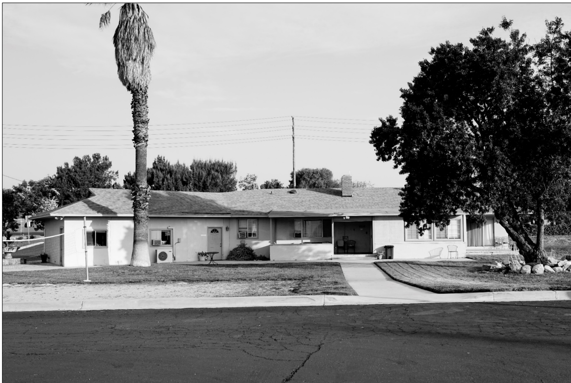
Photo 6: South Elevation. Note Partially Enclosed Patio Porch, Numerous AC Units. View North
