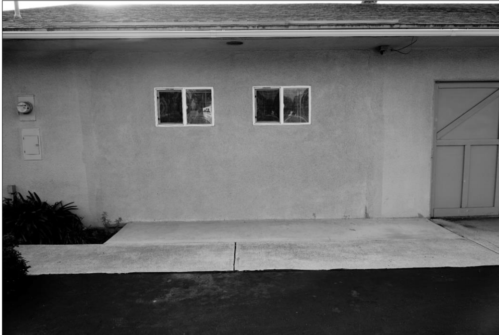
Photo 3: Area of Possible Remodel Adjacent to Garage Doors. View South-Southeast. DSC7151
