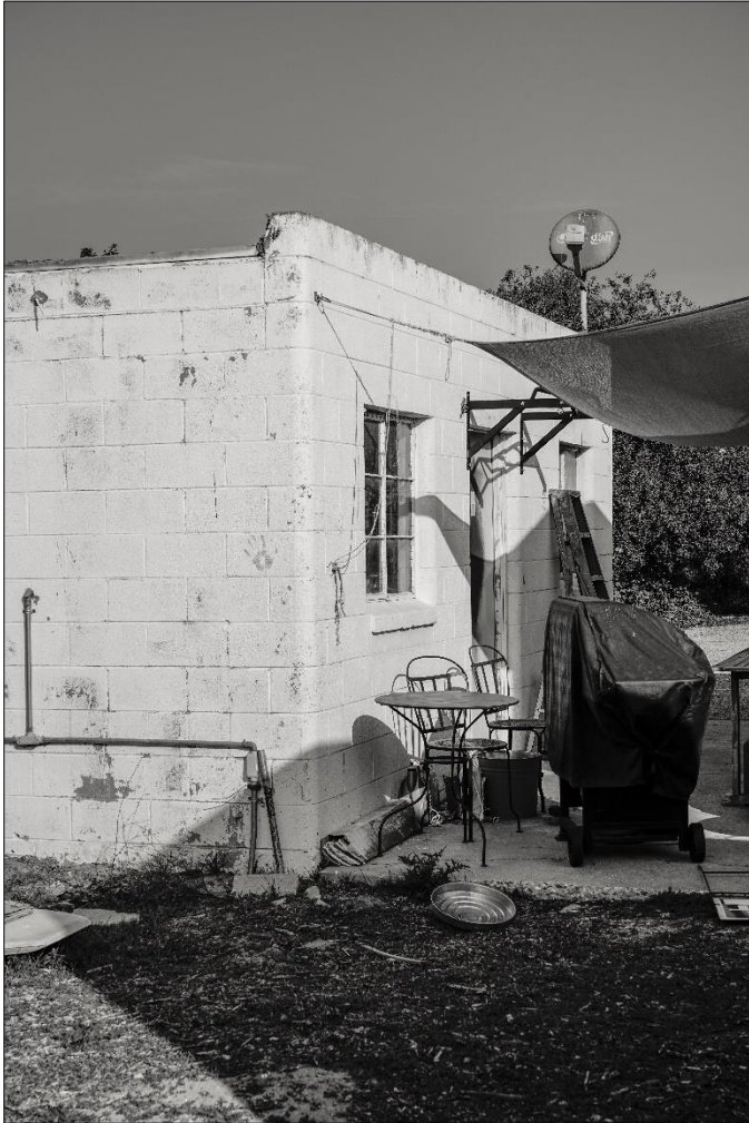
Photo 5: 3/4 view of View of Southeast Corner of Garage. View North-Northwest. DSC7192
