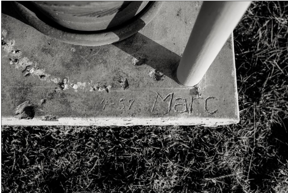
Photo 12: Date Stamp in Slab of Southeast Patio. DSC7132
