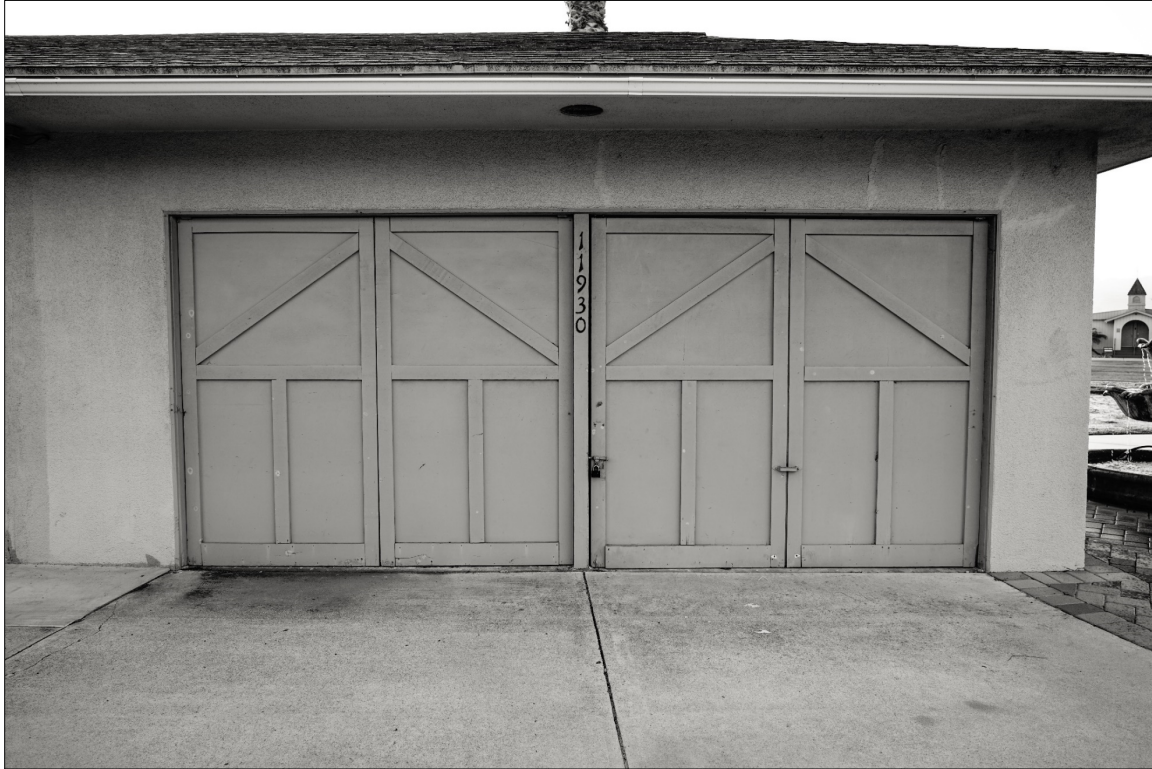
Photo 3: Replacement Garage Doors in Original Framing. View South-Southeast
