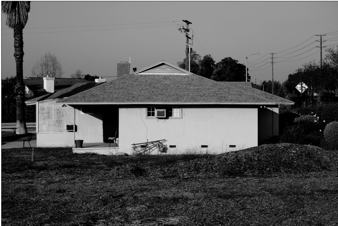
Photo 12: East Elevation. Note Enclosure of Patio Porch no longer Mimics Feeling of Southeast Patio. View West
