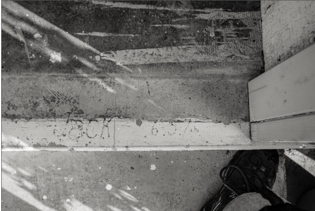
Photo 13: Date Stamp in Rear Patio Porch Slab. Note Removed Stem Wall Ghost Print in Modified Entryway. DSC7125
