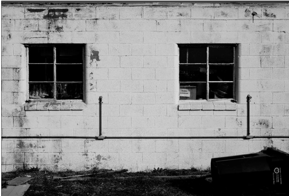
Photo 4: Detail of Window Sets in South Wall. View North. DSC7191
