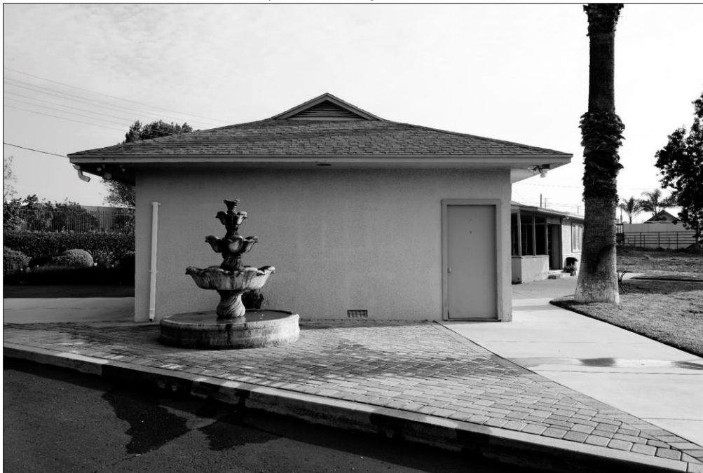
Photo 4: West Elevation, with Replacement Door, Jams, and Casing. View East-Northeast. DSC7149
