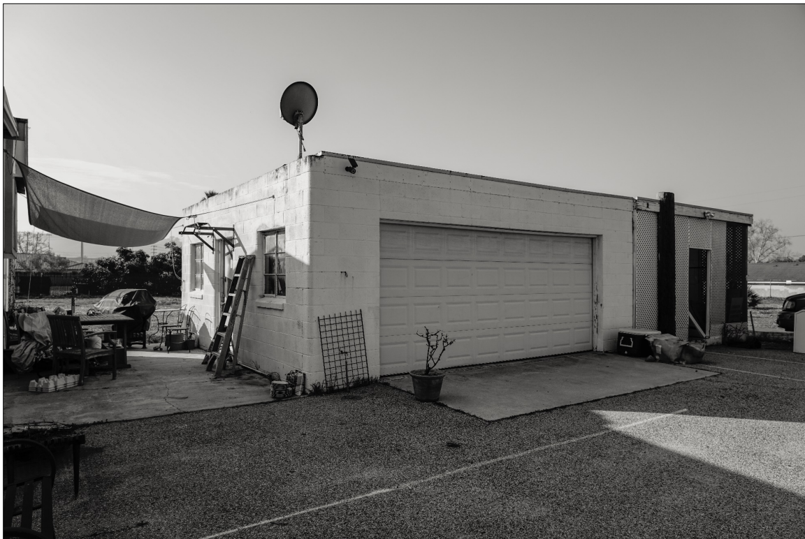
Photo 17: 3/4 View of Garage. View Southwest
