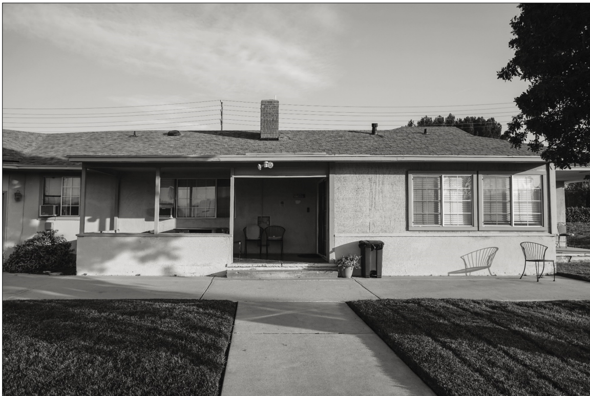
Photo 8: Partially Enclosed Patio Porch with Modified Entryway. View North
