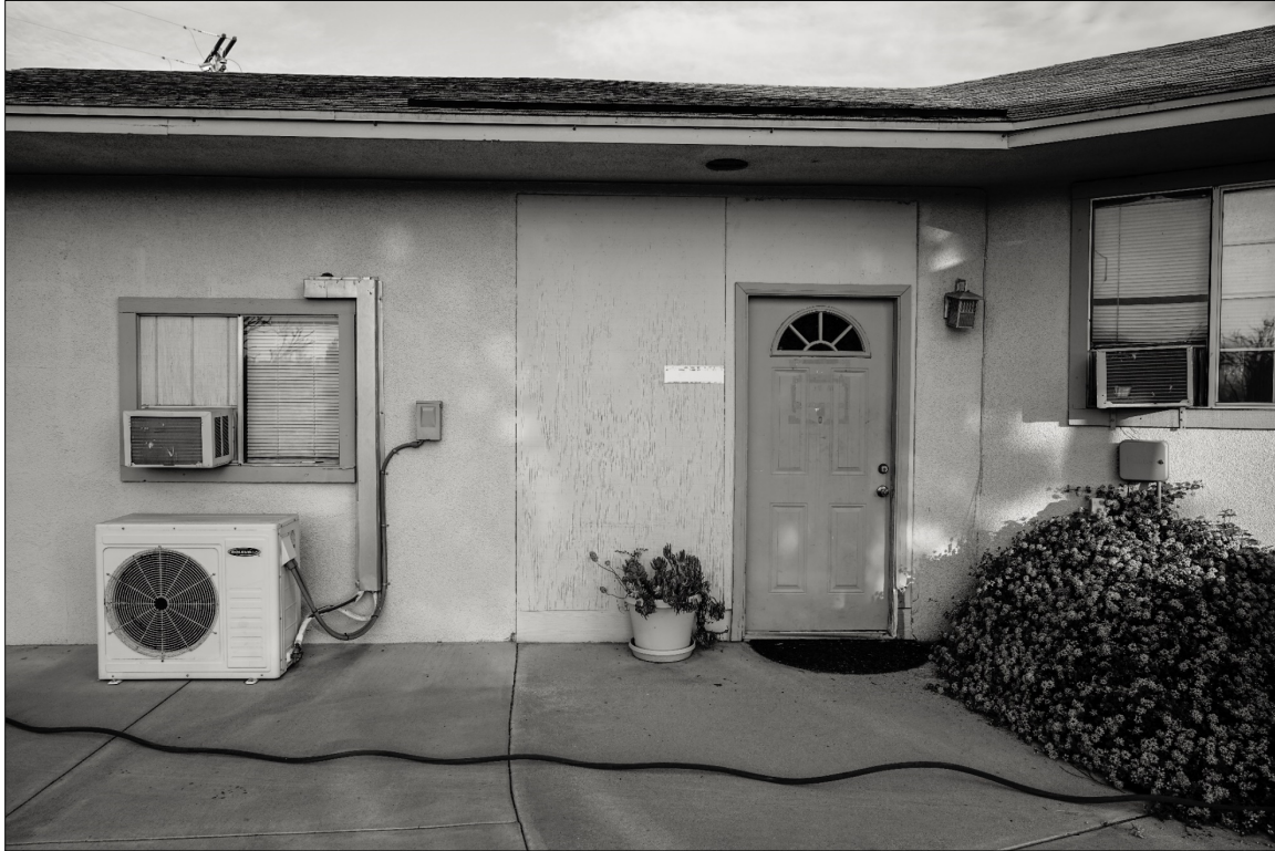
Photo 7: Low-cost Incompatible Infilling of Prior Aperture Between Main House (R) and Garage (L). View North
