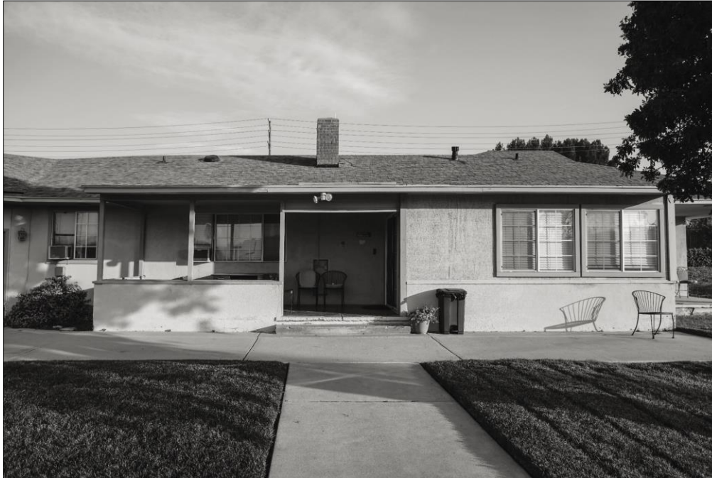
Photo 7: Partially Enclosed Patio with Modified Entryway. View North. DSC7123
