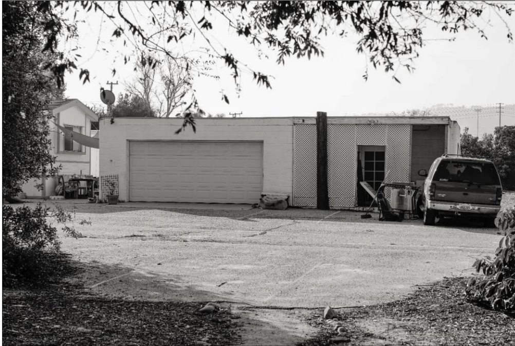
Photo 1: 11932 Los Angeles Avenue, 1952 Menashe Ranch Garage North Profile. View South. DSC7176
