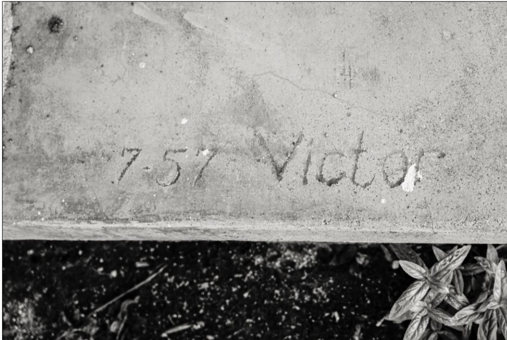
Photo 14: Date Stamp in Front Porch Slab. DSC7104
