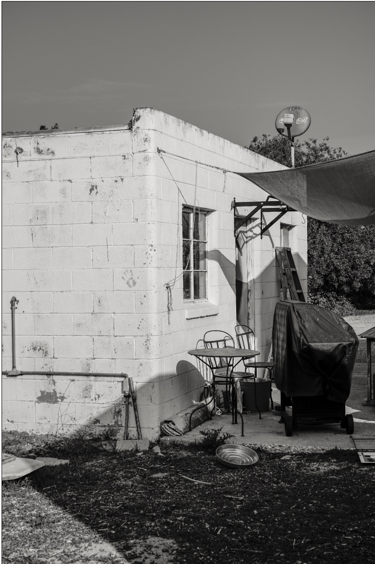
Photo 20: 3/4 View of Southeast Corner of Garage. View North-Northwest
