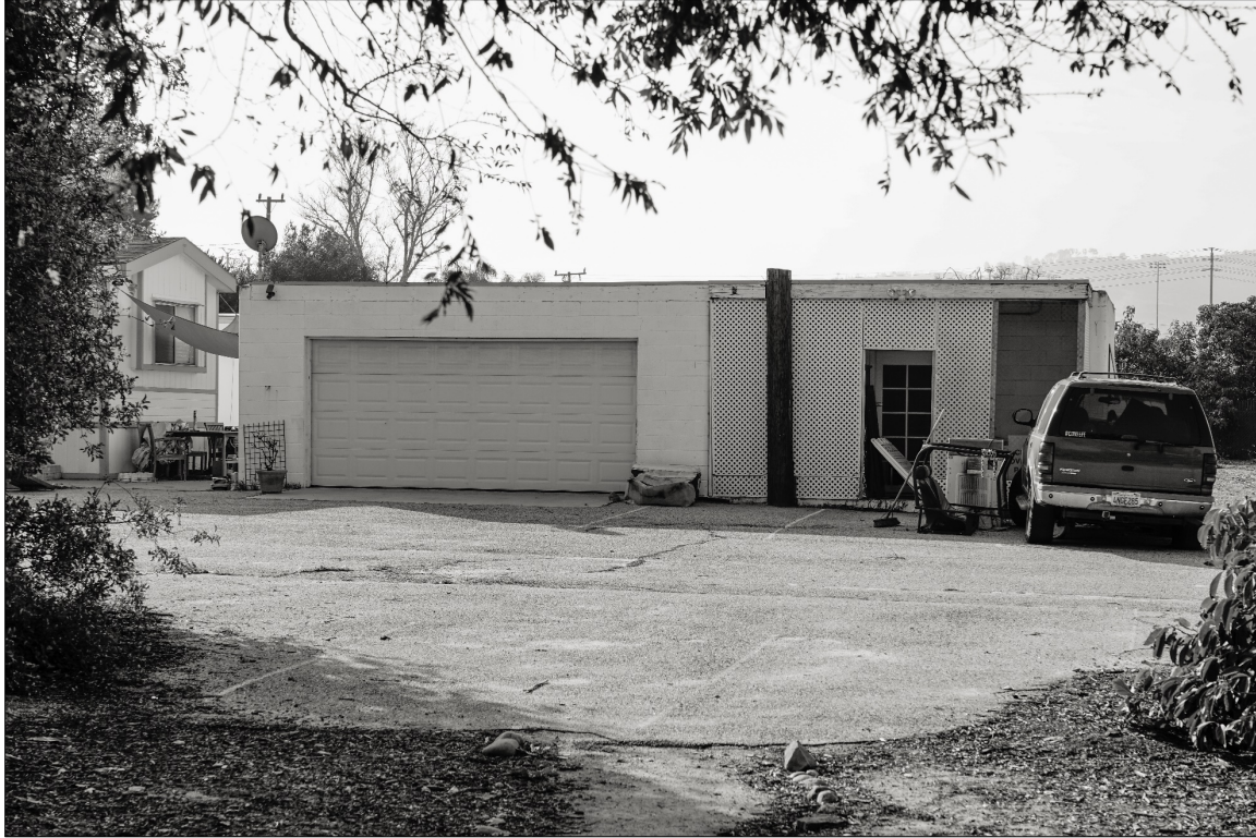
Photo 16: 11932 Los Angeles Avenue Garage. View South-Southeast
