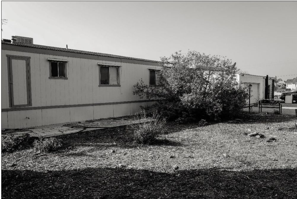
Photo 8: Oblique View of Mobile Home on Original Concrete Slab, and Garage, Illustrating Relative Setting. View West-Southwest. DSC7200
