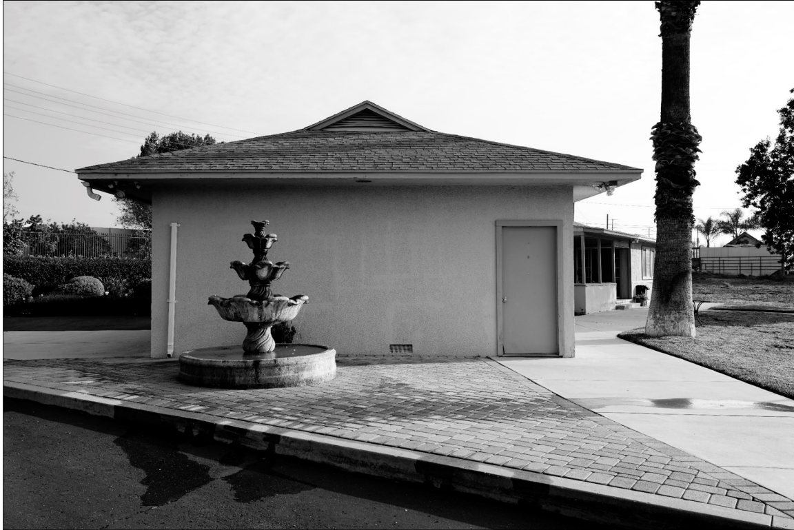
Photo 5: West Elevation, with Replacement Door, Jams, and Casing. View East-Northeast
