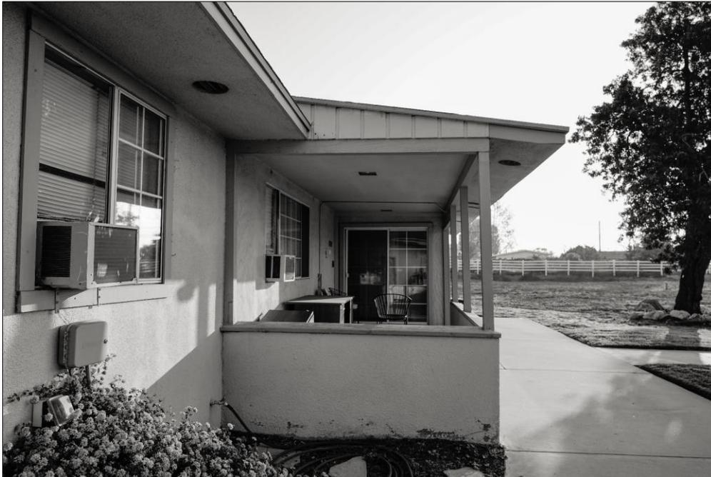
Photo 8: Rear Patio Porch with Original Finishes. Note Vertical Drop-Lap Siding below Shed Roof, and Original Framing. Note Replacement Vinyl Windows and Doors and 1"x4" Casement. Note Round Soffit Vents. View East. DSC7121
