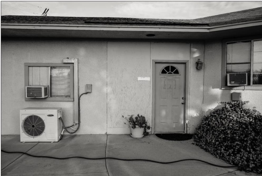
Photo 6: Low-cost Incompatible Infilling of Prior Aperture Between Main House (R) and Garage (L). View North. DSC7120
