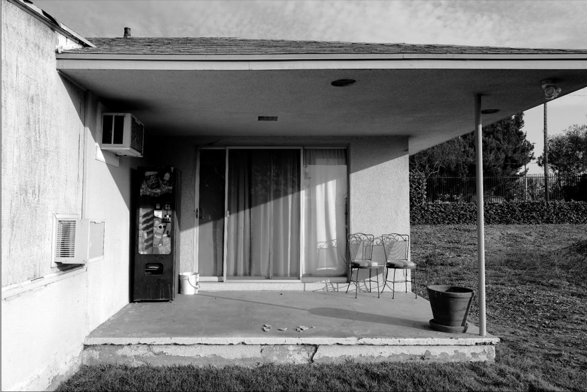
Photo 11: Patio at Southeast Corner of House with Original Aluminum Sliding Doors and Casework. Note Rough-Sawn No Bead Plywood Siding Enclosing Patio Porch and Loss of Fabric Noted in Photo 9. View North
