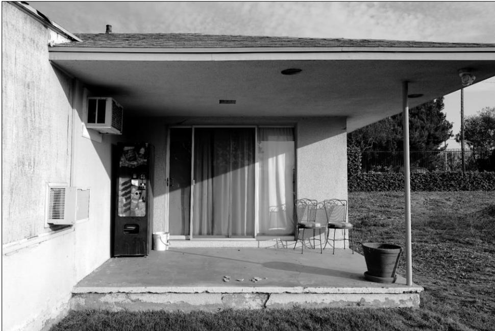
Photo 10: Patio at Southeast Corner of House with Original Aluminum Sliding Doors and Casework. Note Rough-Sawn No Bead Plywood Siding Enclosing Patio Porch and Loss of Fabric Noted in Photo 9. View North. DSC7142
