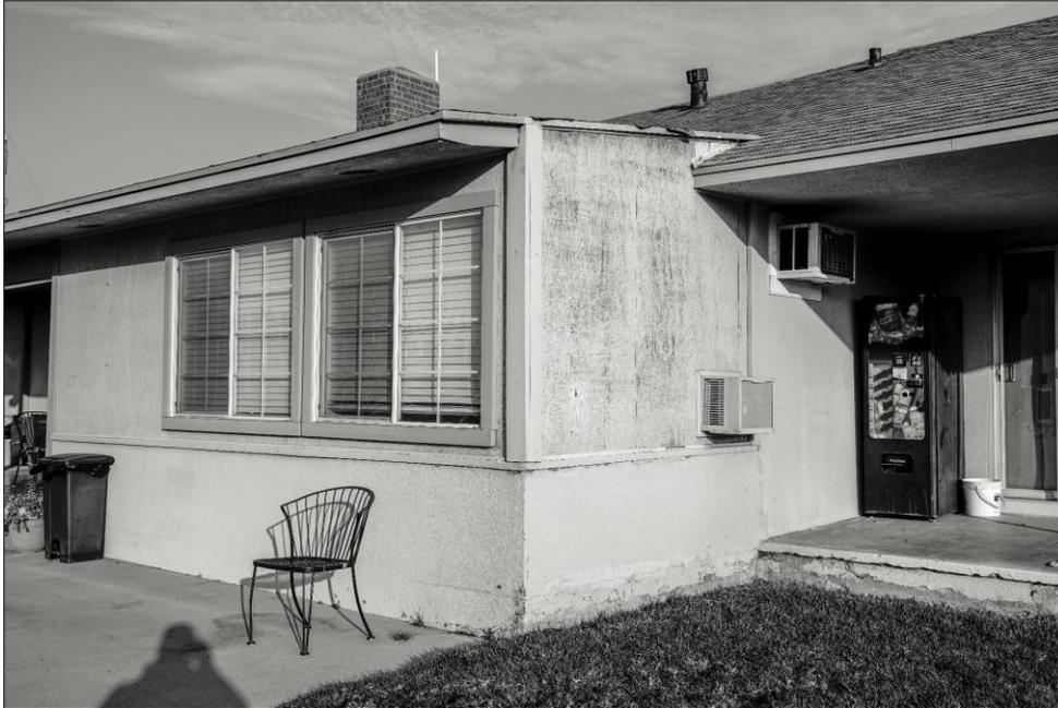
Photo 9: Enclosed Patio Porch. Note Loss of Fabric, Feeling, and Condition Noted in Photo 9. Note use of 2"x4" Studs, instead of Appropriate 1"x4" Common Board for Casing View Northwest. DSC7130
