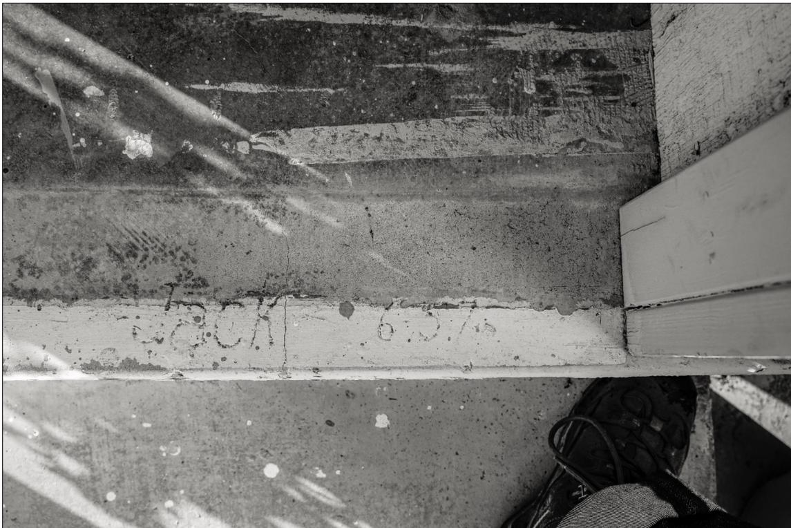
Photo 14: Date Stamp in Rear Patio Porch Slab. Note Removed Stem Wall Ghost Print in Modified Entryway
