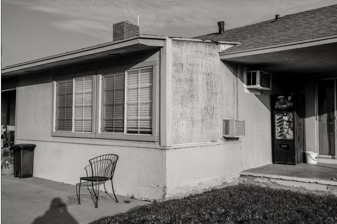
Photo 10: Enclosed Patio Porch. Note Loss of Fabric, Feeling, and Condition Noted in Photo 9. Note use of 2"x4" Studs, instead of Appropriate 1"x4" Common Board for Casing View Northwest
