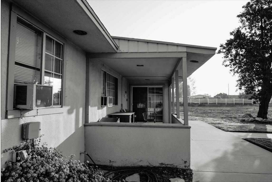
Photo 9: Rear Patio Porch with Original Finishes. Note Vertical Drop-Lap Siding below Shed Roof, and Original Framing. Note Replacement Vinyl Windows and Doors and 1"x4" Casement. Note Round Soffit Vents. View East
