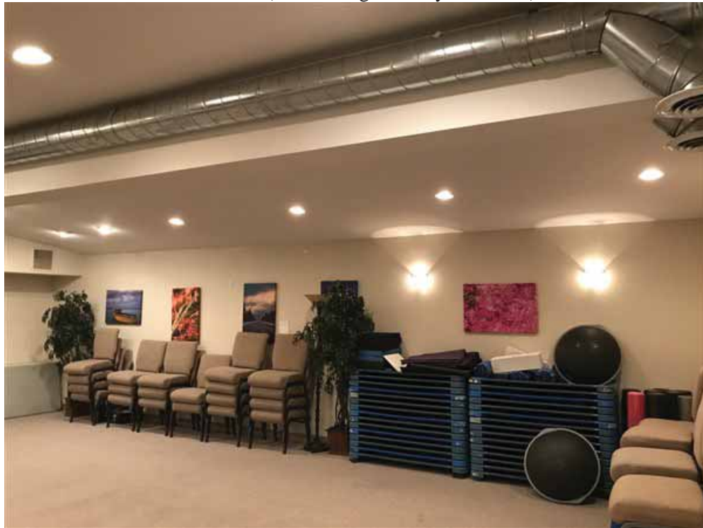
Photo 10: Typical view inside the modular-church-facility building Unit C.
