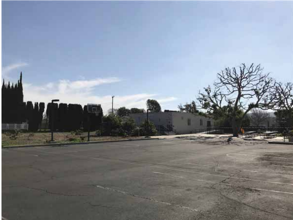
Photo 5: Southeastern-facing view of the asphalt-paved parking lot and (Unit A) one of three modular-church-facility buildings located within the central part of the subject site (background).
