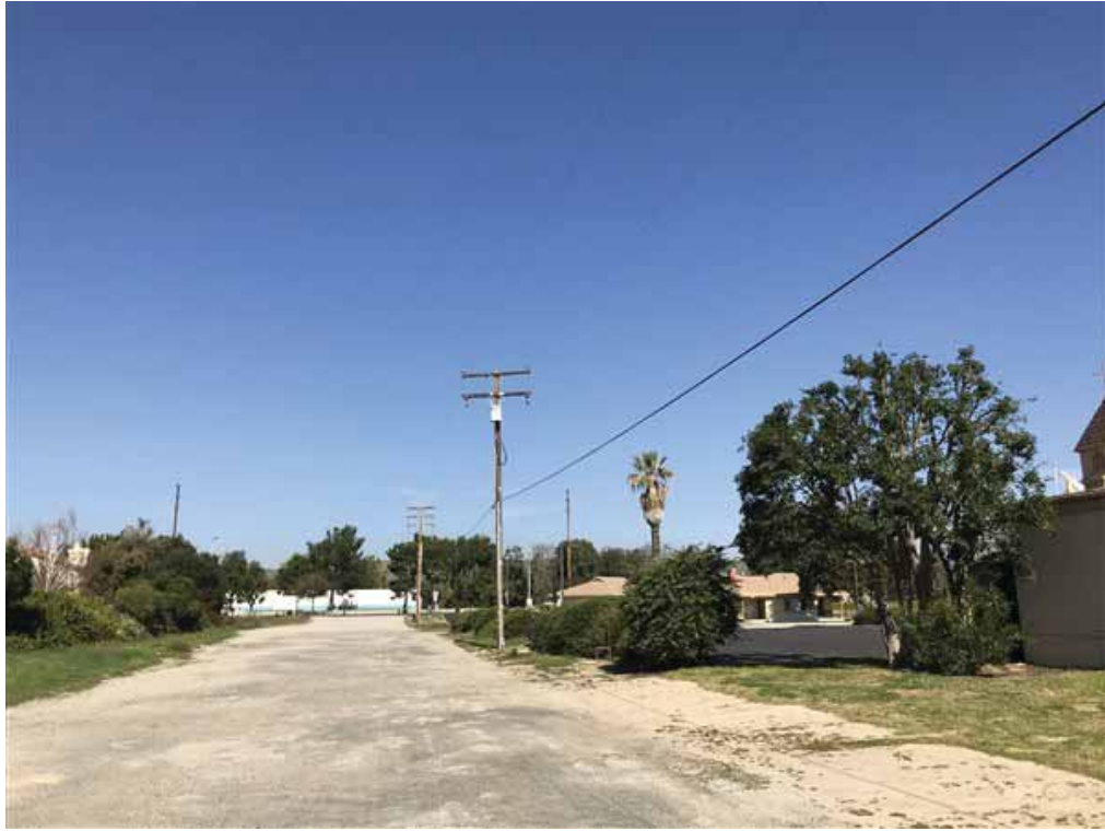
Photo 19: Northern-facing view along the northern portion of Beltramo Road; one of three pole-mounted transformers located at the subject site is also pictured.
