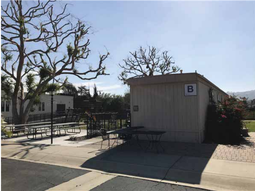
Photo 7: Southern-facing view of Unit B, one of three modular-church-facility buildings located within the central part of the subject site.
