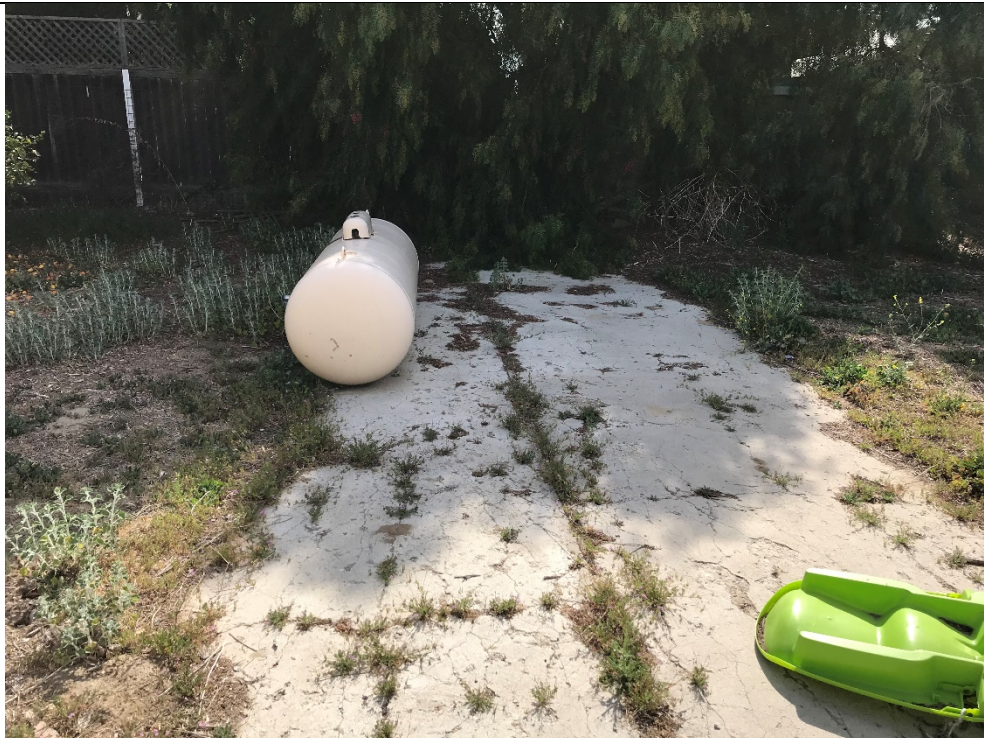
Photo #6 View of a propane aboveground storage tank near the southern church residence.
