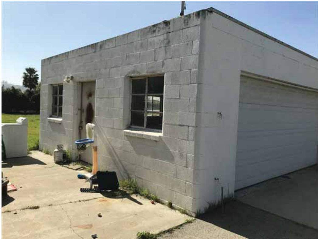
Photo 15: Close-up view of a slab-on-grade dwelling and garage within Parcel 4.
