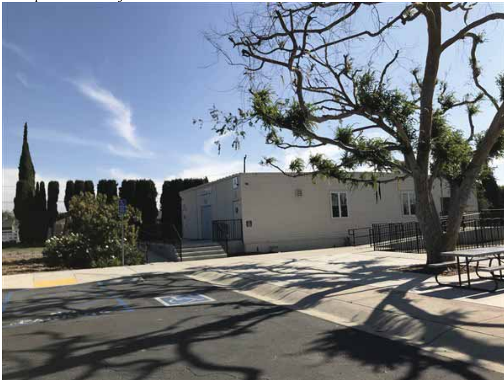
Photo 8: Eastern-facing view of Unit A, one of three modular-church-facility buildings located within the central part of the subject site (background).
