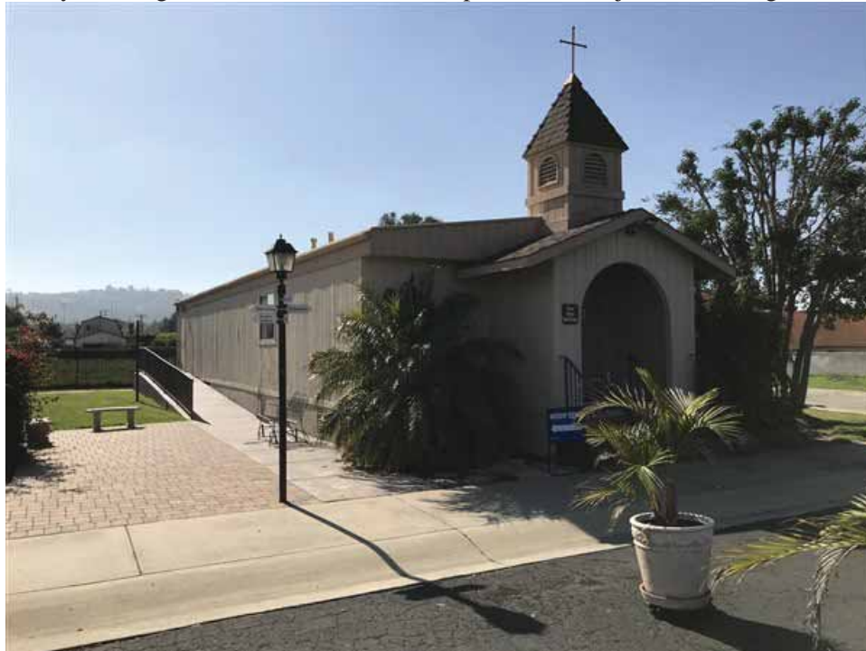
Photo 6: Southern-facing view of Unit C, one of three modular-church-facility buildings located within the central part of the subject site.
