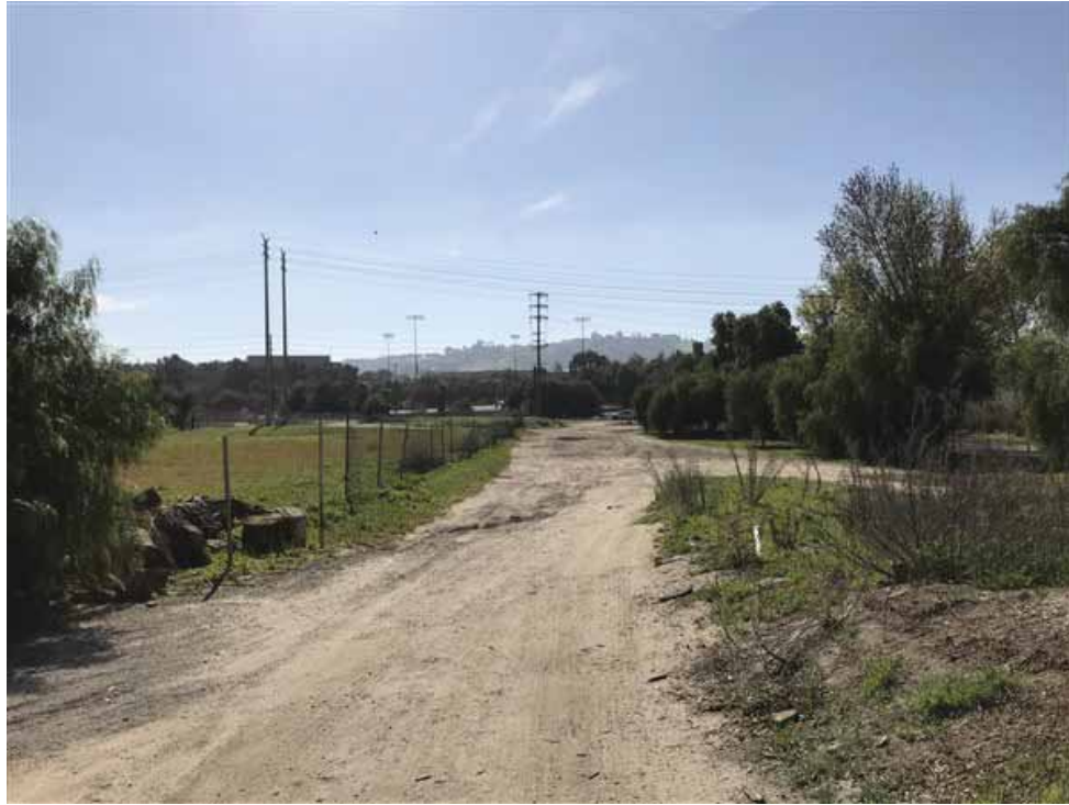
Photo 25: Southern-facing view along the unpaved southern portion of Beltramo Road; one of three pole-mounted transformers is also pictured.
