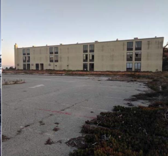
Photo 2: Project site looking north from existing parking lot.
