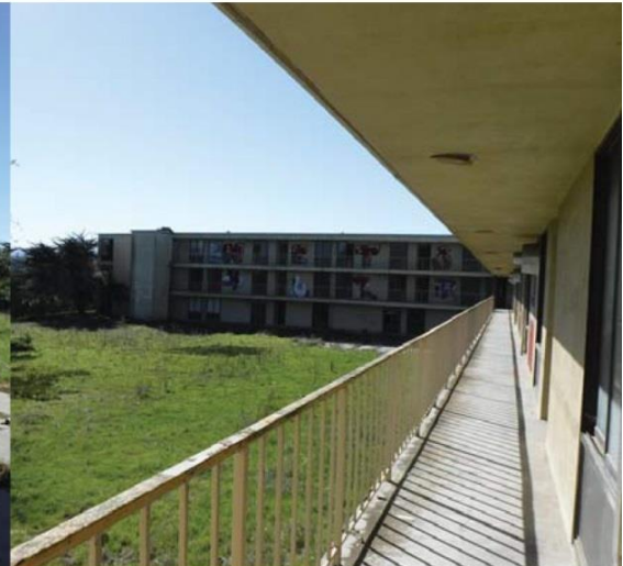
Photo 6: Project site looking south from second story on north end of Building B.
