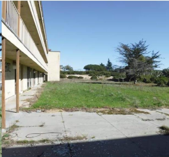
Photo 5: Project site looking northeast from patio area between the building footprints.
