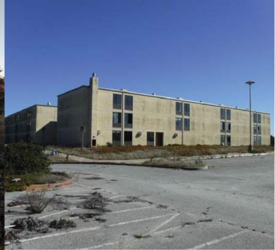
Photo 3: Project site looking northeast from existing parking lot.
