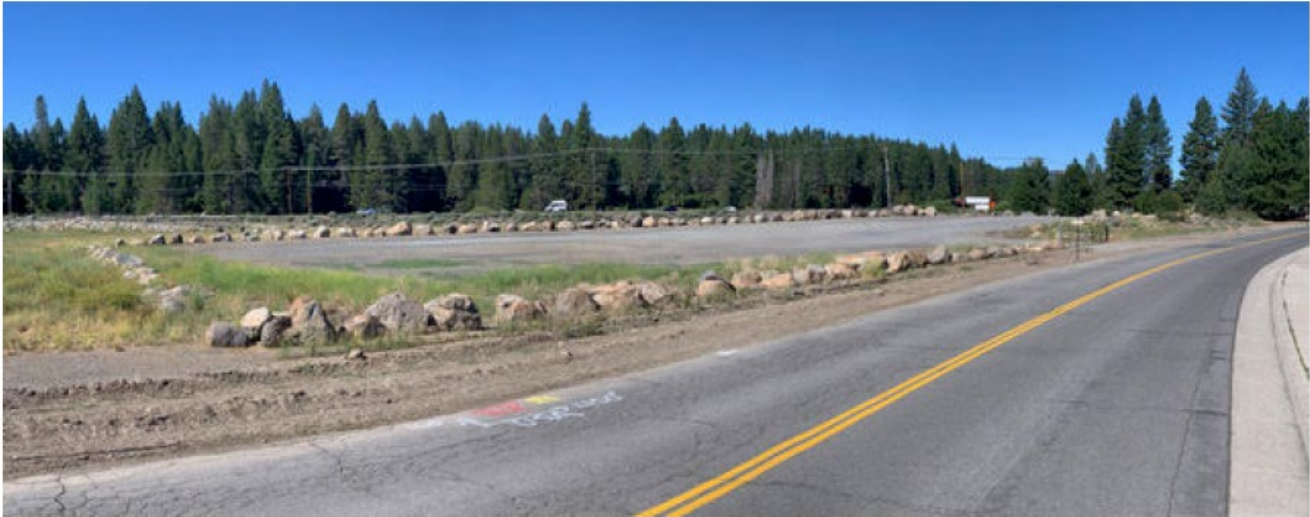
Project overview (view southwest); Estates Drive (foreground)
