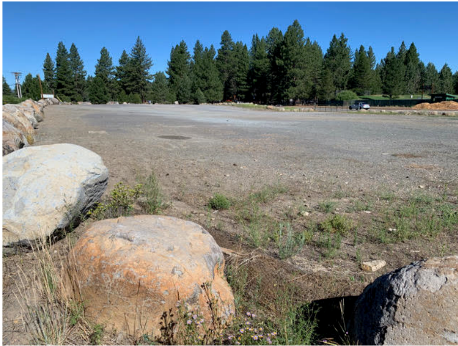
Photo 3. Project overview (view northwest)
