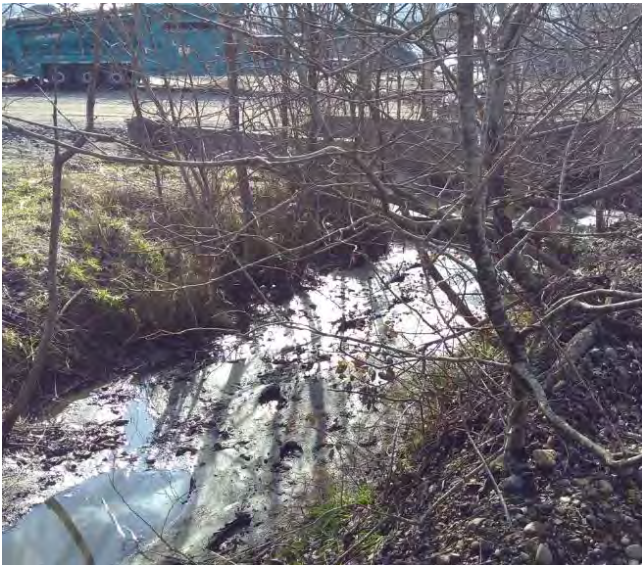
Photo B17: TP17U Site looking east. Note check dam structure and existing industrial use. Sediment is removed annually.
