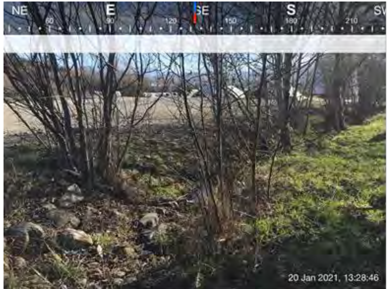
Photo 2. Stormwater overflow conveyance feature in center of facility.
