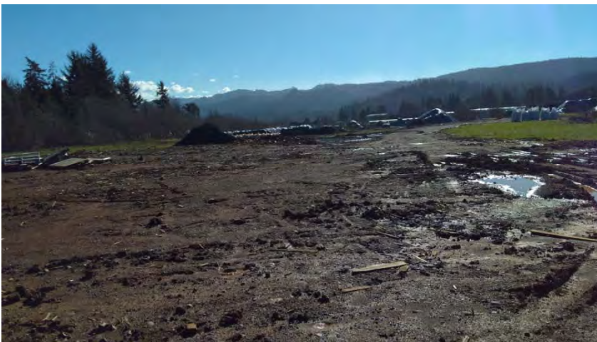
Photo 3. Looking east across the project area. Note Soil piles and lack of vegetation in foreground. Photo taken January 24, 2017.
