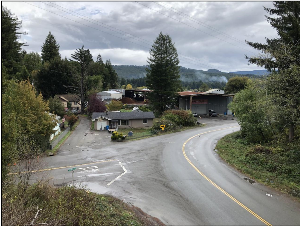
Figure 7: View of southwest edge of Royal Gold site from Highway 299 Overpass
