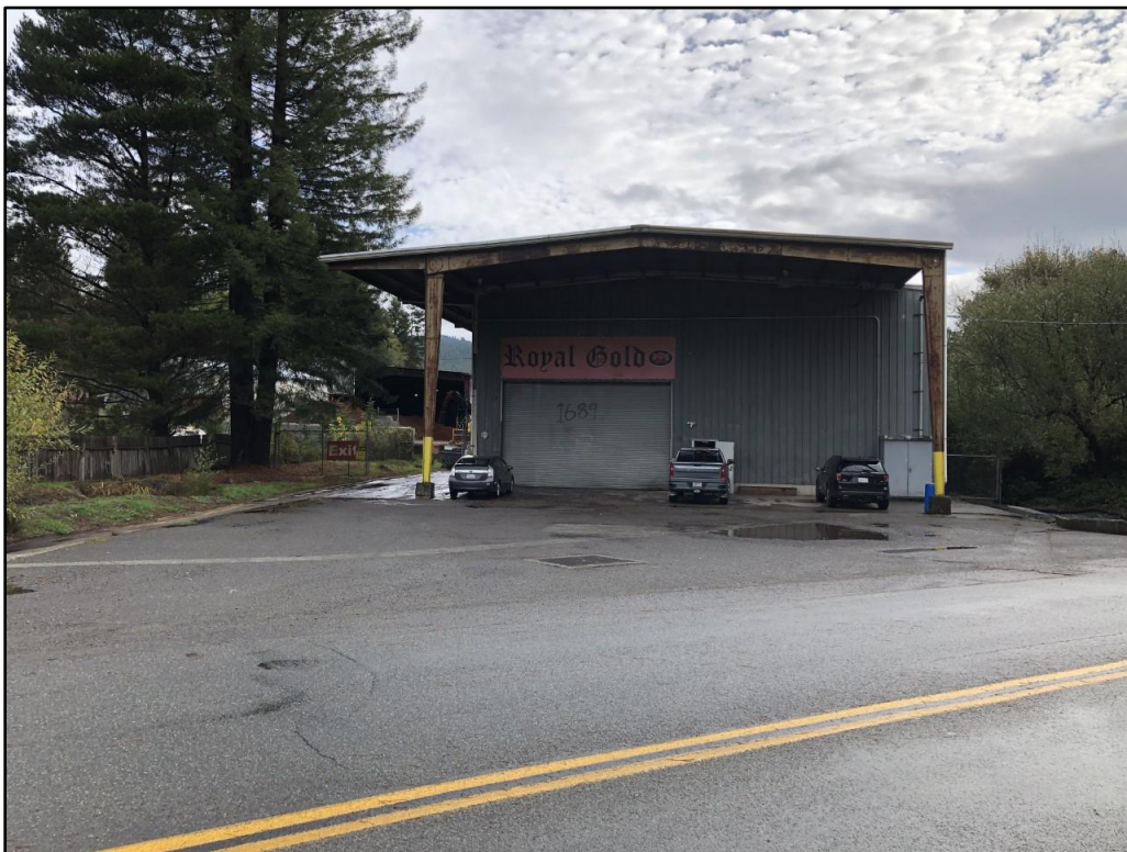
Figure 8: View of southwest exit at Royal Gold site from Glendale Drive
