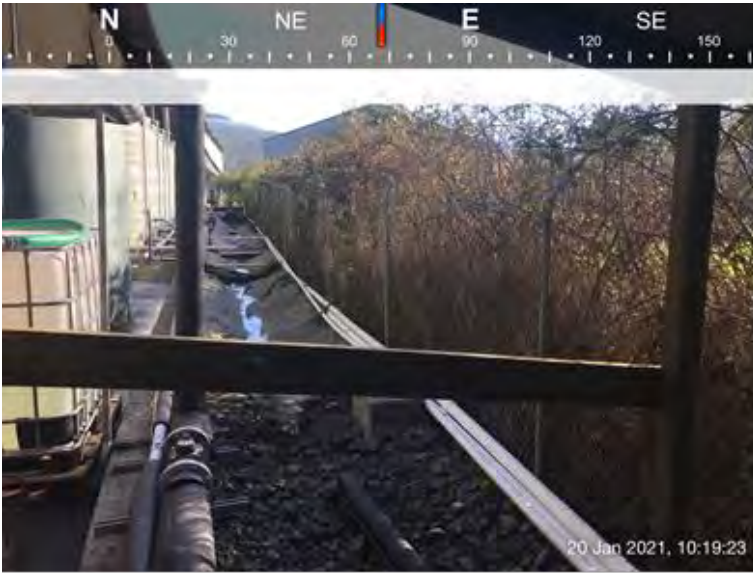
Photo 5. Stormwater conveyance channel along SW boundary.
