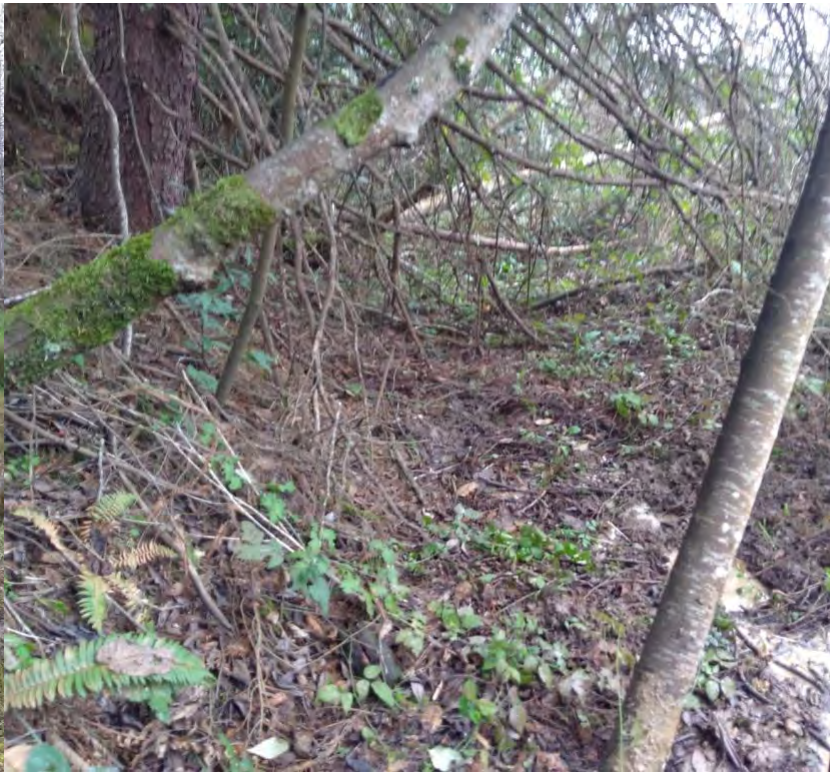
Photo B26: TP21U in old constructed drainageway on the east side of the project.
