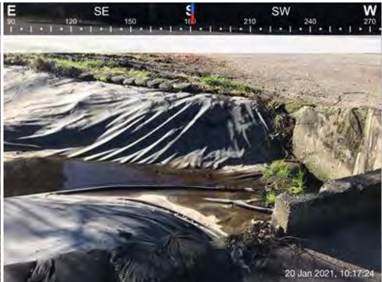
Photo 4. Stormwater conveyance feature in SW corner of facility.
