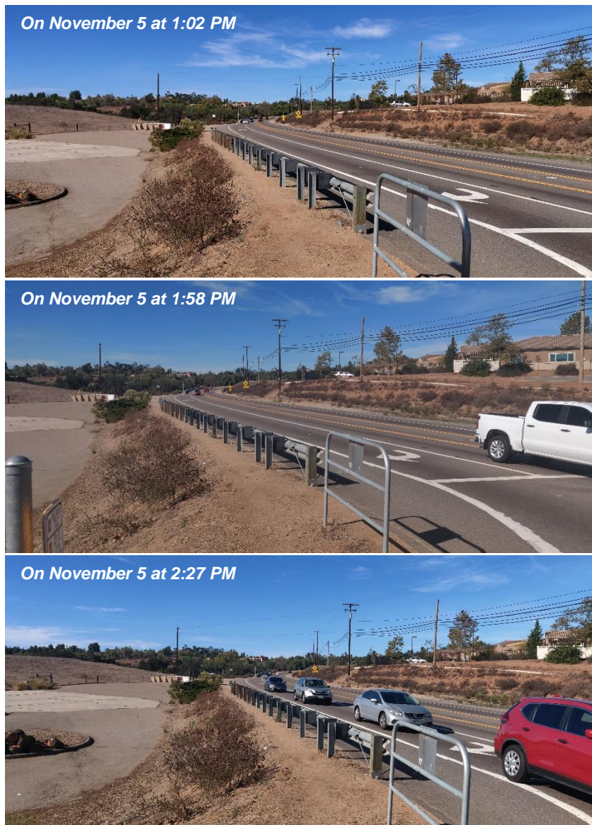
Figure 1: Southbound SR-94 at Daisy Drive
