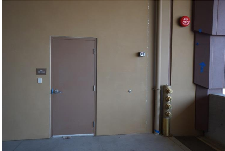
Door to Fire Command Center, at the north parking entrance on floor P8, showing the adjacent Lock box and Fire Department Connection.
