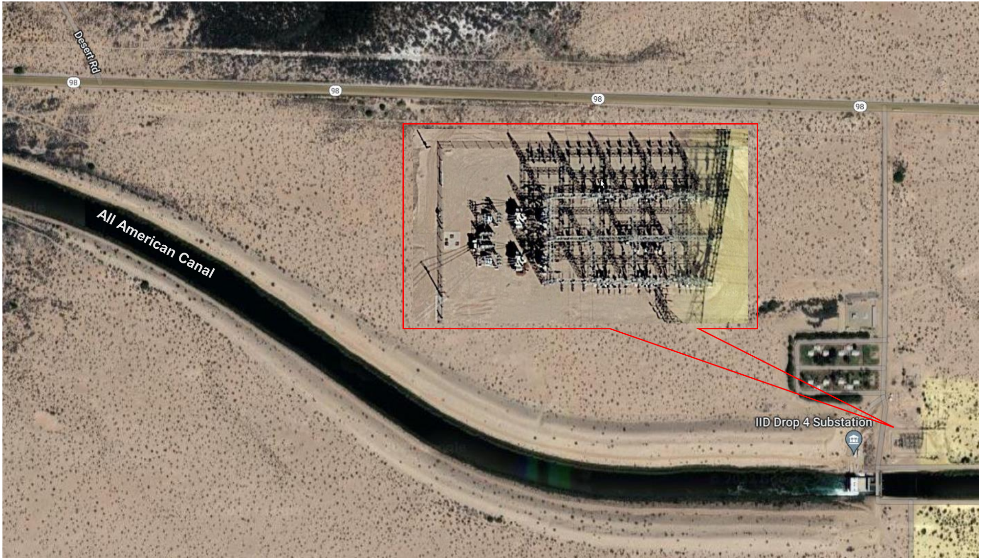
ECSS 92kV Bus Transmission Relay Project (No. 30037966) IID Drop 4 Hydro Plant Substation (1/8 th of mile south of Hwy. 98, 3 miles west of I-8 Junction, along the All-American Canal, east of Holtville, CA) Location Map
