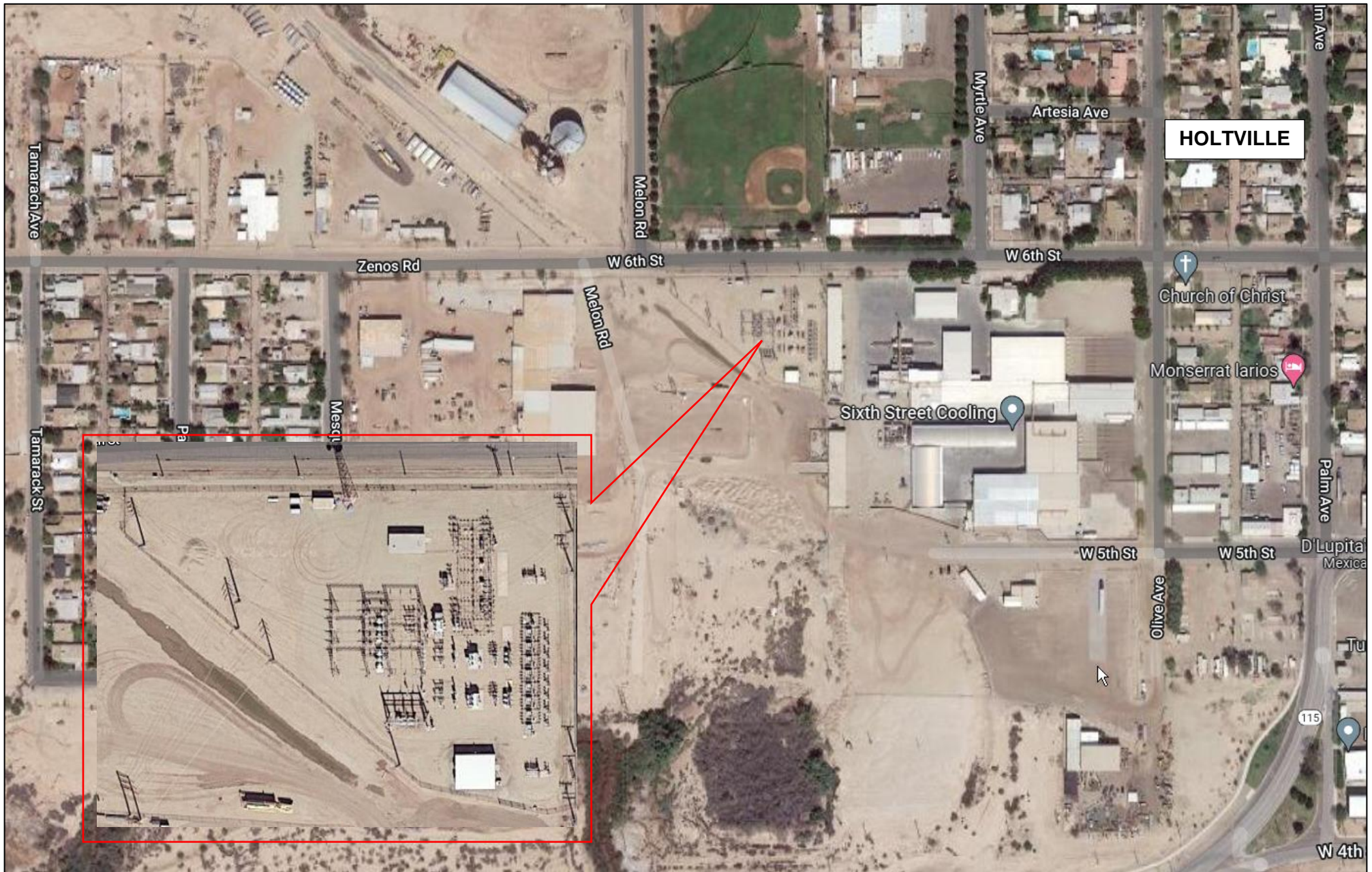
ECSS 92kV Bus Transmission Relay Project (No. 30037966) IID Holtville Substation Location Map
