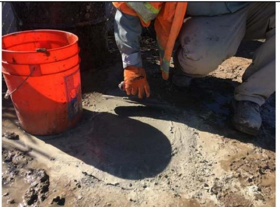
Photo 8. View of abandoned well finished off with cement.
