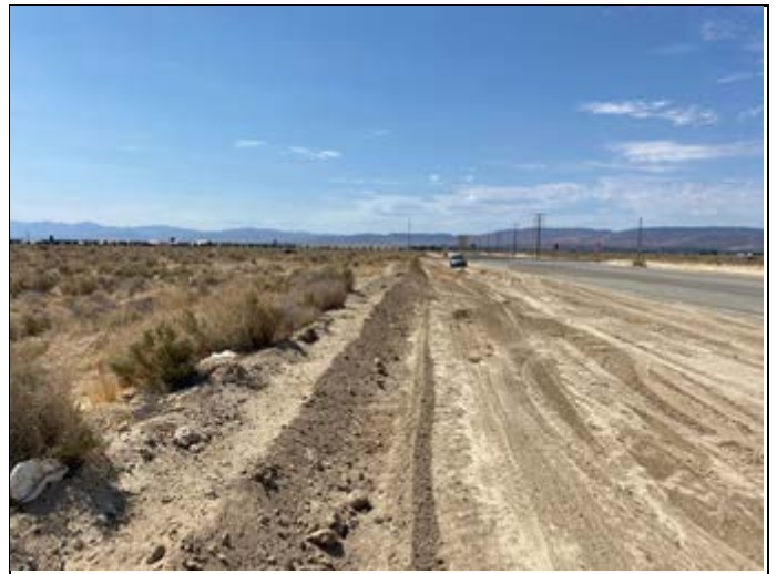
10. View south along western subject property boundary
