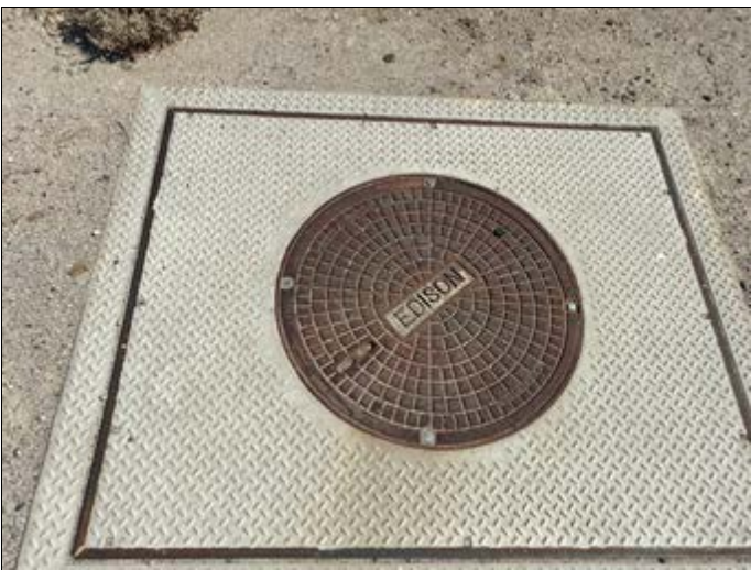
23. View of utility manhole cover near southern boundary of subject property
