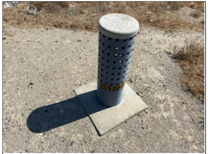
22. View of utility post near southern boundary of property
