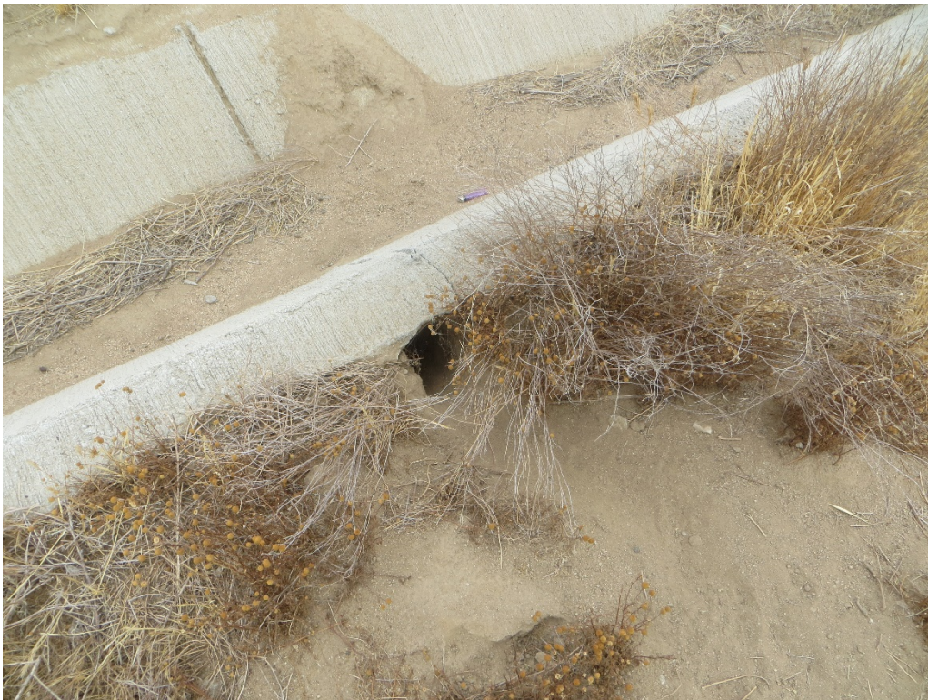
Photograph 10: A suitable burrow beneath a concrete v-ditch along the western boundary of the project site.
