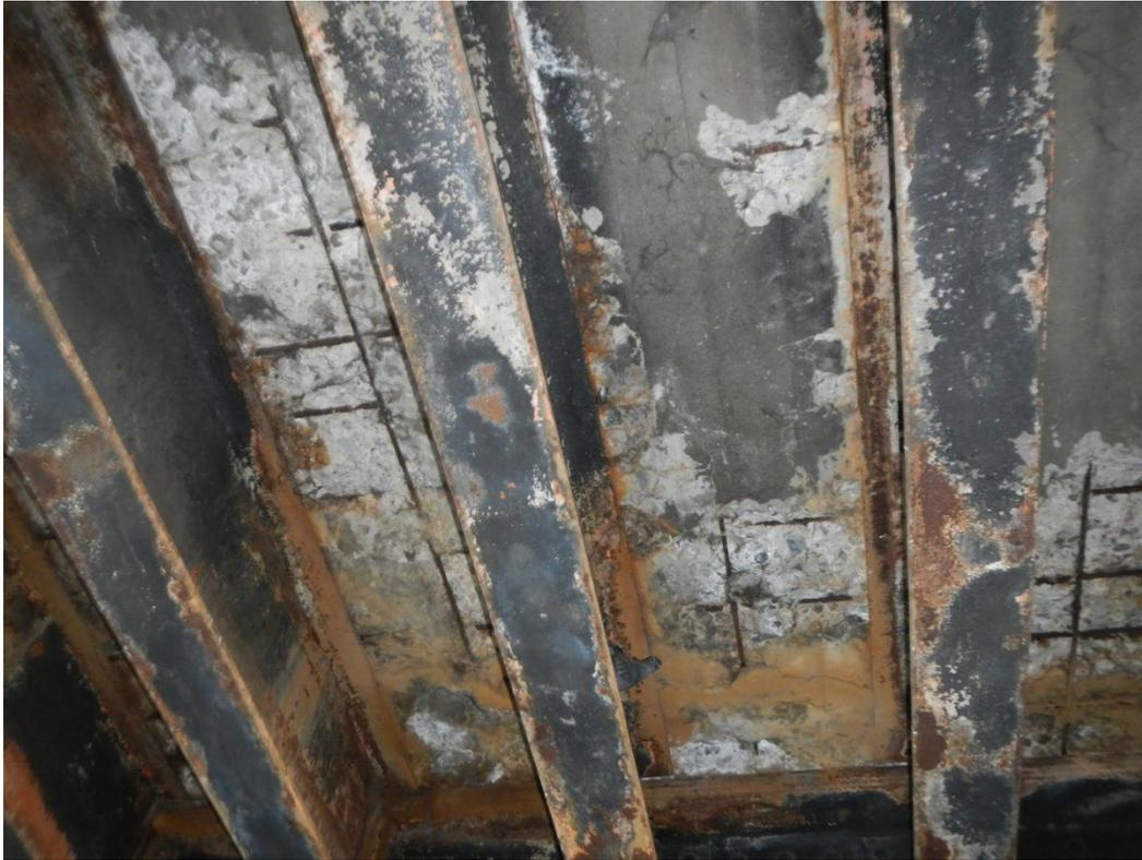
Figure 4. Cracked Steel Stringer at Flange Cope
