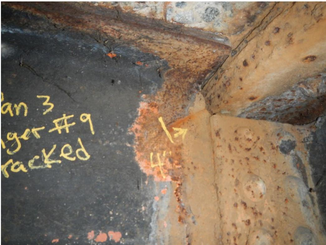
**Figure 5. Span 2 Pier 2 Expansion Bearing with Missing Retainer Plate and 1 of 4 Anchor Bolts Remaining**
