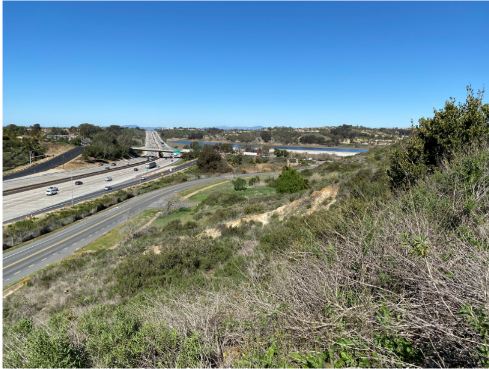
Photograph #9 View to the northeast across the northern portion of the Site.
