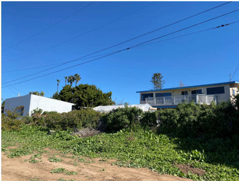
Photograph #18 Residential homes adjacent to the east of the Site.
