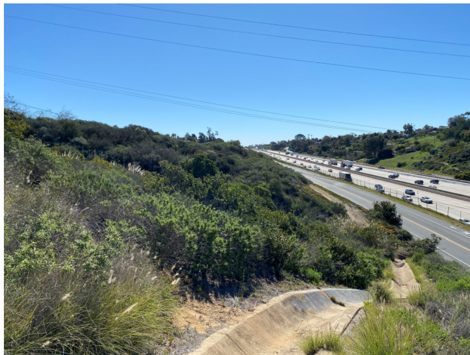
Photograph #14 Concrete brow ditch along the western boundary of the Site.
