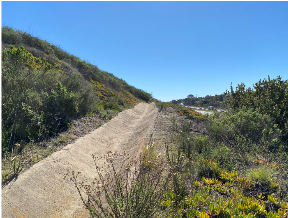
Photograph #13 Concrete brow ditch along the western boundary of the Site.
