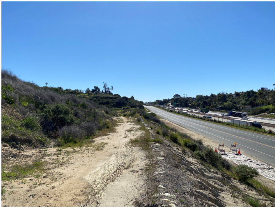
Photograph #8 View to the south along the western boundary of the Site.
