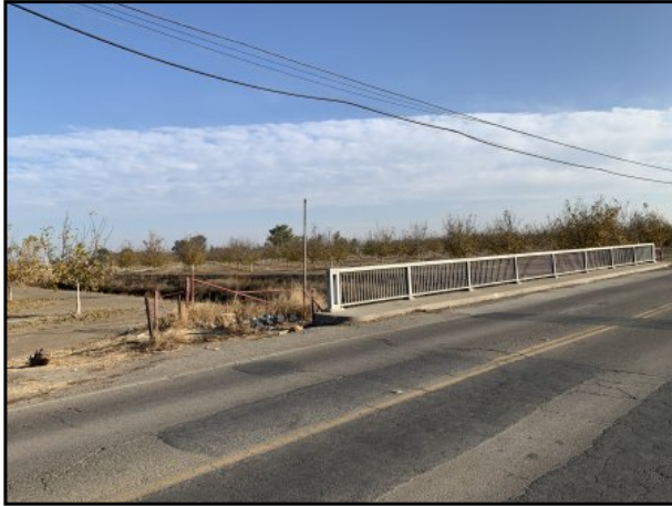
1 : View looking southeast showing bridge over drainage ditch.
