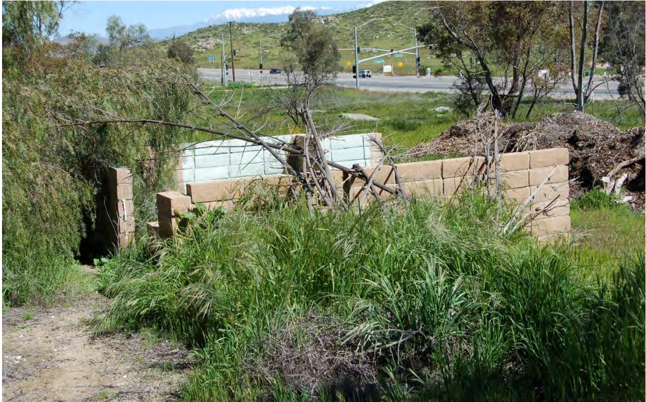
Remnants of an old structure located on the southwest side of the site
