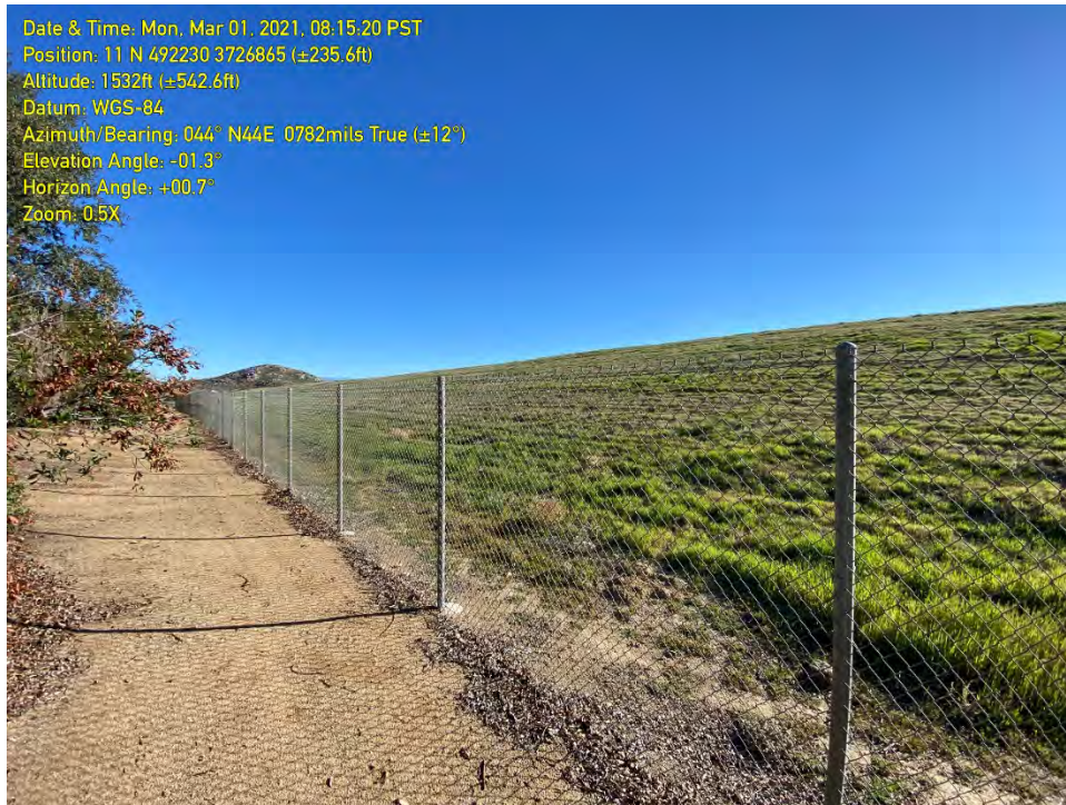
PHOTOGRAPH 7: A view of the moderate-quality BUOW habitat east of Hwy 79. The manufactured slope was sloped towards planted native trees and shrubs along Hwy 79, thus reducing the overall habitat suitability for BUOW.
