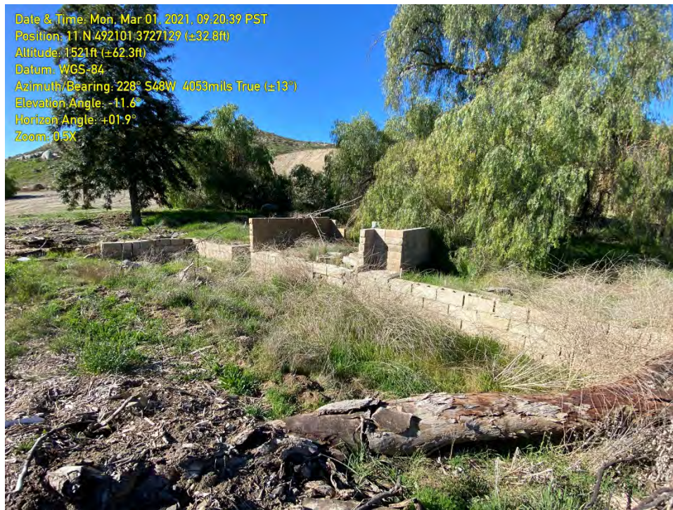
PHOTOGRAPH 3: Partial foundation remaining from a former structure in the central-portion of the Site.
