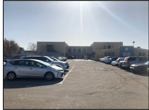
6 : View of the exterior of the site, facing south.
