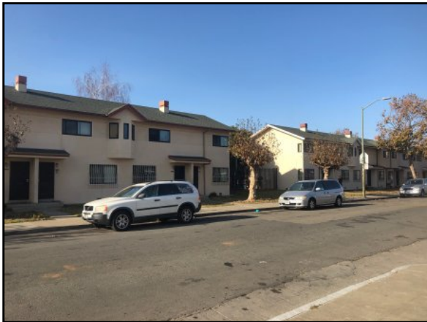
11 : View of the property adjacent to the west of the site.
