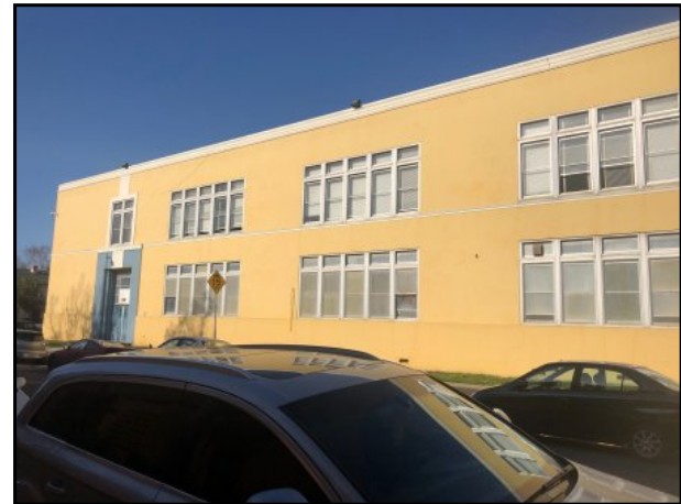
8 : View of the southern exterior of the building.
