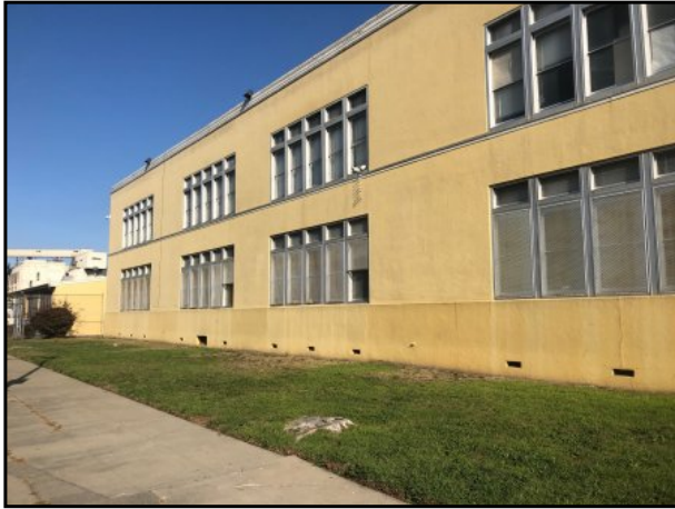
9 : View of the western exterior of the building.
