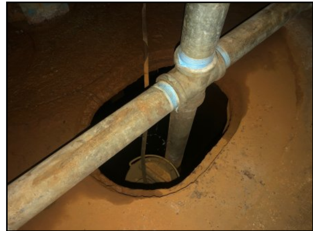
28 : View of the sump in the boiler room.
