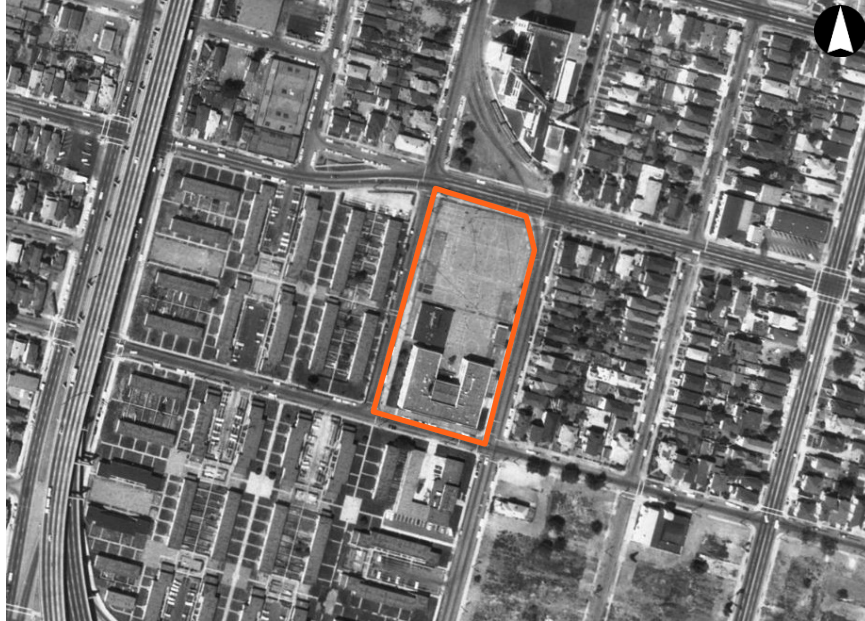
Figure 79: Aerial photograph of subject property and vicinity, 1965. Source: UC Santa Barbara Library Special Collections, Cartwright Aerial Surveys, Flight CAS_65_130, Frame 15-117.
