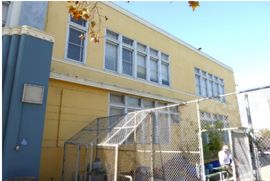
Figure 12: Three westernmost bays at the primary façade, looking northwest.
