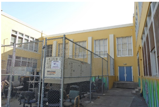
Figure 25: Center, recessed portion of rear façade at auditorium/gymnasium, looking south.
