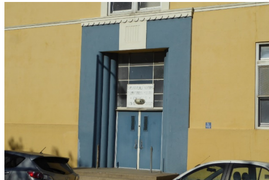
Figure 18: West entrance at south façade, looking north.
