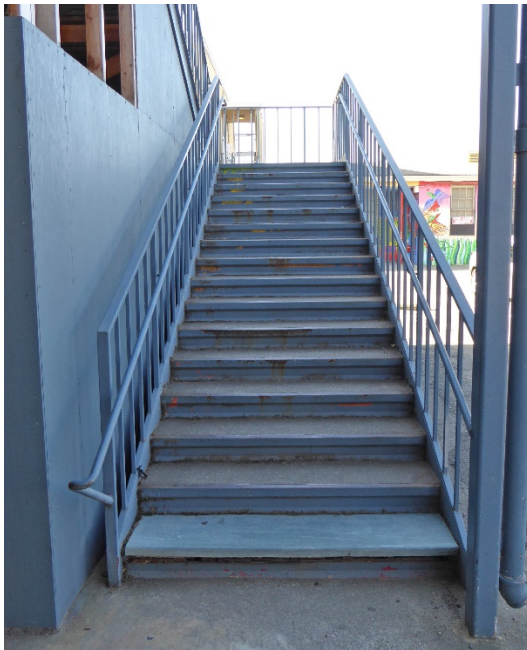
Figure 21: Looking west at steel-frame staircase at rear of the east wing.
