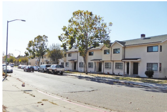
Figure 54: Looking southwest along Poplar Street toward vernacular housing typologies within the Peralta Villa Public Housing Community located west and southwest of the subject property.
