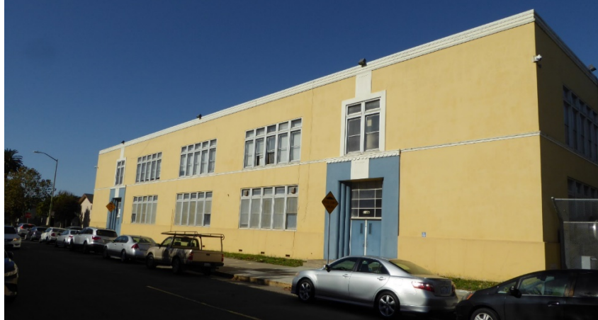
Figure 16: South façade, view southwest.
