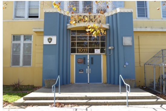
Figure 9: Primary entrance, looking west.
