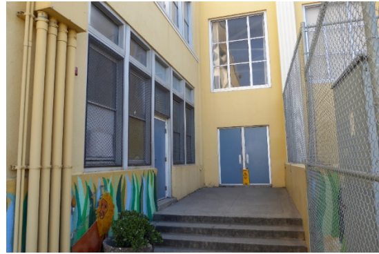
Figure 24: Entrances and windows at rear façade.
