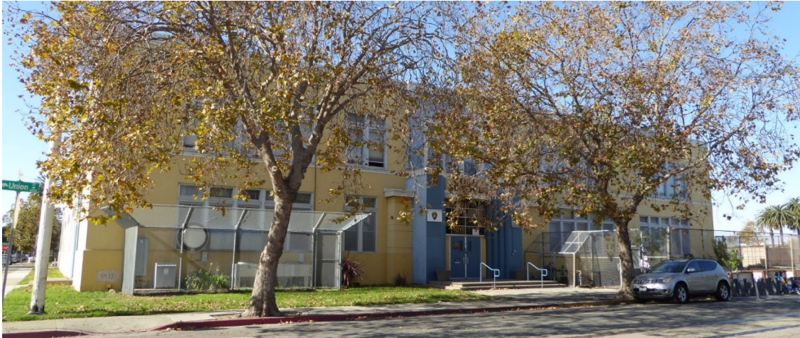
Figure 7: Cole School, looking northwest from Union Street.
