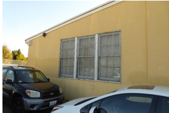
Figure 31: Three standard sash windows divided by wood mullions at the north façade, looking southeast.
