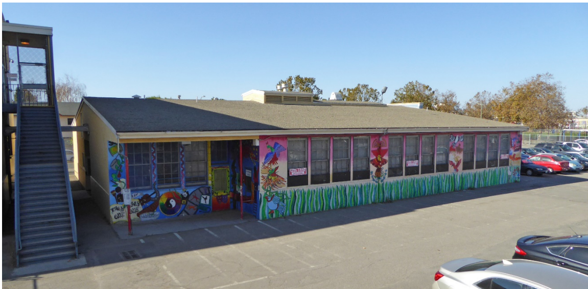
Figure 29: Cafeteria Building viewed from second story of Cole School, looking northwest.
