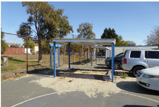
Figure 46: Structures at rear of site near north perimeter, looking east.
