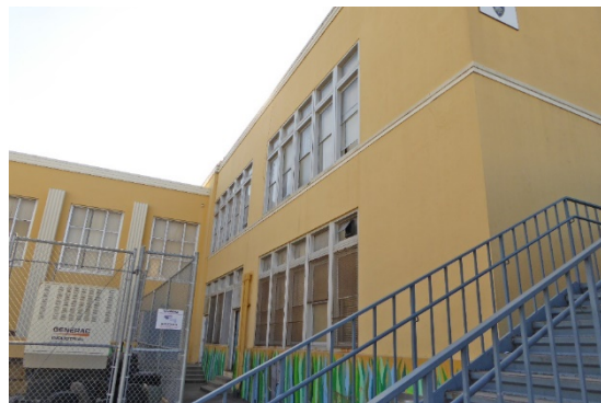
Figure 26: East-facing windows along northwest wing of the rear façade, looking south.
