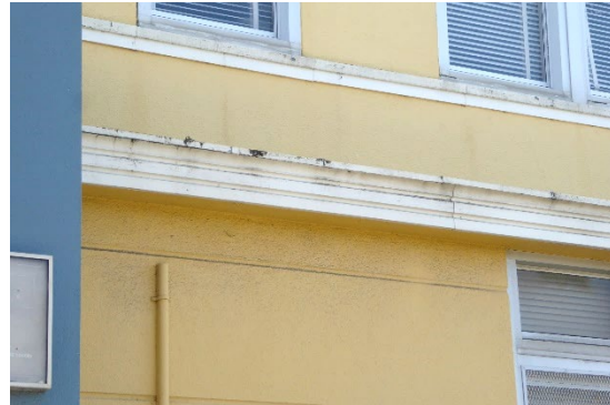
Figure 13: Molded sheet metal fascia extending northward from the main entrance above the second to northernmost bay of the primary façade.
