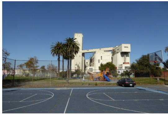
Figure 45: View looking north at north perimeter of the site from basketball court.
