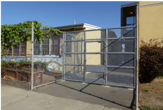
Figure 44: Security fence with gate along west perimeter of property, looking east.
