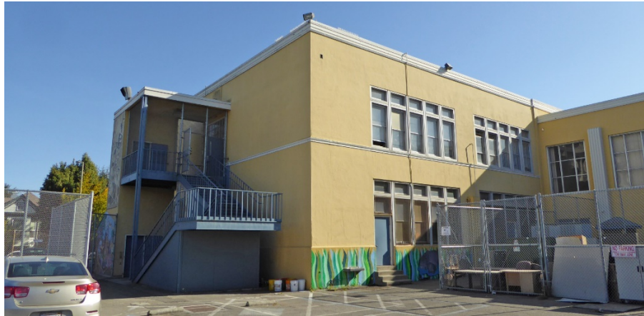
Figure 20: View of northeast wing at rear façade, looking southeast.
