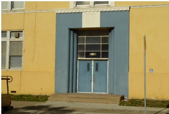
Figure 17: East entrance at south façade, looking north.
