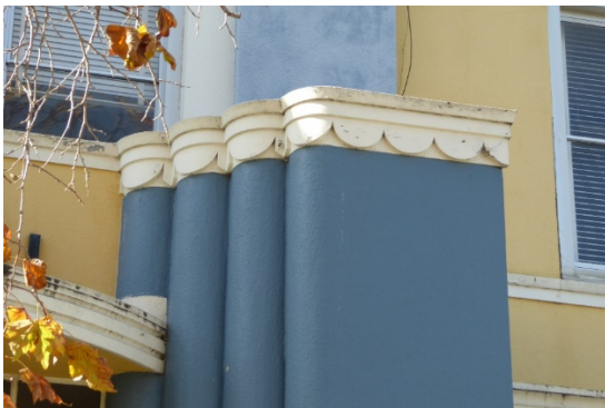
Figure 5: Scalloped capital details, visible at columns flanking main entrance, looking west.
