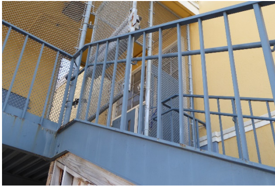
Figure 23: Detail of staircase and second story landing, looking southeast.
