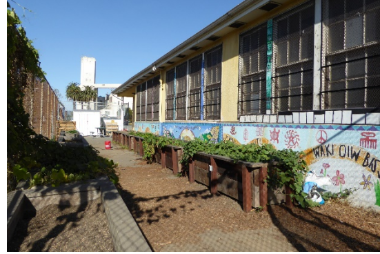
Figure 35: West façade, looking north.
