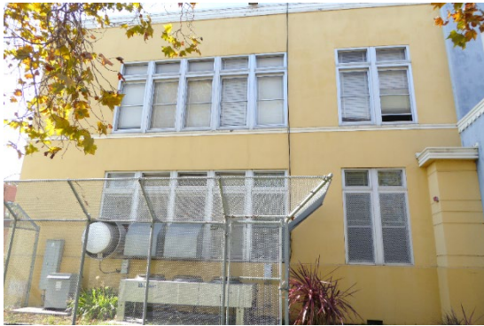
Figure 8: Two southernmost bays at the primary façade, looking west.
