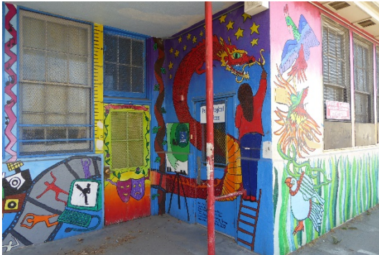
Figure 30: Recessed entrance at southeast corner, looking northwest.
