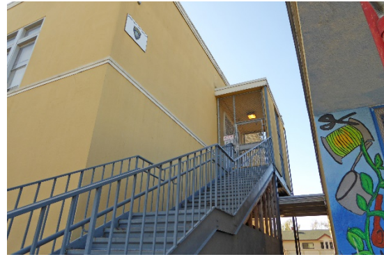
Figure 28: Linear staircase at rear façade of the west wing, looking west.
