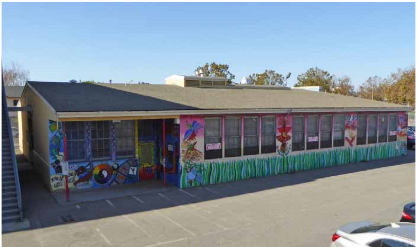
Former Cafeteria Building
