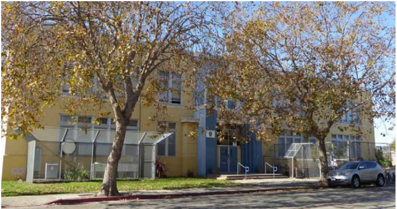
Existing Cole Middle School Building
