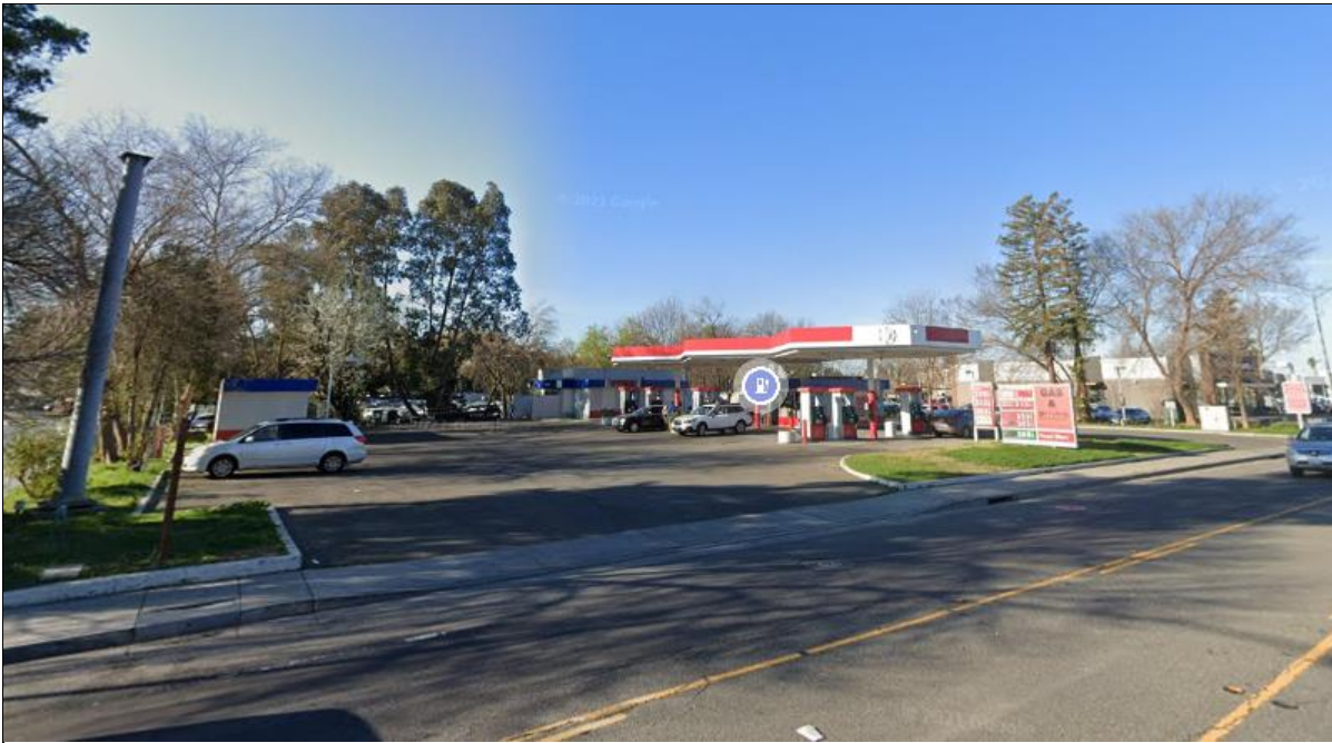
Figure 1. Google Street View of Subject Site – 4480 Chiles Road
