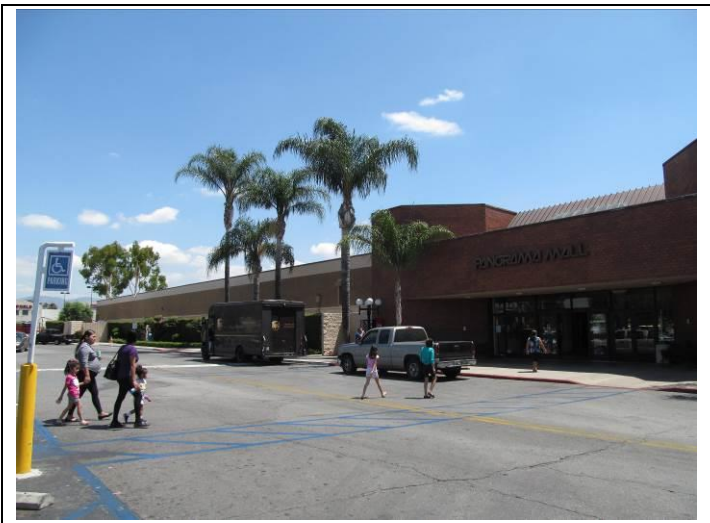
3. West elevation and single-story construction
