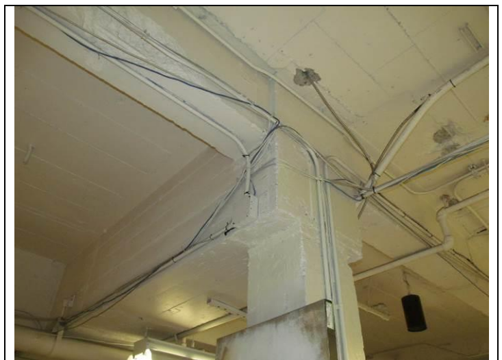
18. Concrete framing in basement of Curacao
