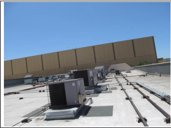
19. Roof deck over Building Sections A & B and gas lines
