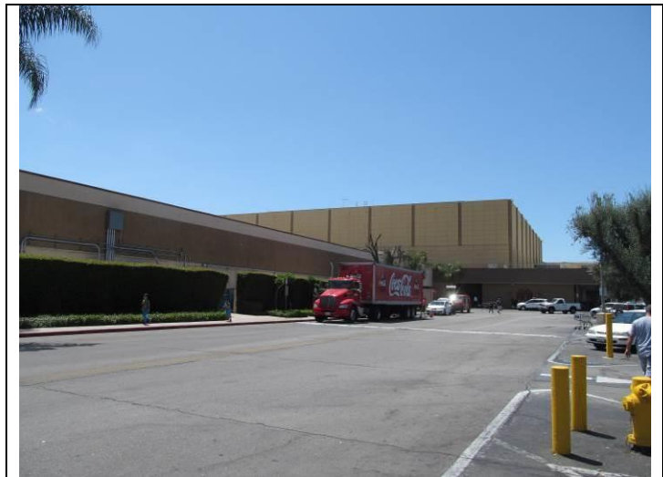
4. West elevation and brick veneer
