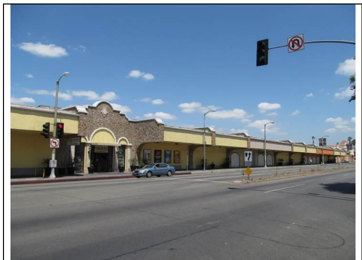
6. East elevation and east entrance
