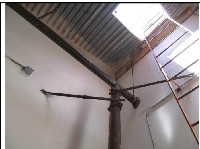
29. Four-inch fire suppression lines braced
