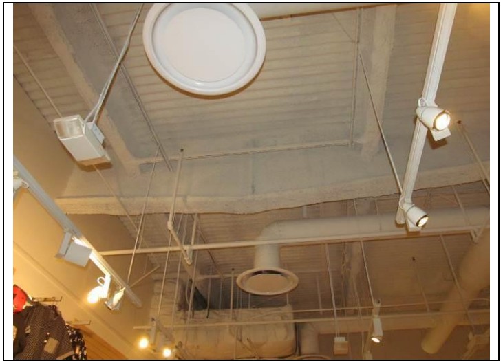
32. Tapered steel girder beams in Buildings A & B 1979
