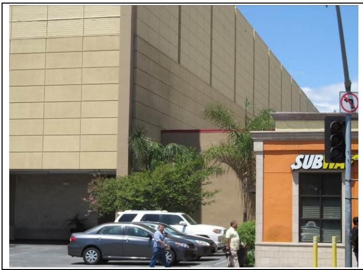
7. Abutment to the Walmart building
