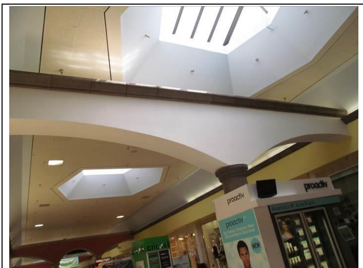
11. Linkage between the older building section and the newer wings A & B
