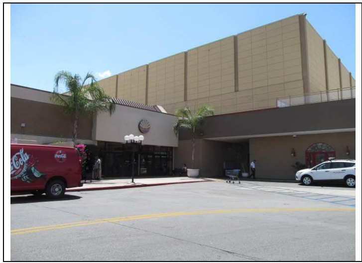
2. West elevation abutment to two-story building (Walmart)
