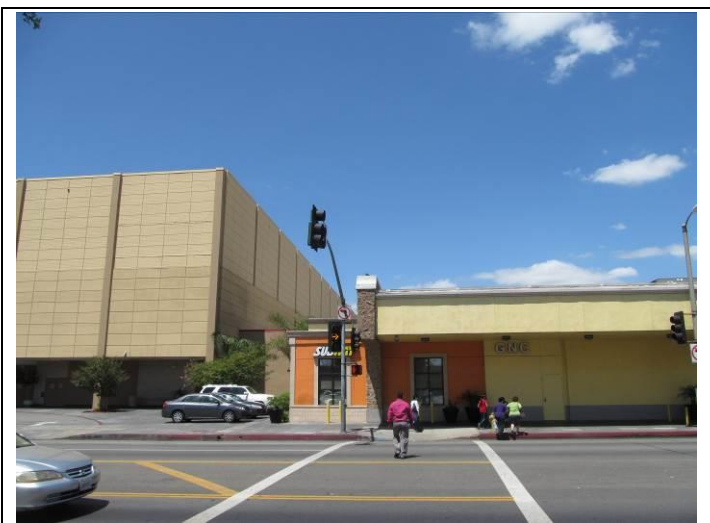
5. East elevation at abutment to Walmart
