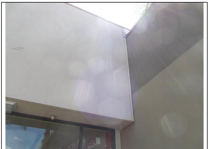
36. Building separation at transition to Walmart
