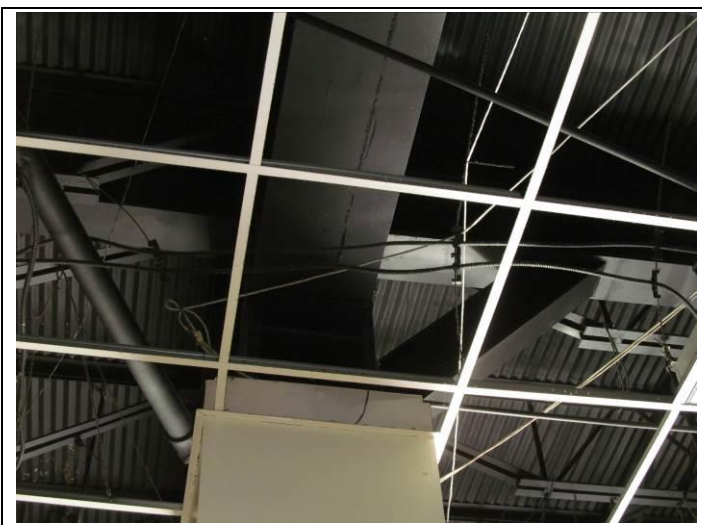
17. Steel framing and knee bracing in Curacao
