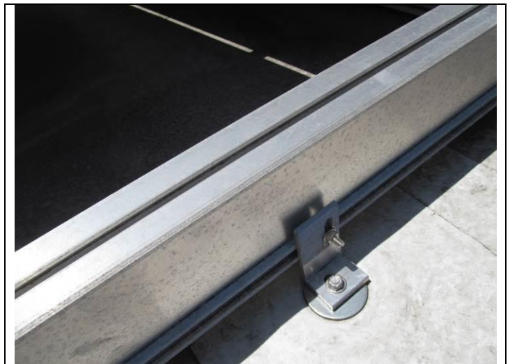
24. Solar system anchorage against sliding
