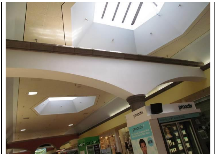
34. Linkage framing between old and newer construction
