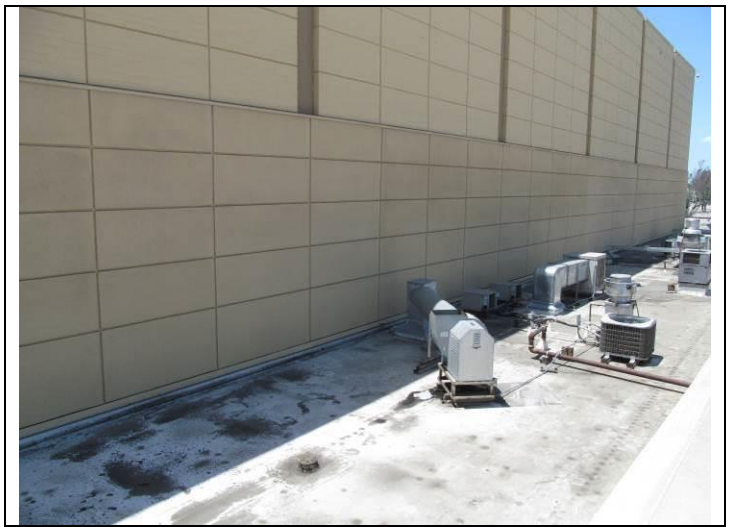
8. Roof view of abutment to the Walmart building
