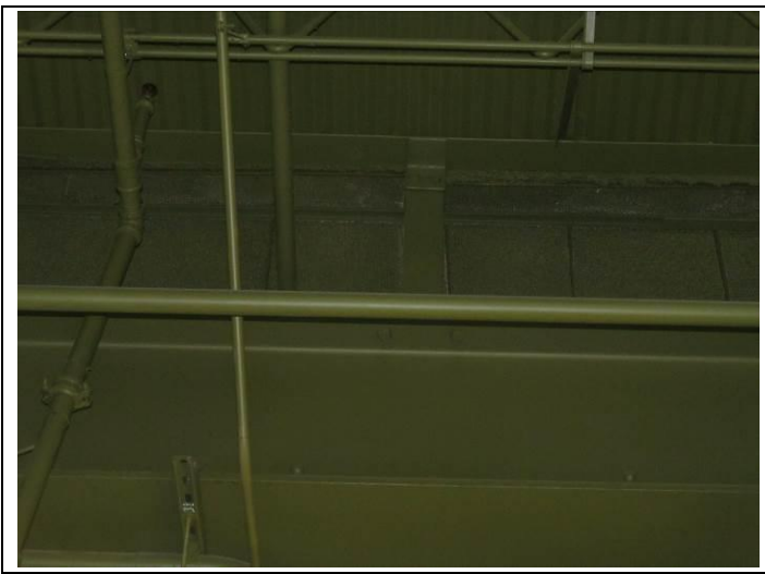
13. Steel roof framing and corrugated steel deck roof
