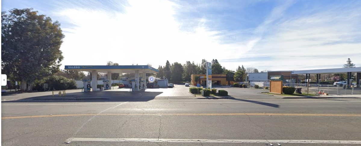
Figure 1: Google Street View of Subject Site – 4748 & 4810 Chiles Road
